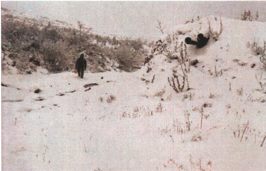
Photograph 14: Steel decant pipes in constructed ponds along the water course
