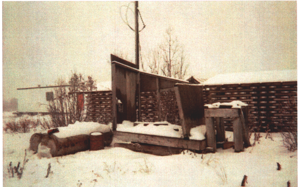
Photograph 23: Collapsed shed presumably used for refueling or storage of related products.
