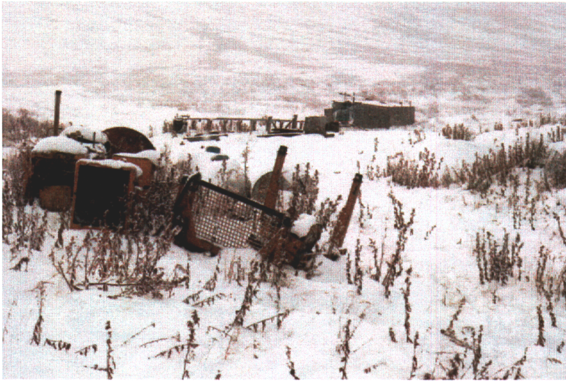
Photograph 4: View toward maintenance shed with disassembled dozers in foreground and conveyor in the middle ground
