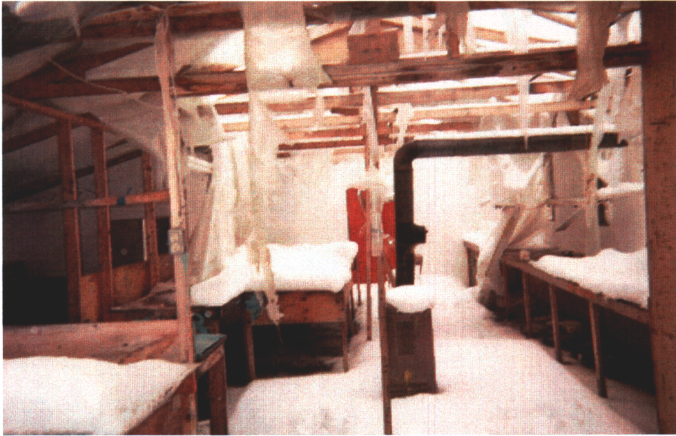
Photograph 26: Interior of one of the core examination sheds
