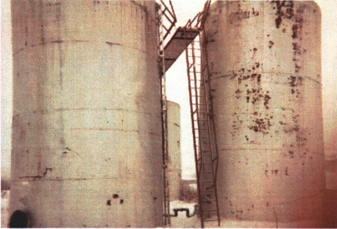
Photograph 9: Three vertical storage tanks on tank farm showing open manhole cover.
