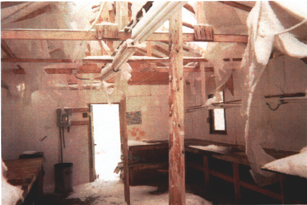
Photograph 25: Interior of one of the core examination sheds
