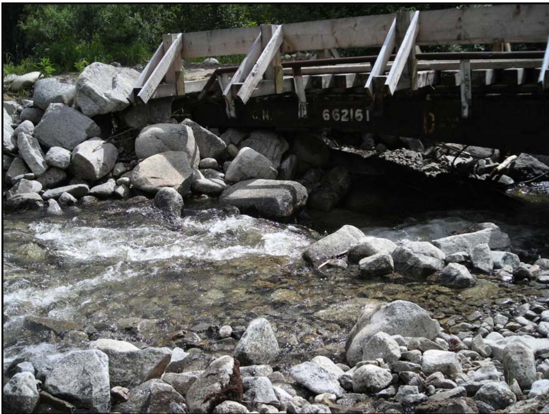
CMC-M2- downstream towards bridge 2007
