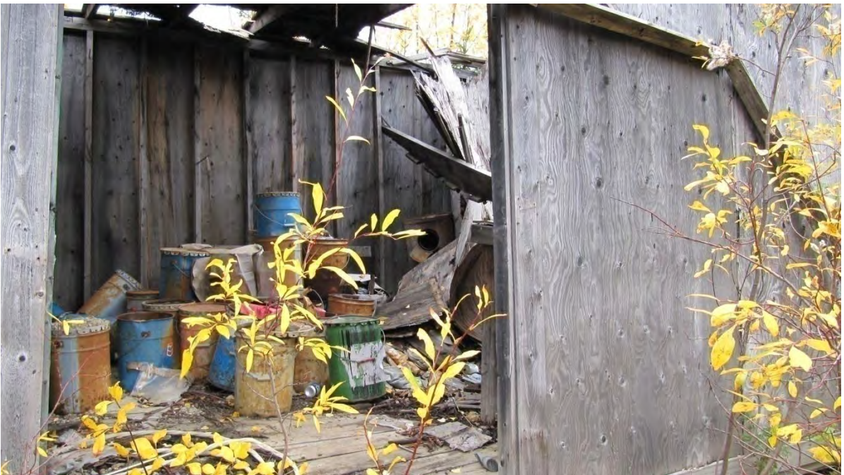
Plate 16: Site 1, interior view west of structure [6]
