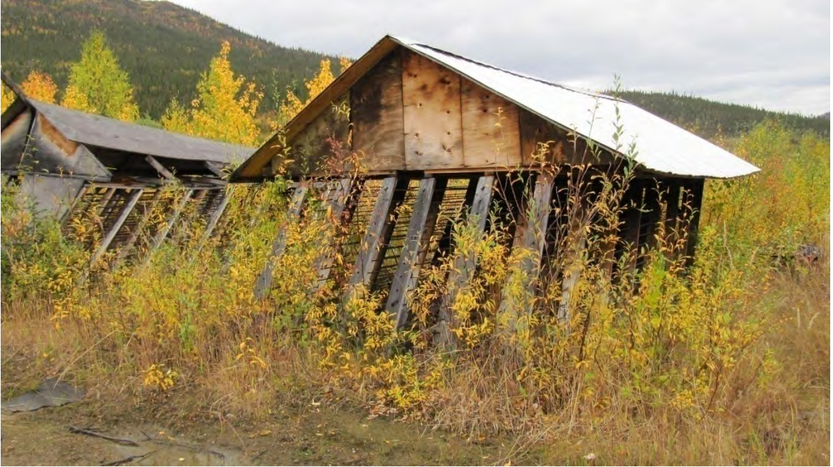
Plate 17: Site 1, view west at core structures [3]
