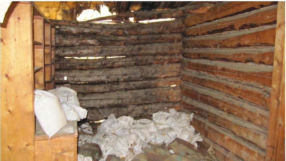
Plate 30: Site 2 structure, interior view of north wall
