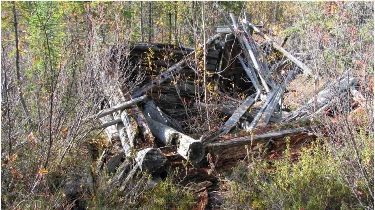
Plate 35: Site 3 structure, view west
