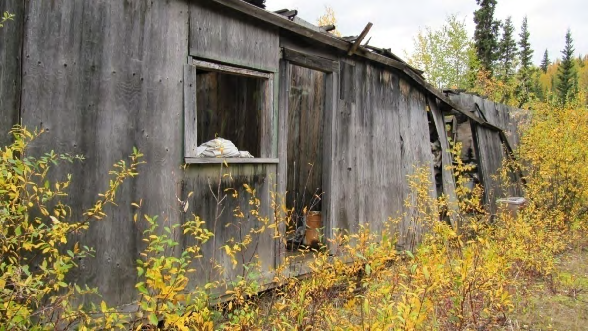
Plate 15: Site 1, plank/board/plywood structure [6], view northwest
