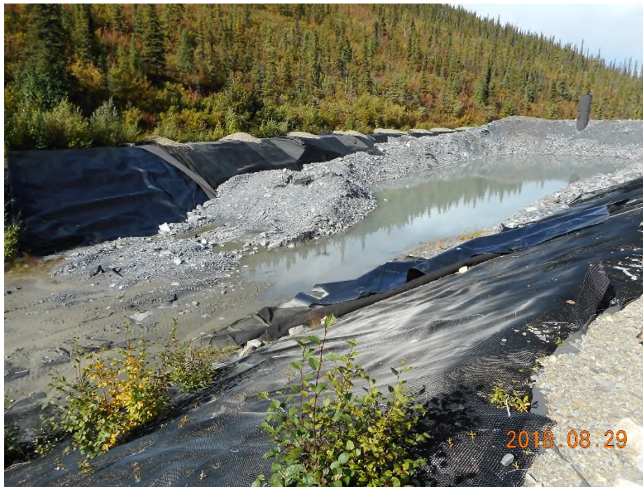
Photo 1: View of PAG waste storage cell south of Bellekeno portal
