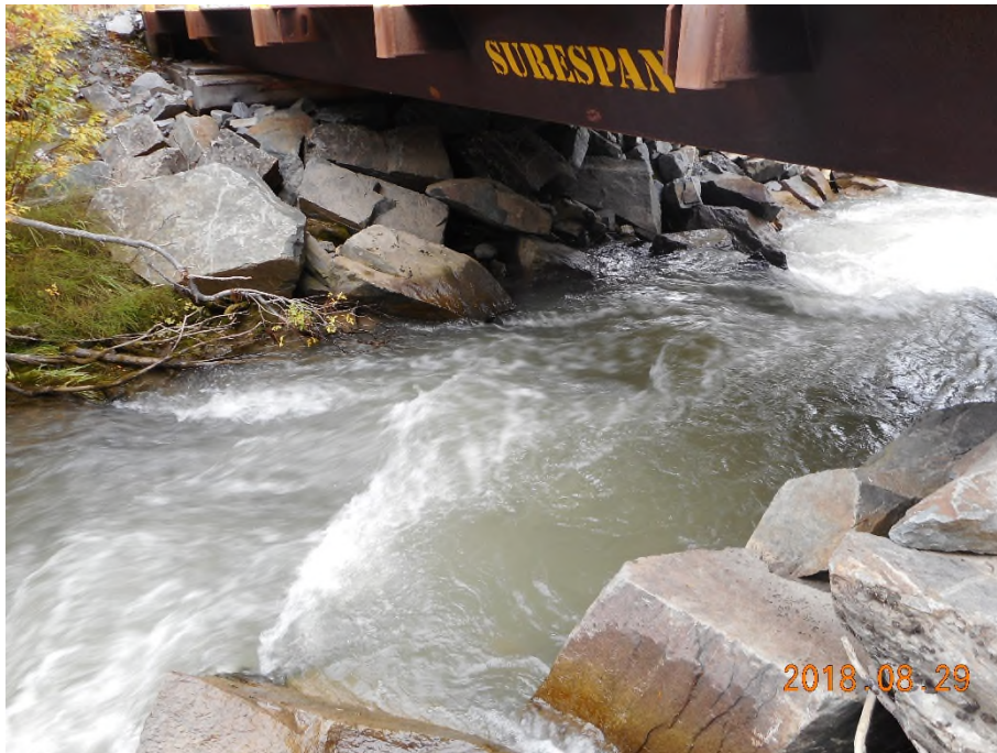
Photo 4: Well armoured bridge abutments at Lightning Creek crossing by the Onek road.
