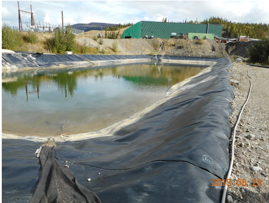
Photo 6: One of the mill water ponds at the Mill Site – stable berms and sideslopes.
