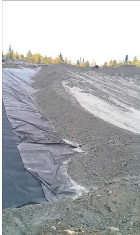
Photo 11: Compacted DSTF Lift
