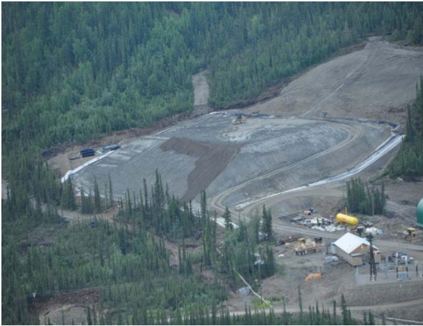
Photo 12: Aerial view of progressive reclamation of DSTF – 2012
