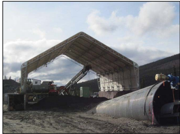
Photo 3: Fine Ore Storage
