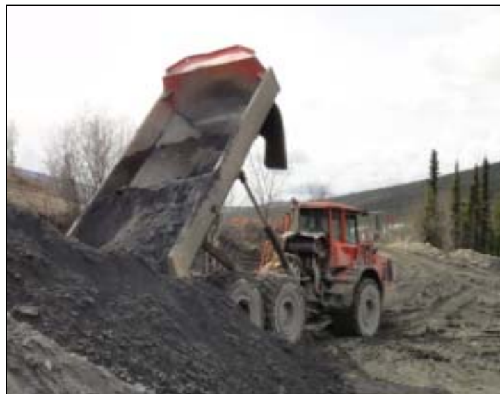
Photo 1: ROM Ore Crushing, Ore Storage and Reclaim
