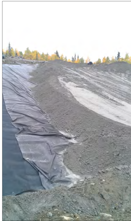
Photo 11: Compacted DSTF Lift
