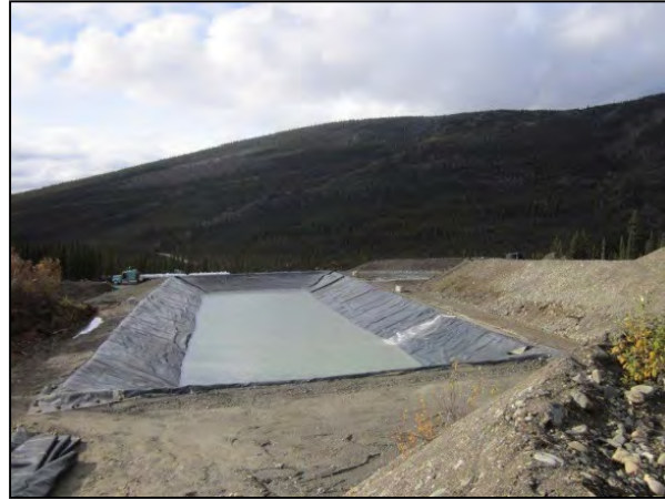
Photo 15: Process Water Pond
