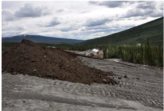
Photo 13: Progressive reclamation of DSTF
