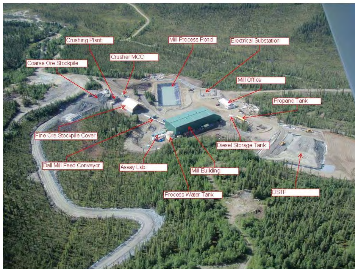
Figure 4-1 Mill Infrastructure Overview
