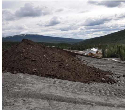
Photo 13: Progressive reclamation of DSTF - 2012
