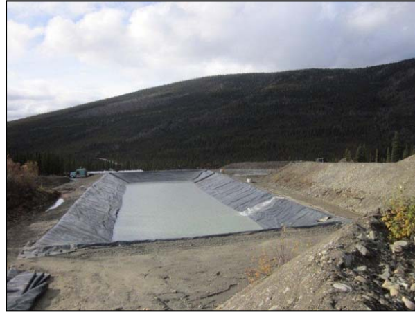
Photo 16: Process Water Pond
