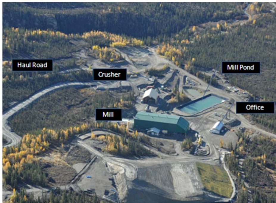
Figure 4-1 Mill Infrastructure Overview
