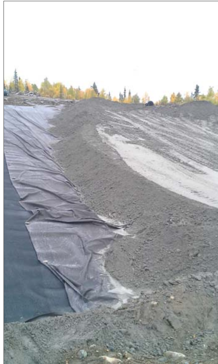
Photo 11: Compacted DSTF Lift
