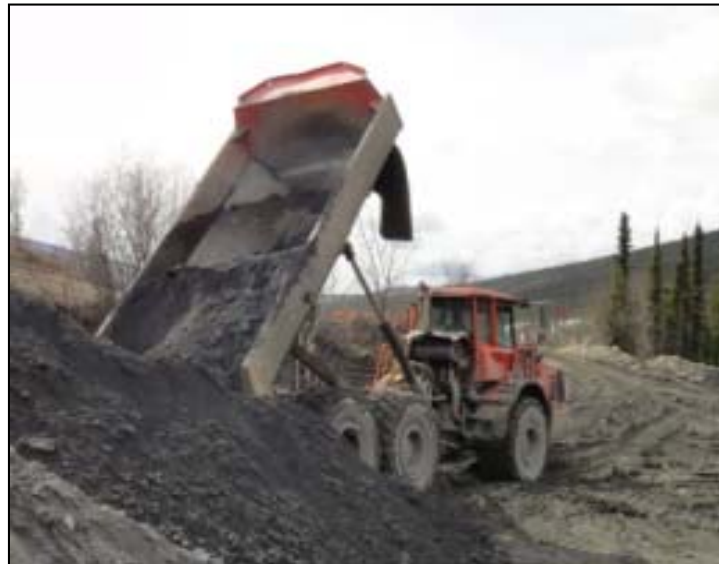
Photo 1: ROM Ore Crushing, Ore Storage and Reclaim
