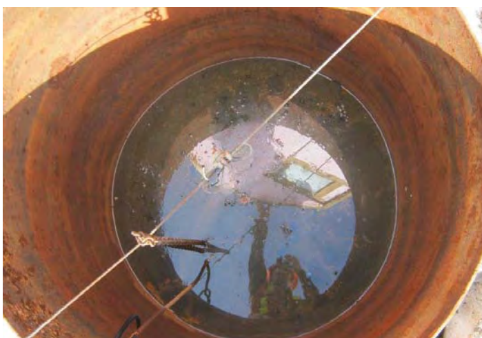
Figure 3 - Bioreactor Influent Sump
