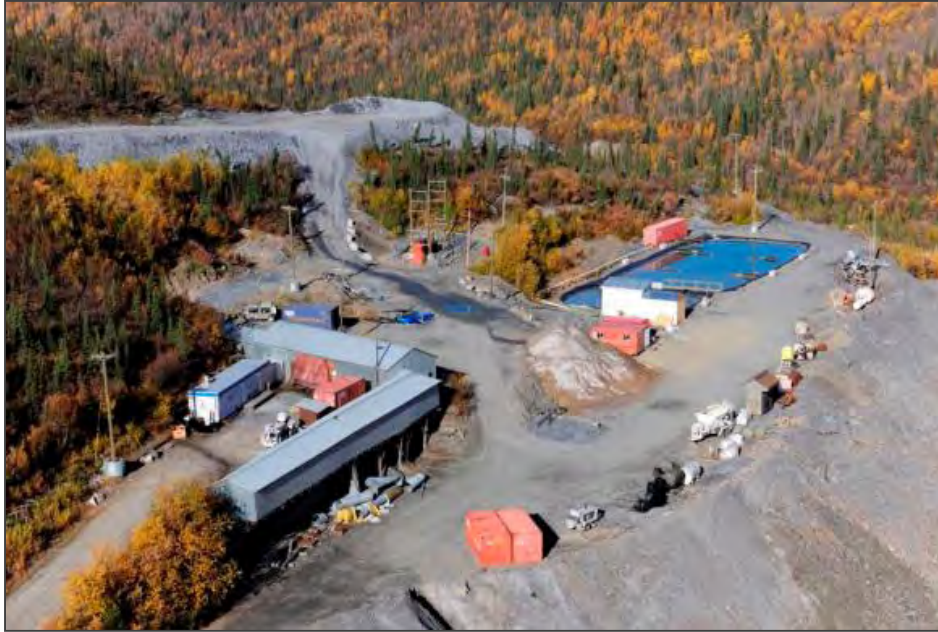
Plate 7-1: Bellekeno 625 Area Overview
