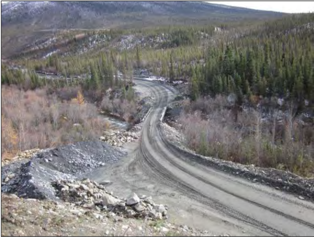
Plate 7-4: Lightning Creek Bridge and Typical Haul Road Section
