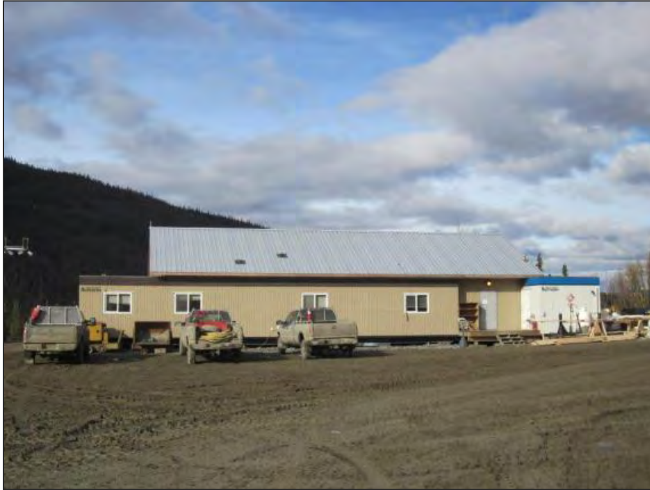
Plate 7-7: Mill Office and Dry
