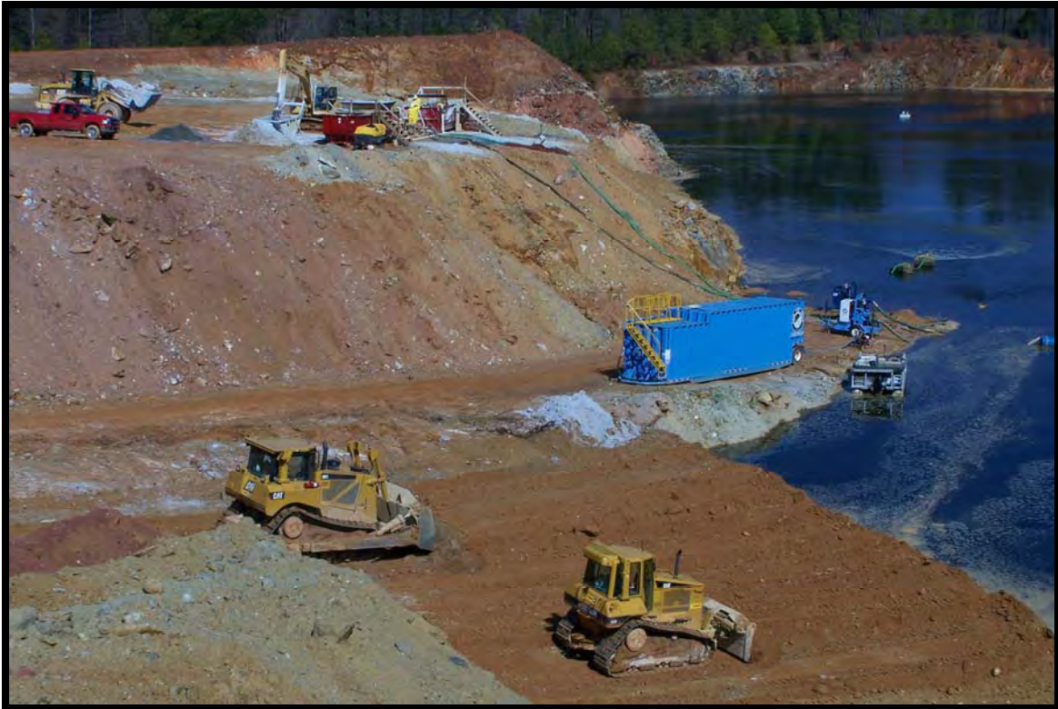
Figure 5 Simultaneous waste rock grading and carbon loading/carbide lime in situ neutralization at the pit lake
