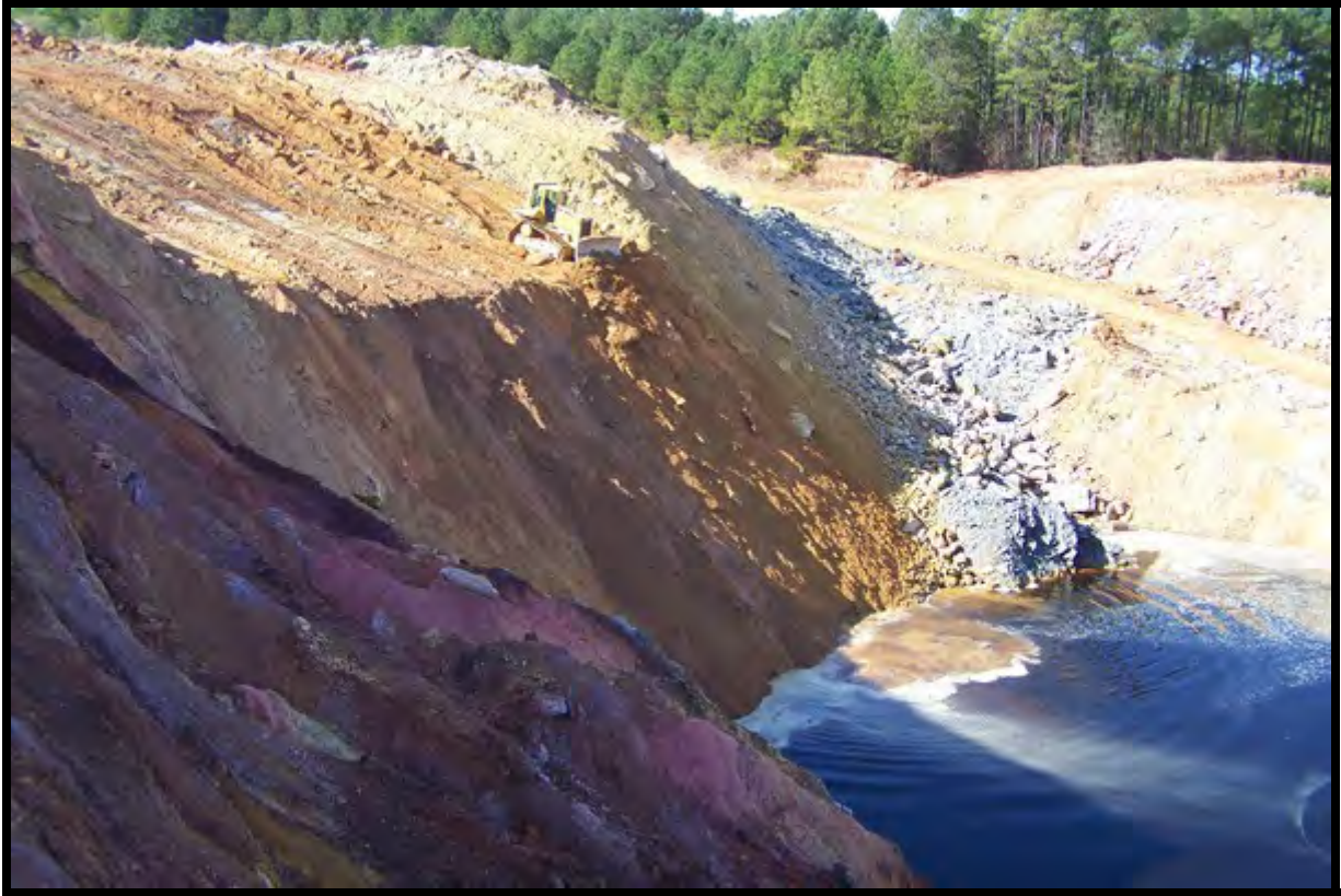
Figure 4 Grading of the South Waste Rock Pile
