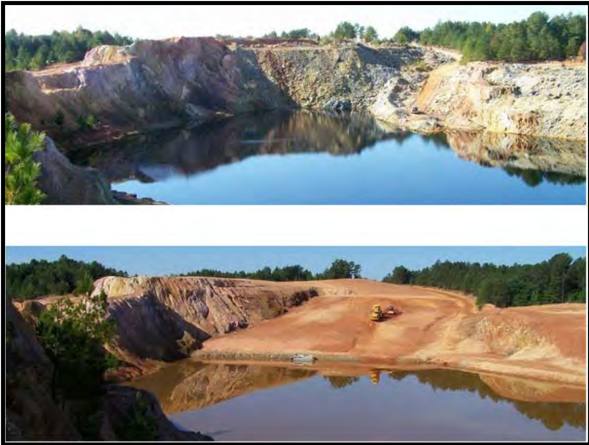
Figure 3 Pit Lake before and after implementation of the chosen remedy (pre toe and topsoil construction)
