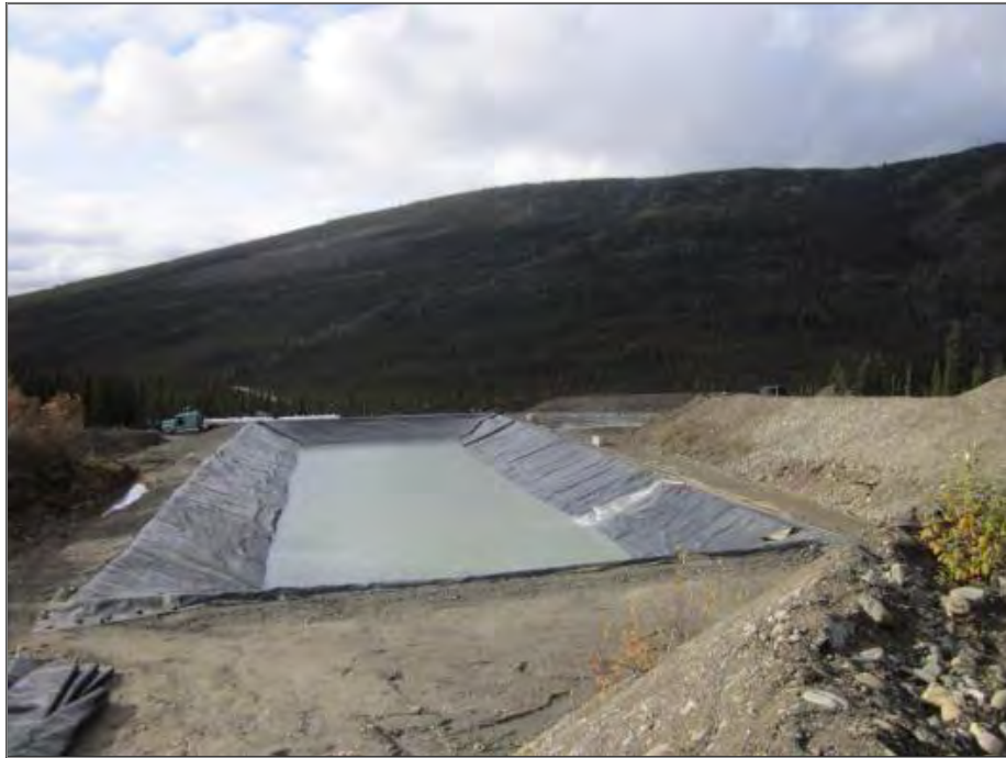
Plate 7-9: Mill Process Pond
