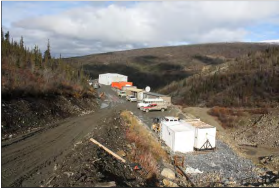
Plate 7-2: Bellekeno East Surface Facilities
