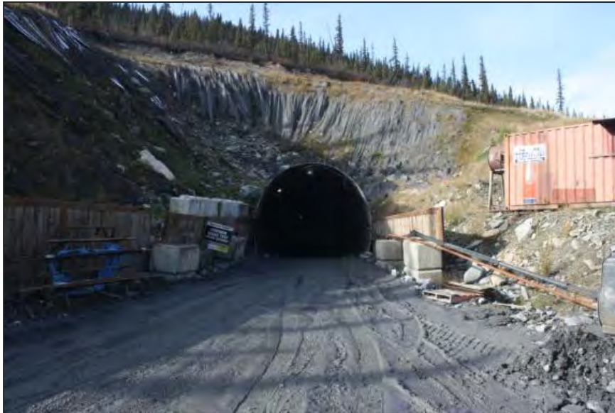
Plate 7-3: Bellekeno East Portal
