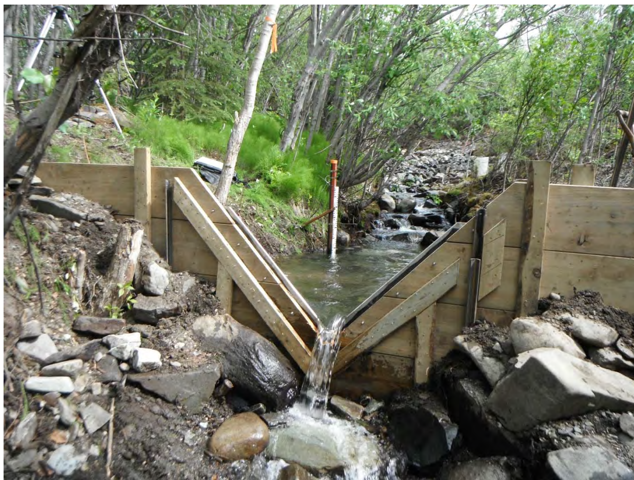
Figure 3 – Weir at KV-21, June 2015
