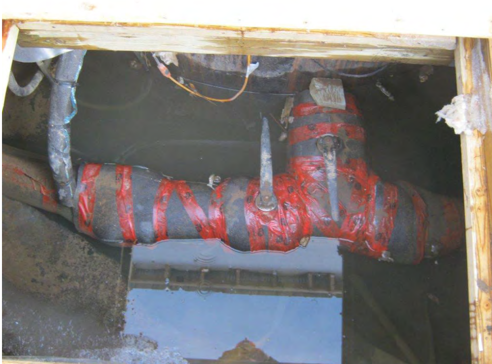
Figure 8 - Bioreactor Discharge Valves
