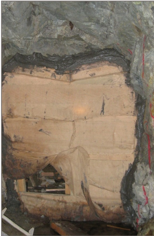
Photo 9: Temporary Bulkhead - Perimeter of lagging packed with burlap and grouted
