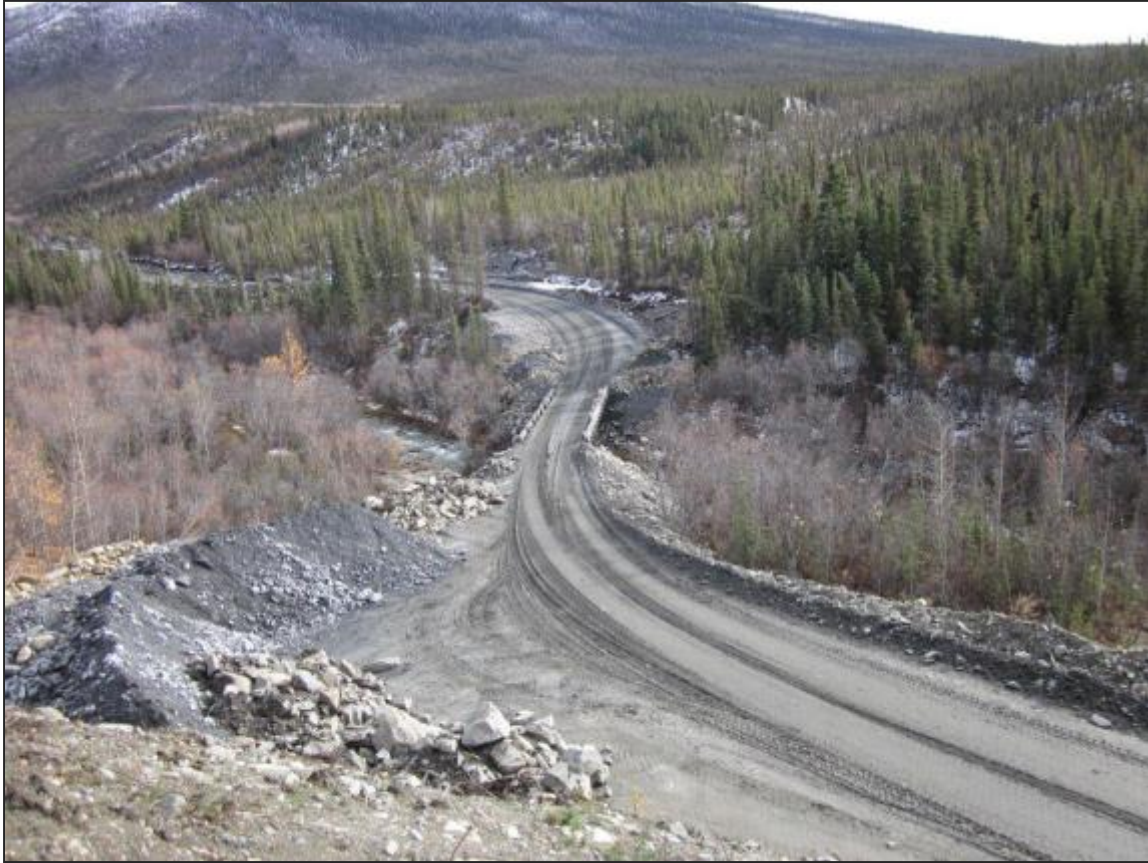
Plate 6-5: Lightning Creek Bridge and Typical Haul Road Section
