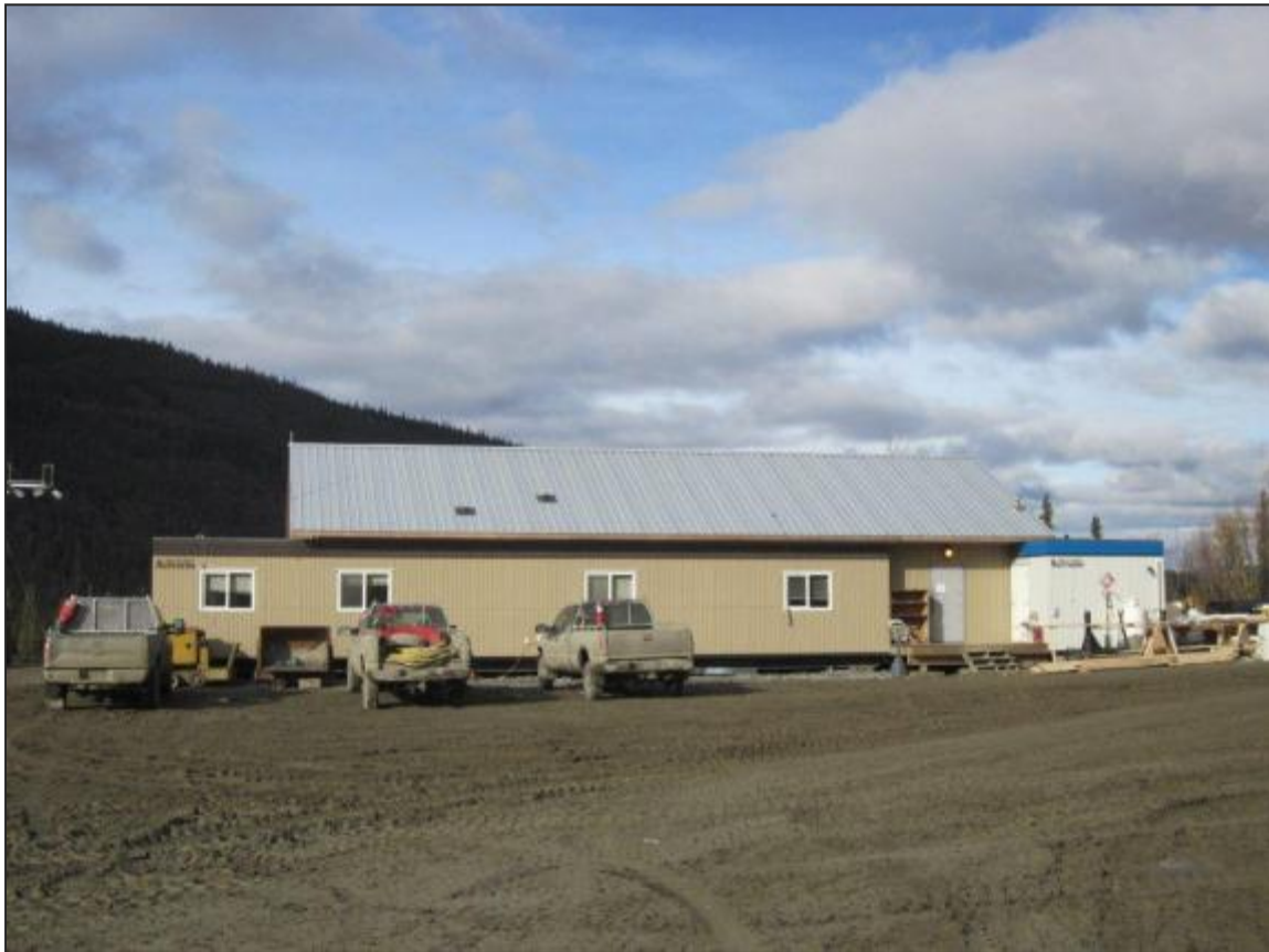
Plate 6-8: Mill Office and Dry
