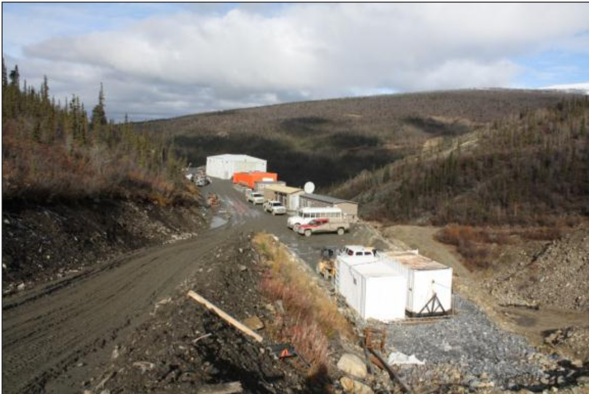
Plate 6-2: Bellekeno East Surface Facilities
