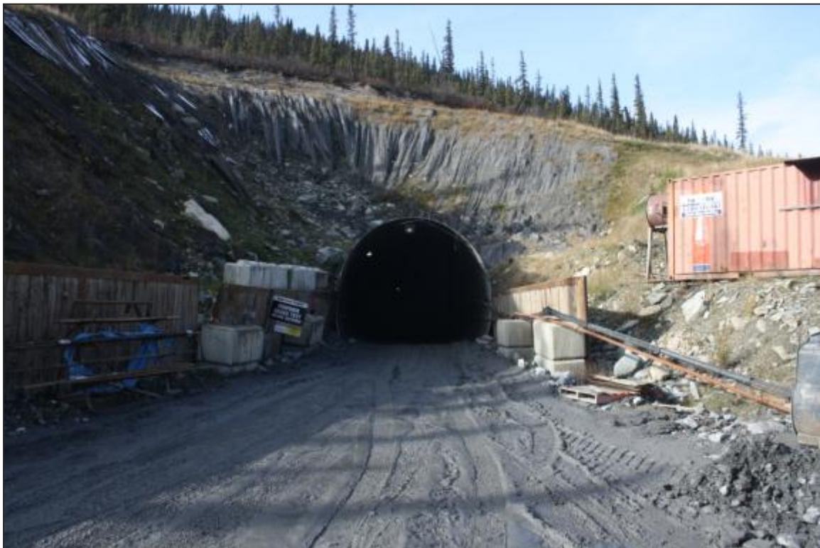
Plate 6-1: Bellekeno East Portal
