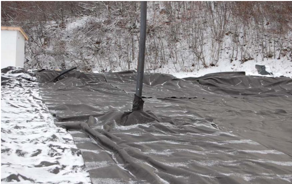
FIGURE 6 – BIOREACTOR STANDPIPE
