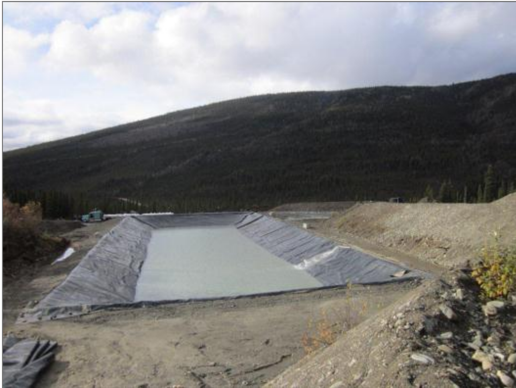
Plate 6-10: Mill Process Pond
