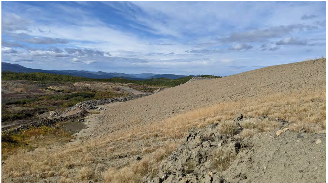
Photo 4-4: Regraded MWD slope looking towards the Reclamation Overburden Dump.
