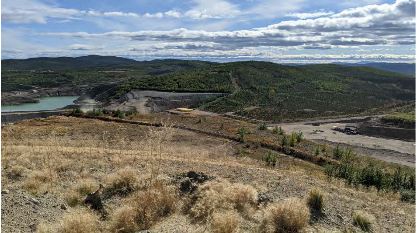
Photo 4-5: View from the top of the MWD Expansion looking down to the top of the original MWD.
