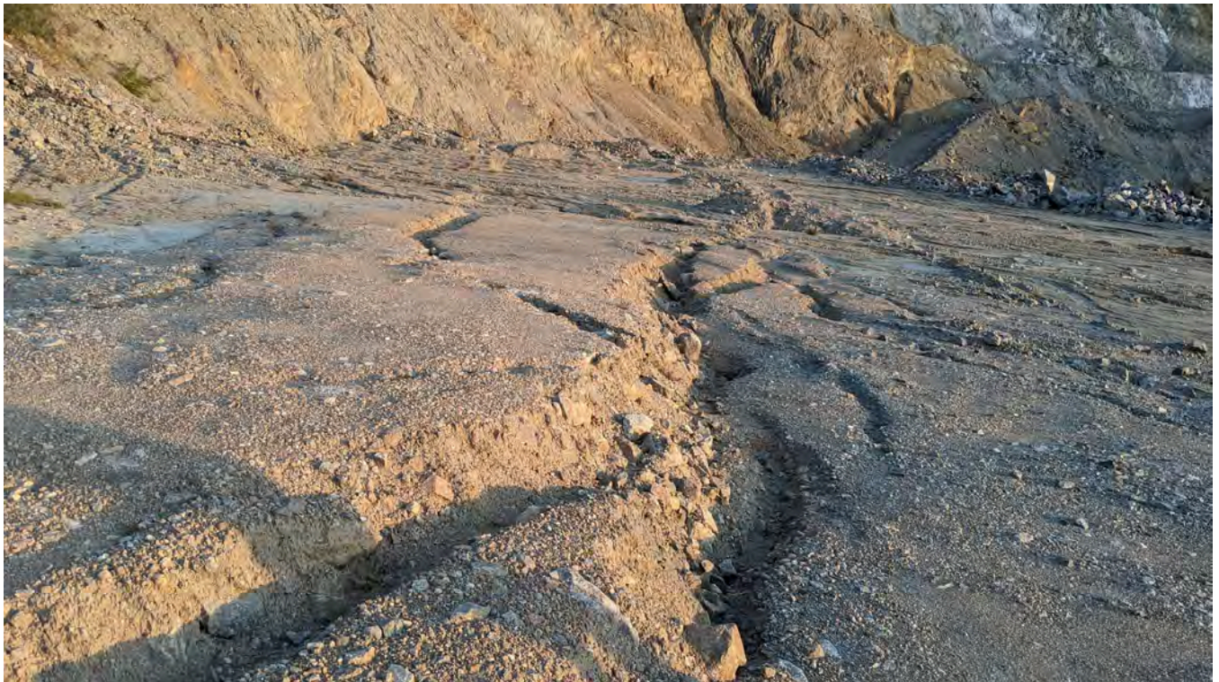
Photo 14-8: Historical cracking of the In-Pit Dump above the SAT Dump. The cracks are filling-in and near-by survey hubs indicate no current movement.
