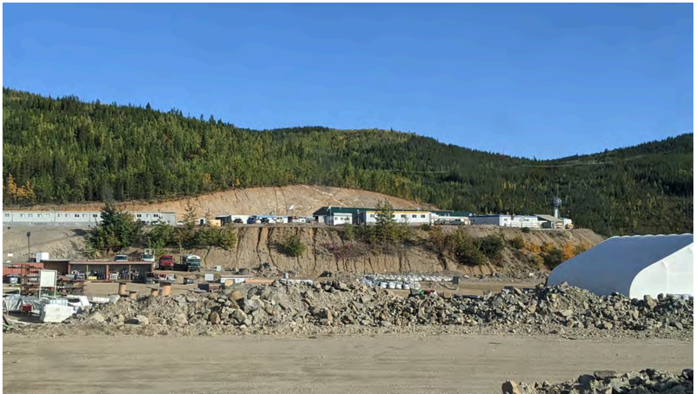
Photo 10-4: Historical erosion gullies below the camp pad. The condition of the gullies is unchanged from previous inspections and the camp pad is graded to prevent runoff entering the top of the gullies.
