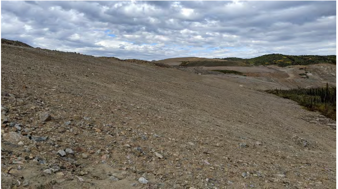
Photo 6-6: Reggraded SWD slope below the longitudinal cracks.
