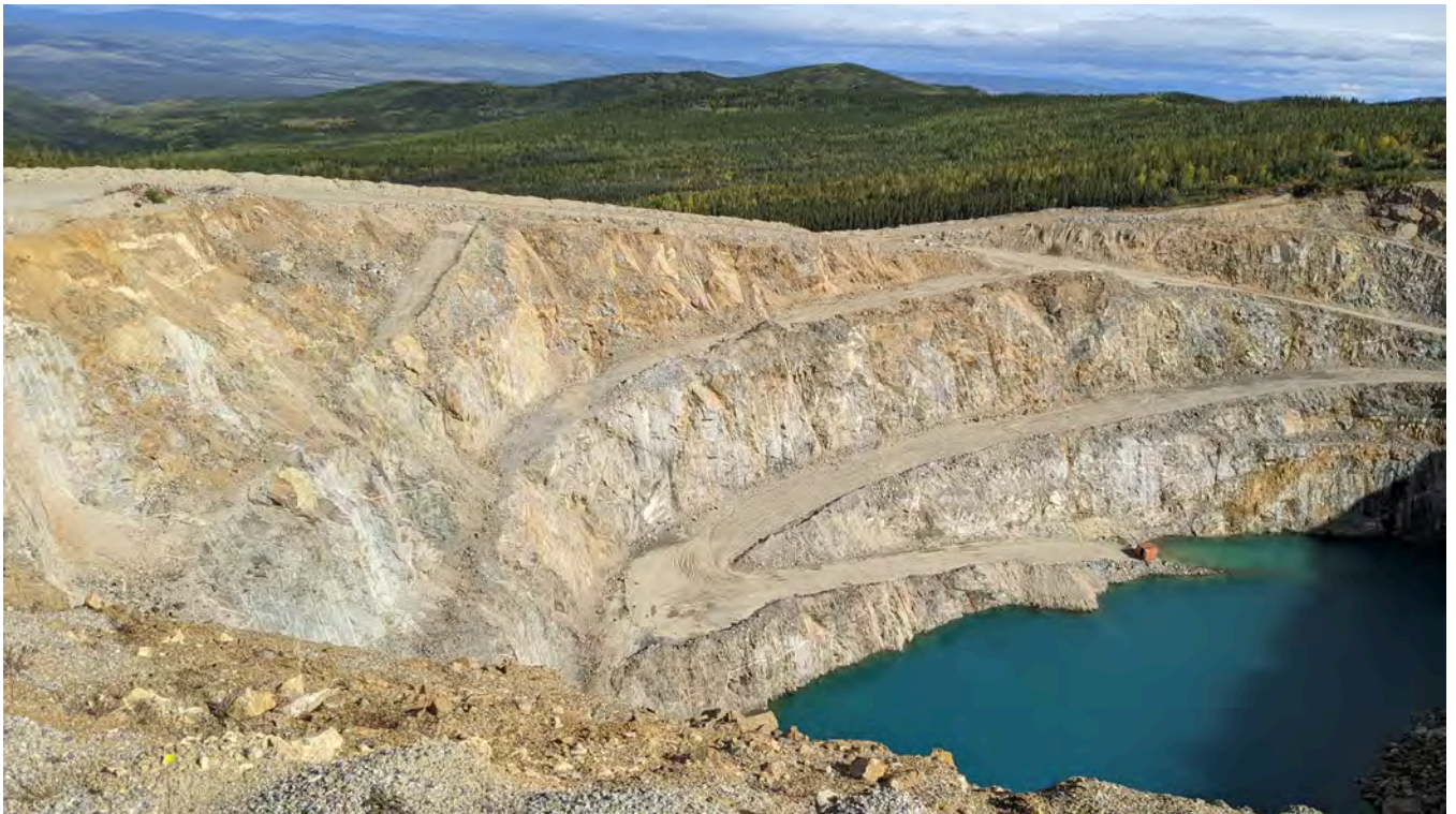
Photo 17-2: North pit wall.
