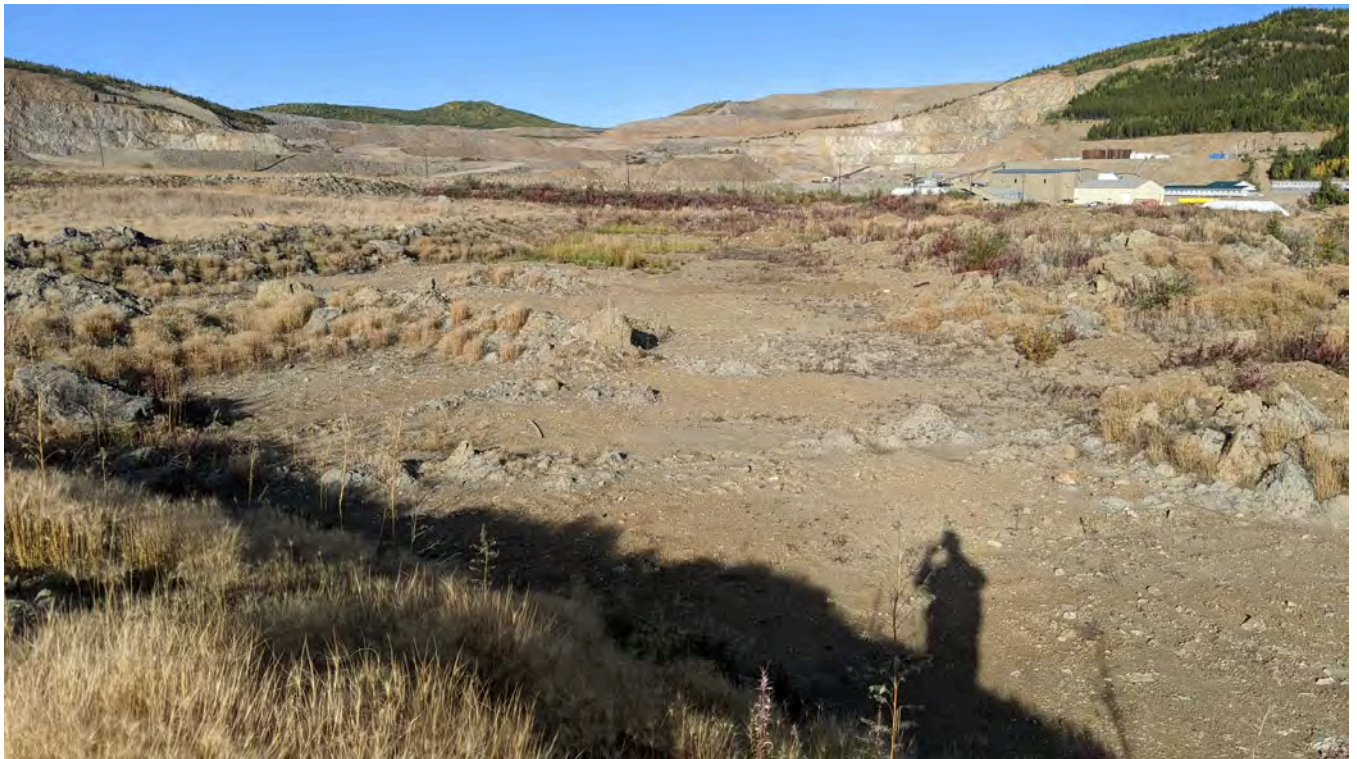
Photo 1-4: Covered DSTSF surface in an area with no vegetation.
