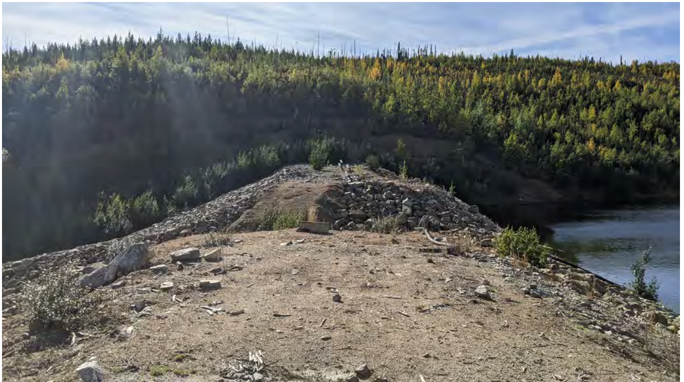
Photo 12-2: WSP Crest taken from the north abutment looking south.
