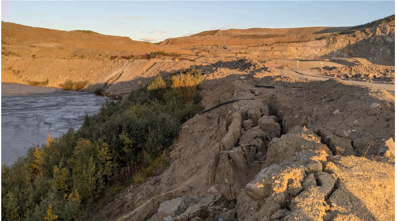
Photo 15-5: Cracking along the pit rim.
