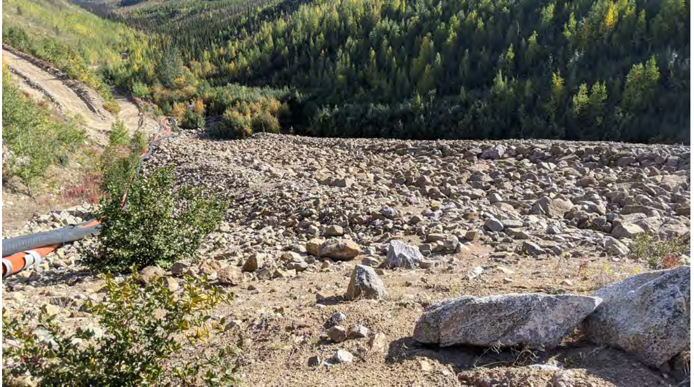
Photo 12-3: WSP spillway looking downstream.
