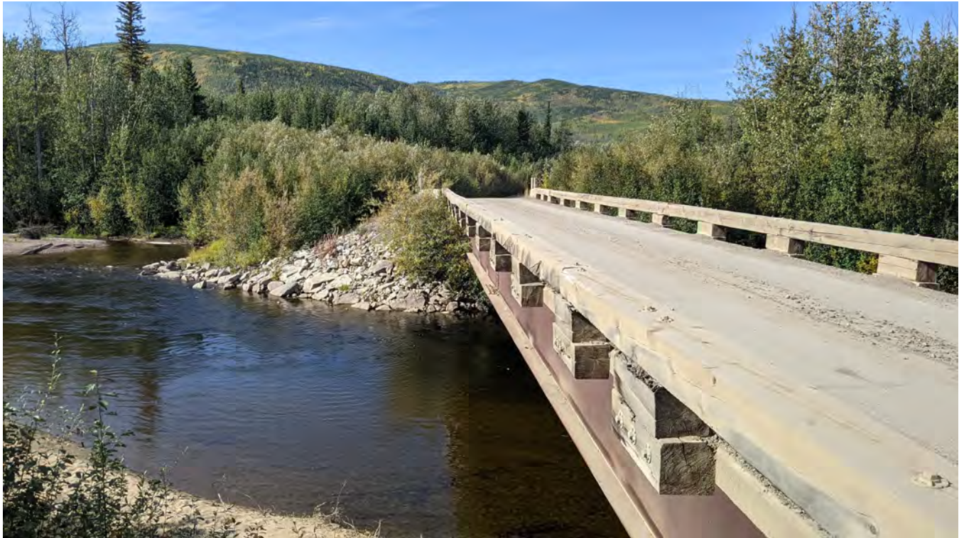
Photo 13-1: Western bridge abutment.
