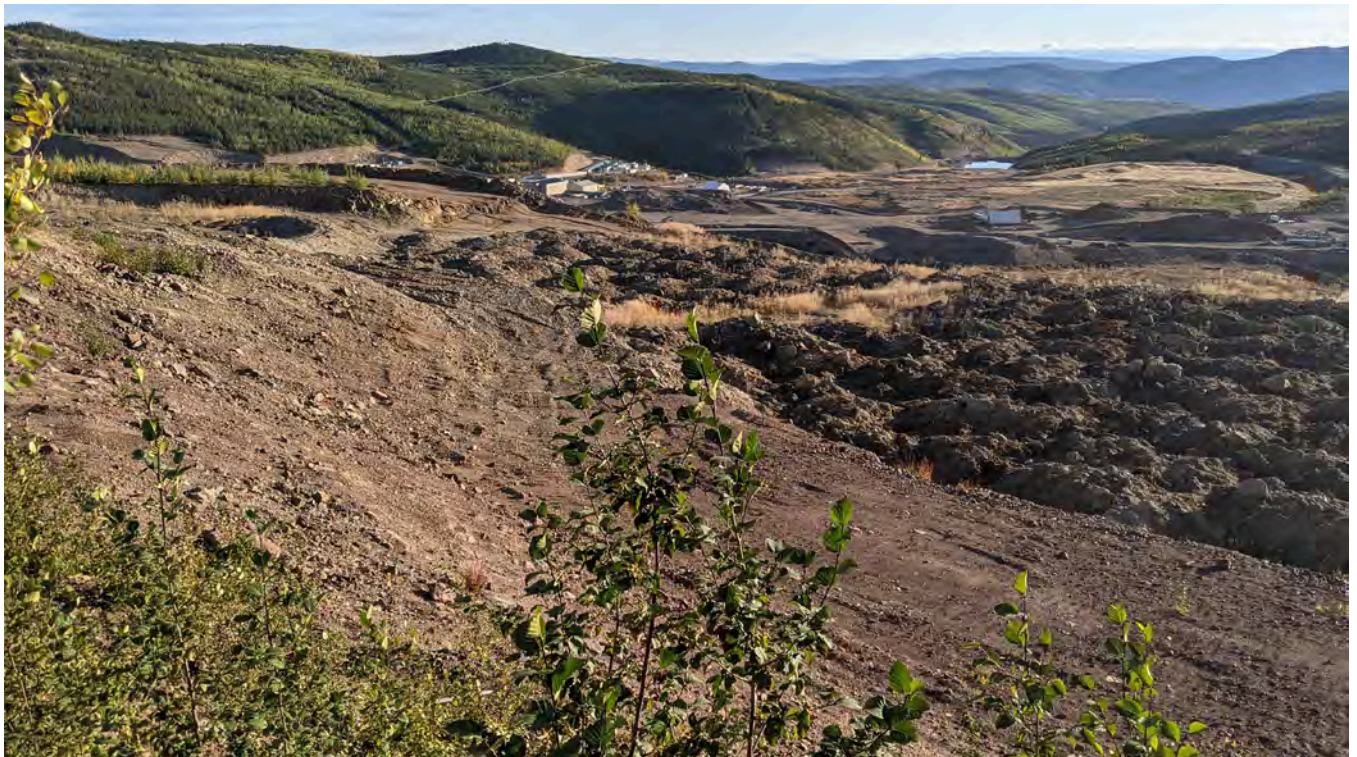
Photo 16-2: North end of the Area 118 Pit
