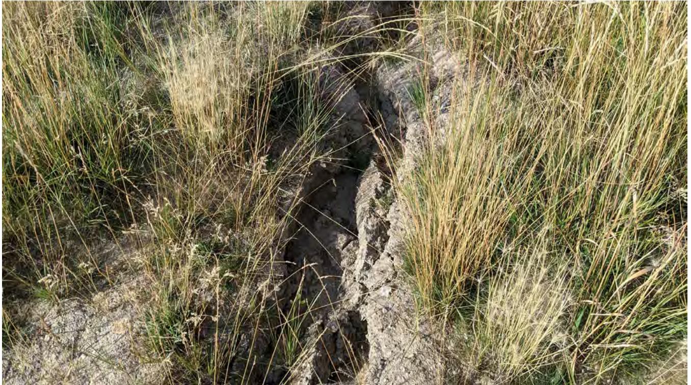
Photo 1-7: Erosion gully on regraded cover slope at the northeast corner of the DSTSF.
