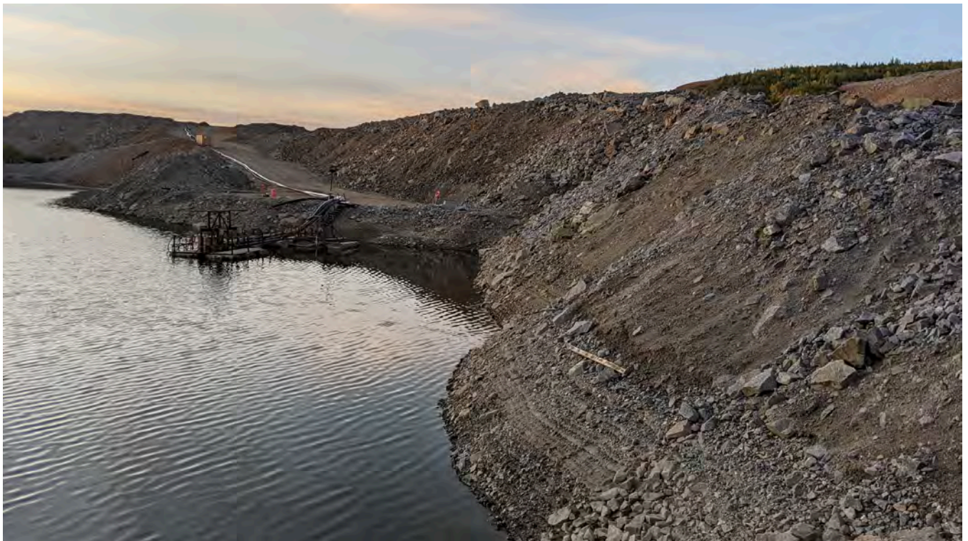
Photo 14-6: Main Pit Reclaim Barge and In-Pit Dumps.
