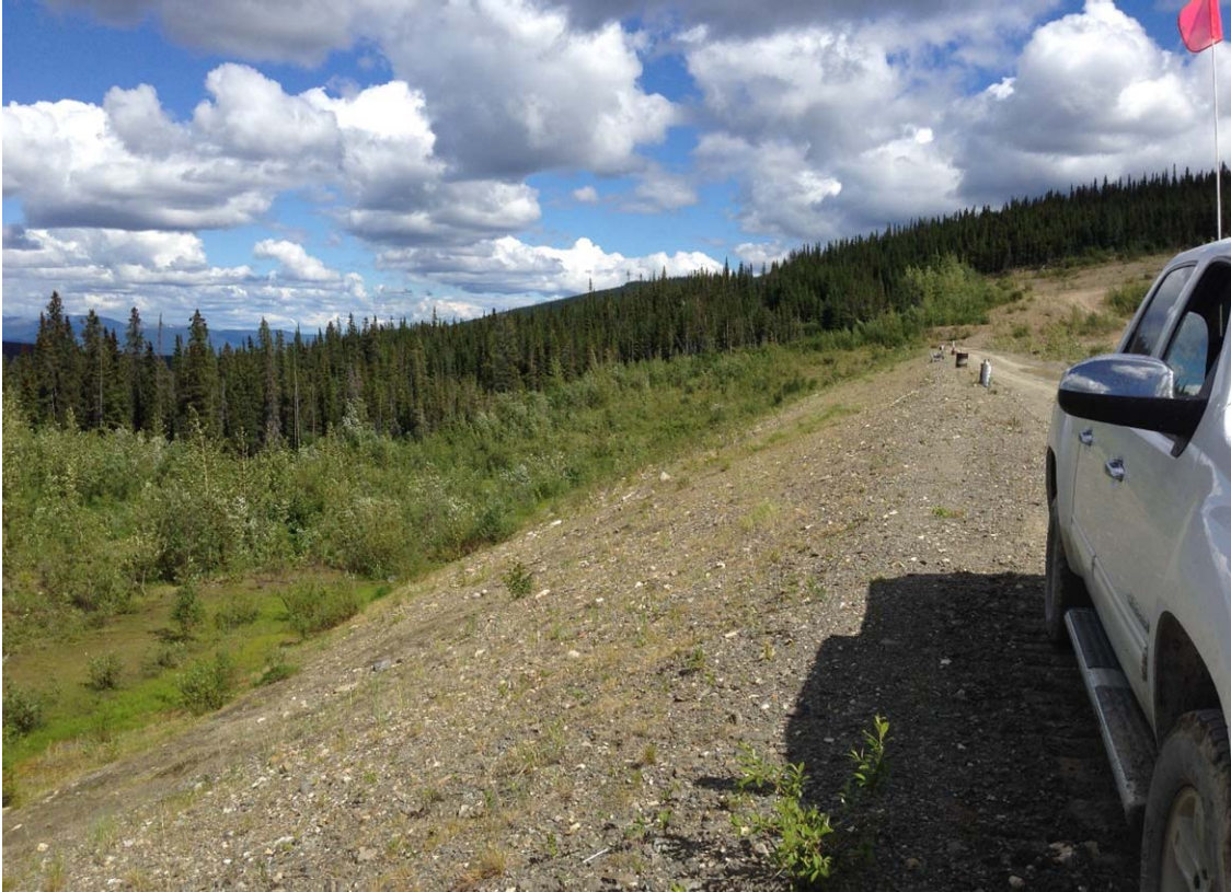
Photo 5: View of the downstream face of the North Dam.
