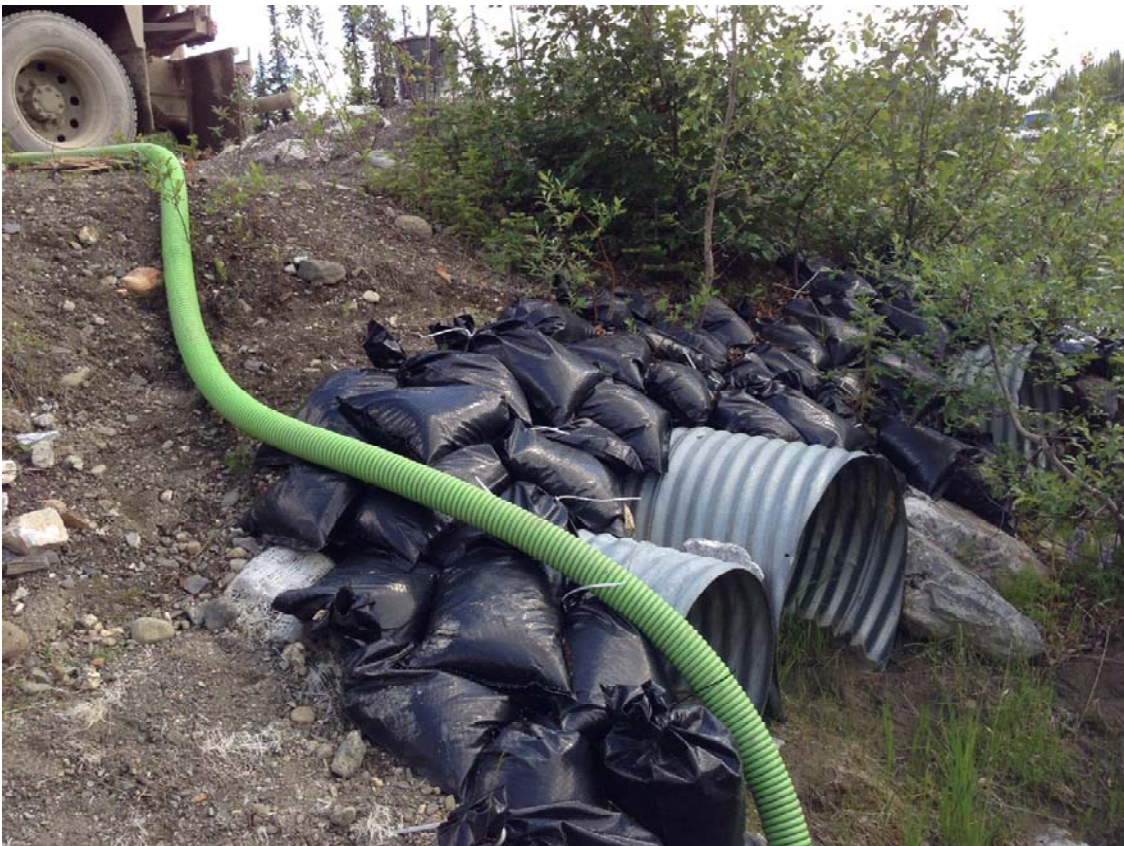
Photo 6: Inlet Culverts at the North Creek Dyke.
