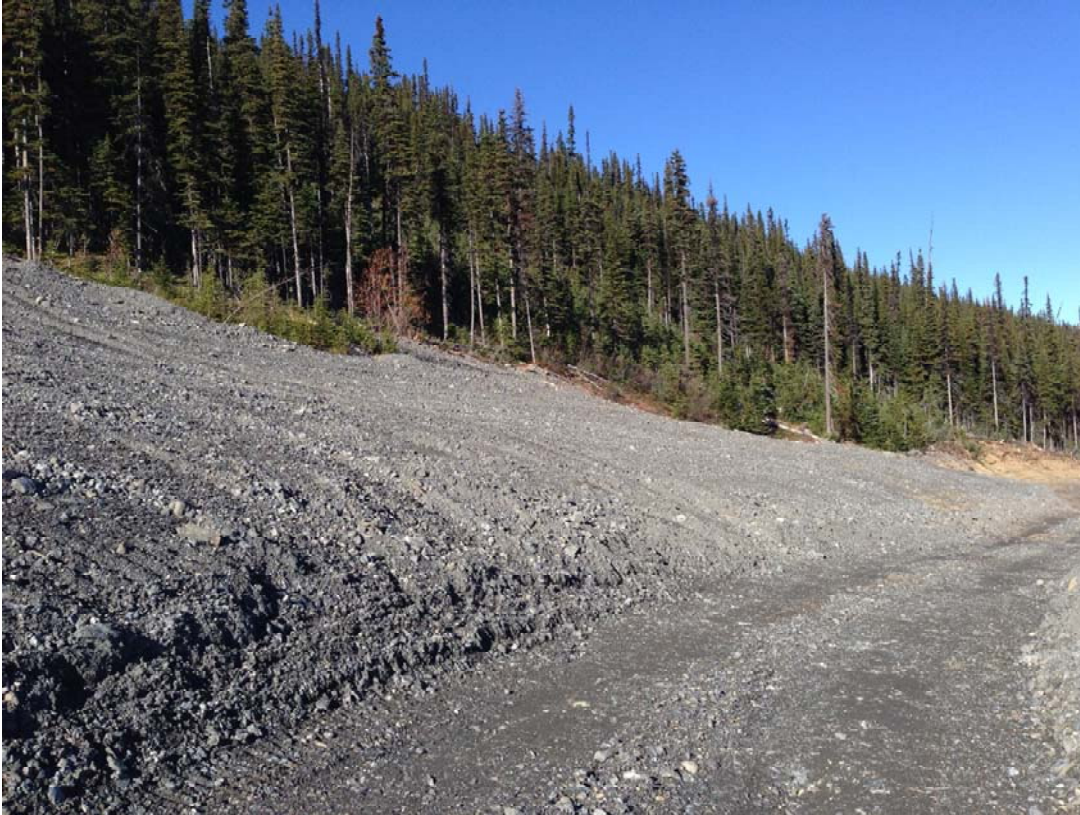
Photo 13: Contoured backfill placed up against the 1200 Portal.
