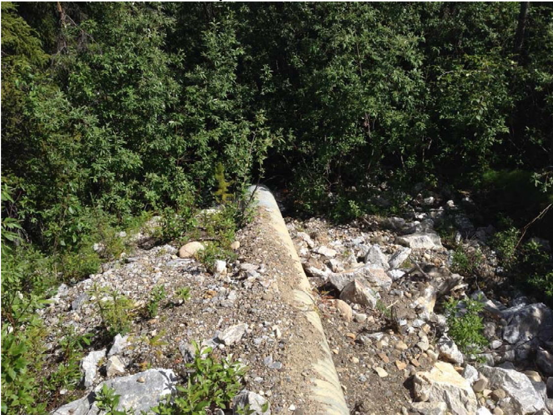
Photo 8: Main outlet culvert at the North Creek Dyke.
