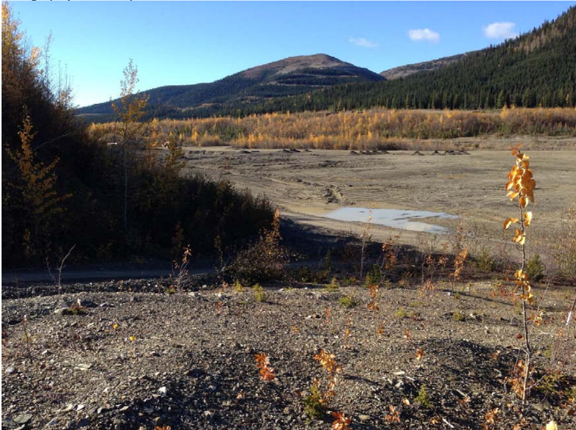
Photo 4: View over the capped tailings surface at the north end of the TMF (Sept 23, 2014).
