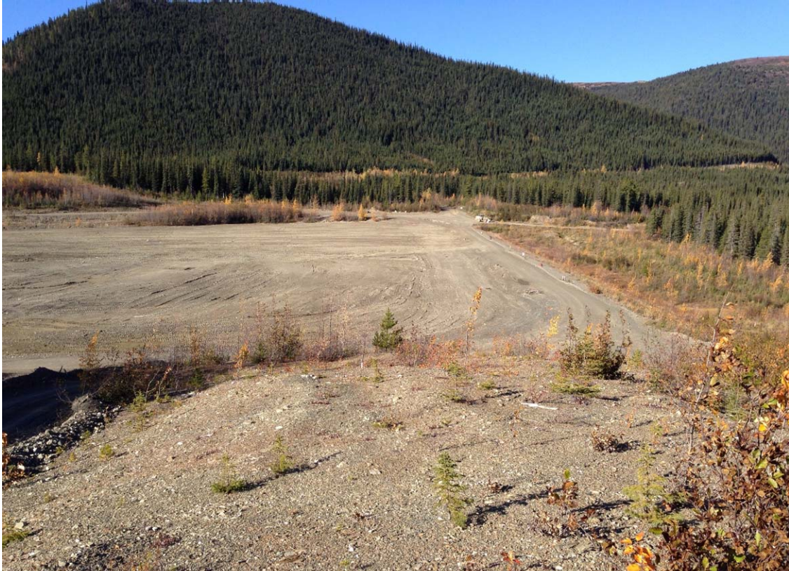
Photo 3: View looking east along the North Dam and the soil cover that was placed over the tailings (Sept 23, 2014).
