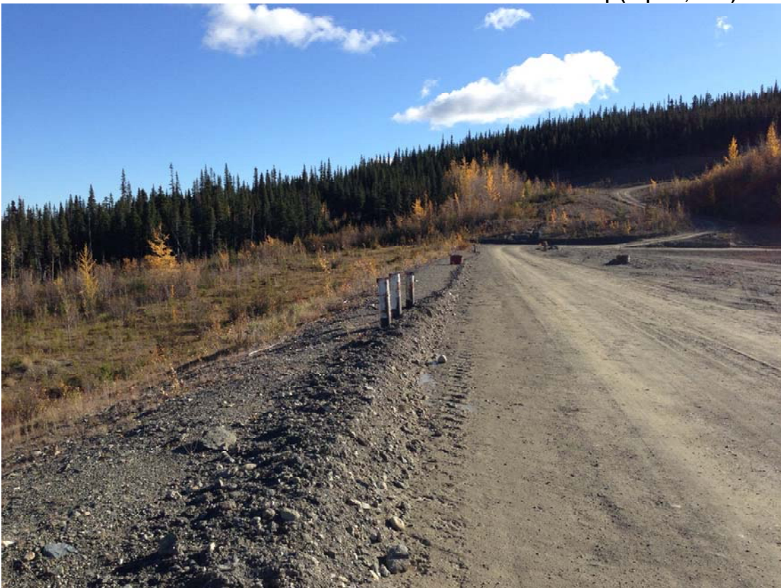
Photo 2: View east along the North Dam Crest.
