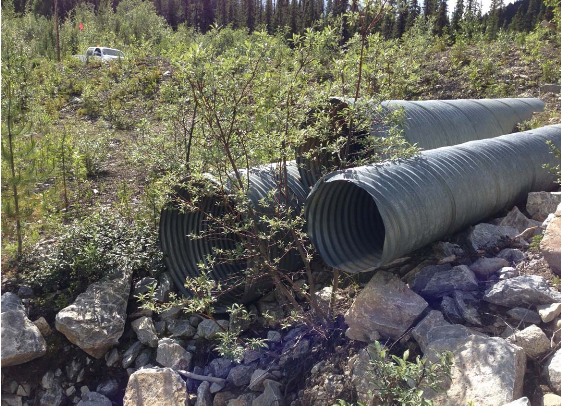
Photo 7: Outlet culverts at the North Dyke.
