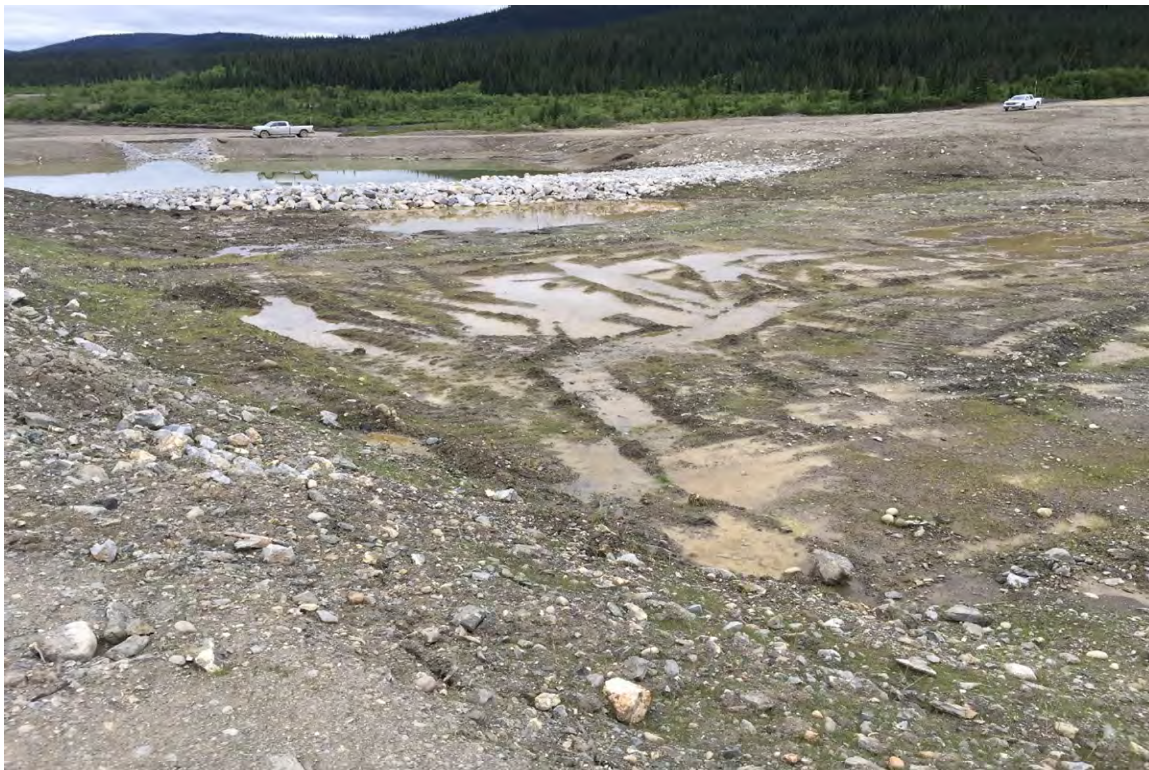
Photo 13: View of the rockfill cofferdam above the SRS
