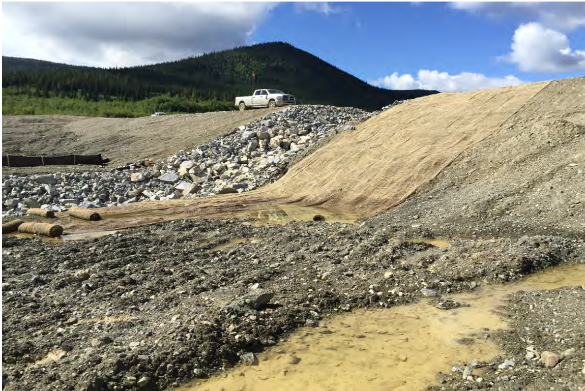
Photo 14: View looking west of the spillway through the SRS.
