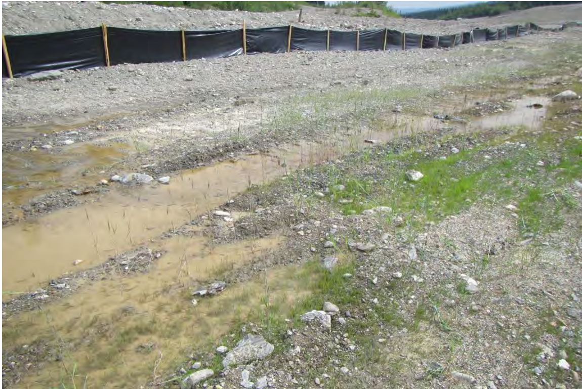
Photo 16: Silt fences for TSS management
