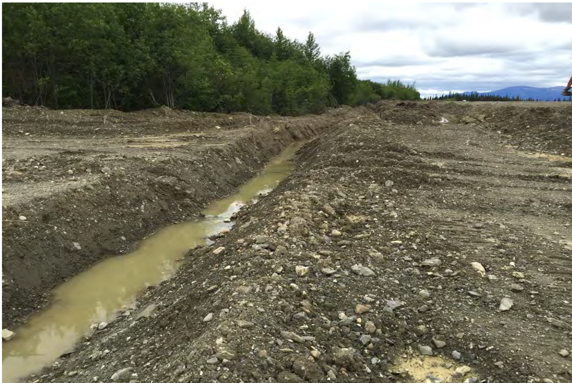
Photo 11: Temporary drainage ditch to manage water during cover placement
