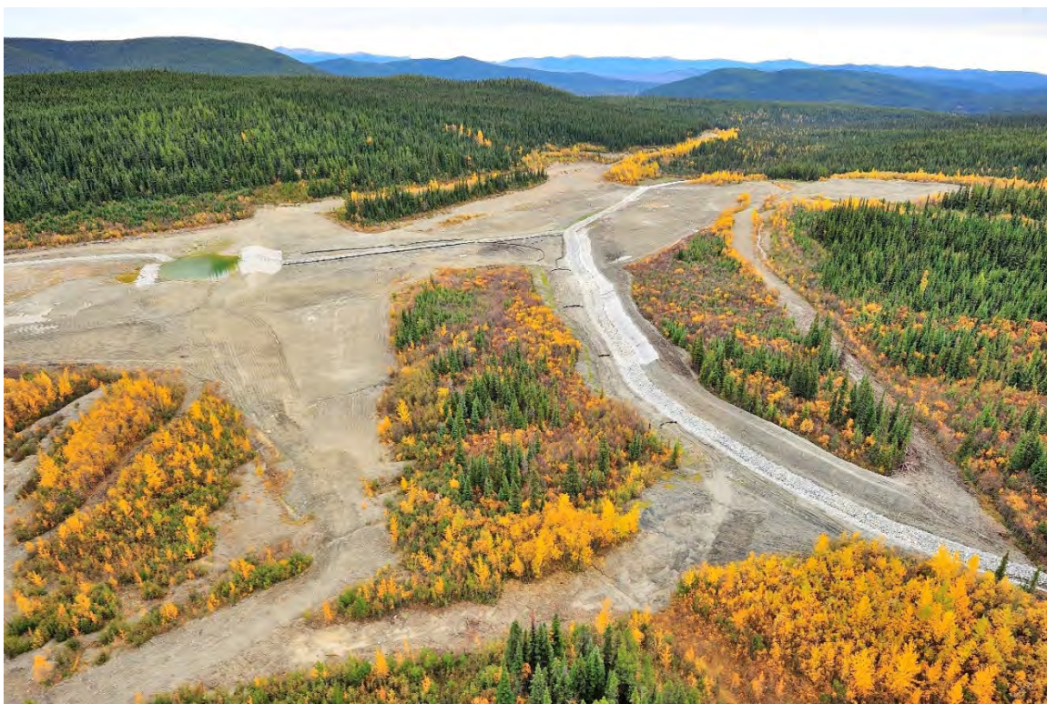
Photo 3: View east over the Sediment Retaining Structure
