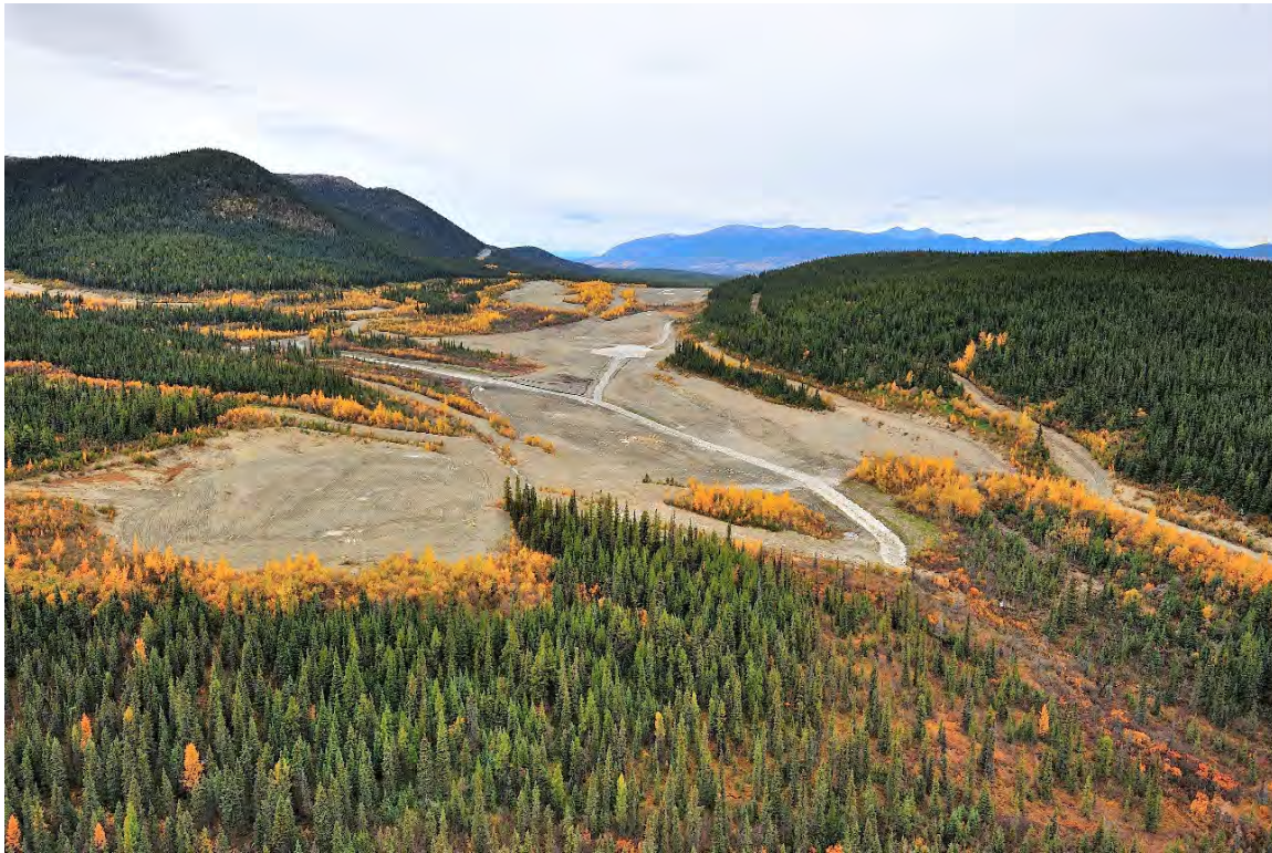
Photo 4: View North of the new Camp Creek Drainage Channel
