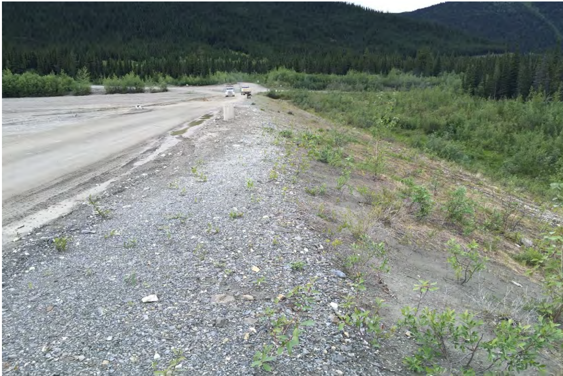
Photo 6: View looking west along the North Dam showing the downstream slope
