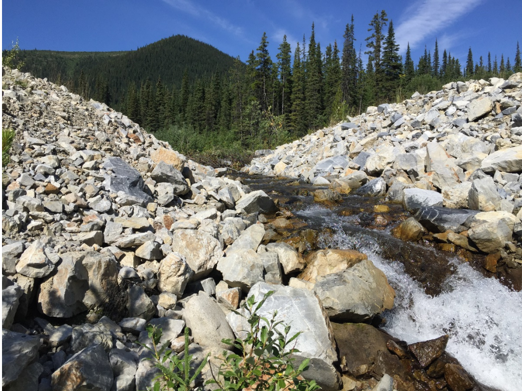
Photo 15: View looking upstream of the North Creek Dyke
