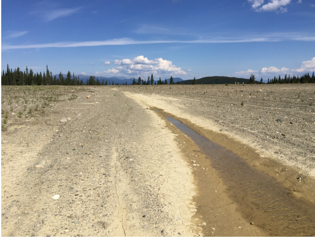
Photo 11: Drainage channel looking north
