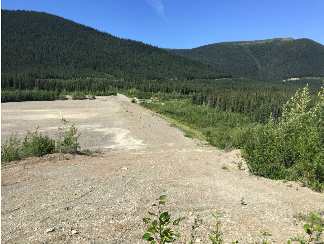
Photo 1: North Dam Crest looking west
