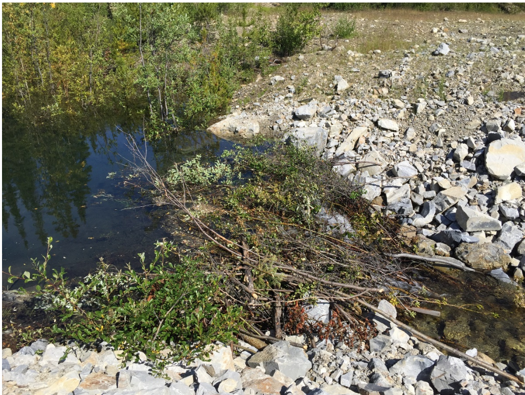
Photo 12: Beaver dam at inlet to North Creek crossing
