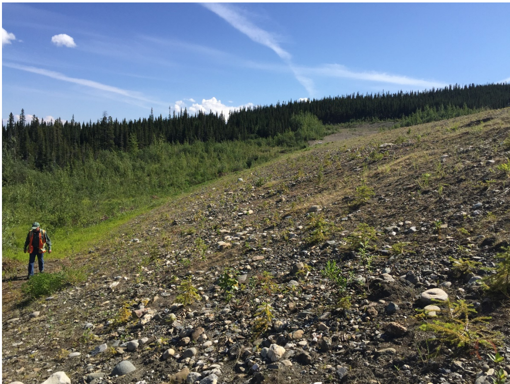
Photo 2: Downstream slope of the North Dam. Oversized trees have been removed
