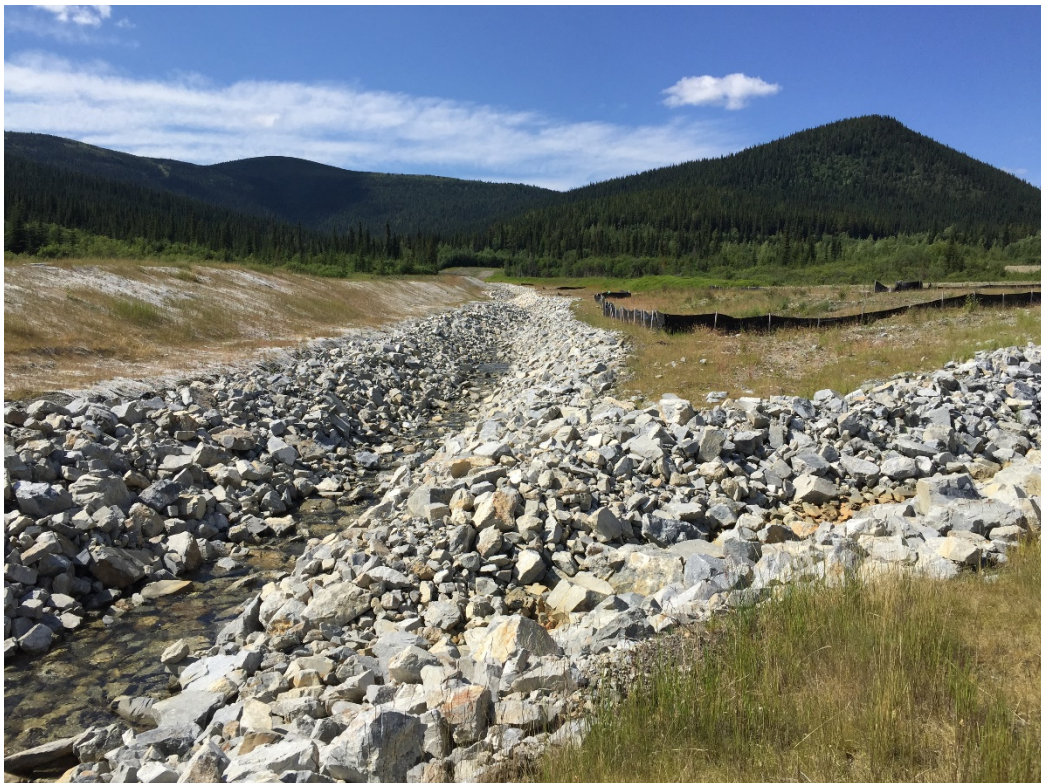
Photo 22: View upstream of the Camp Creek channel
