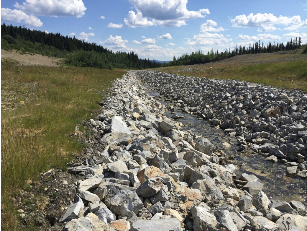
Photo 23: View south of the Camp creek drainage channel
