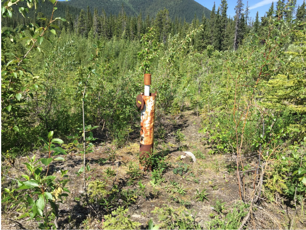
Photo 3: North Dam Piezometer at toe NDW 4A
