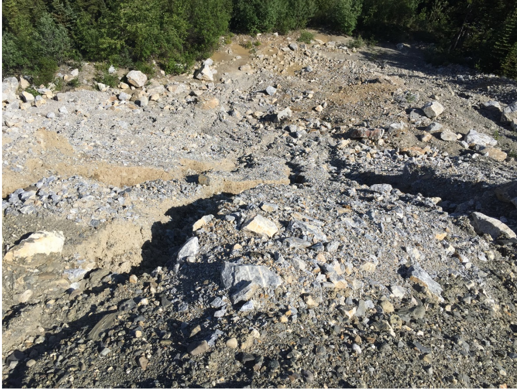
Photo 25: Erosion gullies at toe of Jewelbox Waste rock dump
