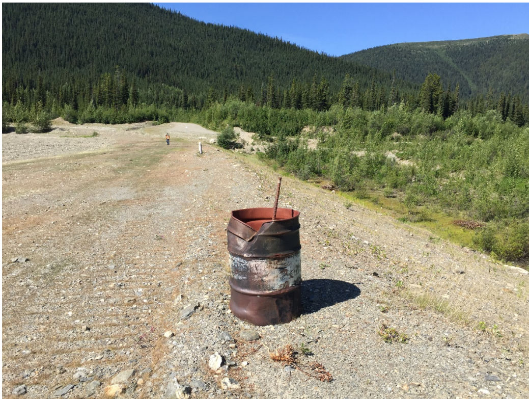
Photo 8: Slope Displacement pin on north edge of Dam (redundant)
