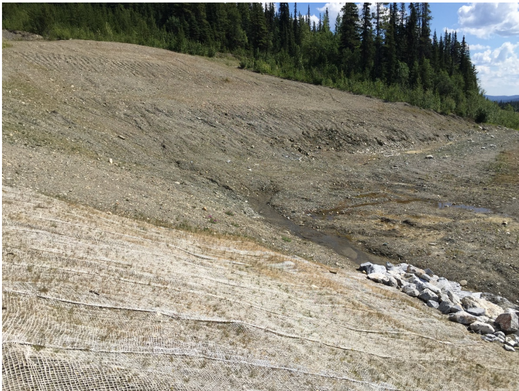
Photo 18: Hillside seepage along D/S toe of dyke
