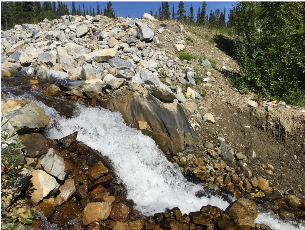
Photo 14: Outlet of North Creek crossing
