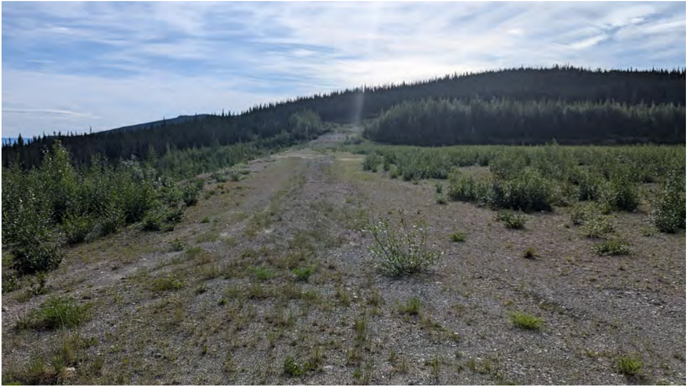
Photo NE-01: North Embankment alignment seen from the west abutment; it shows no abnormal deformation.
