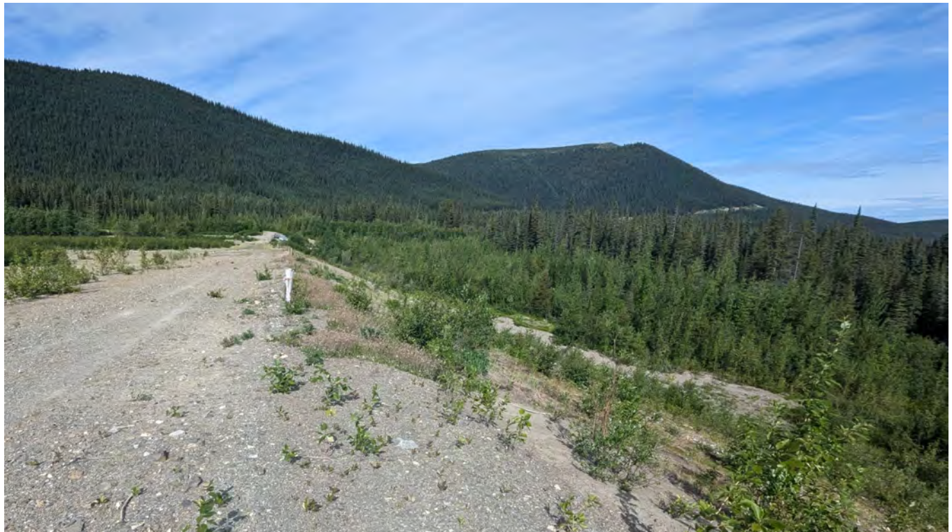
Photo NE-02: A closer look to the North Embankment crest seen from the east abutment.
