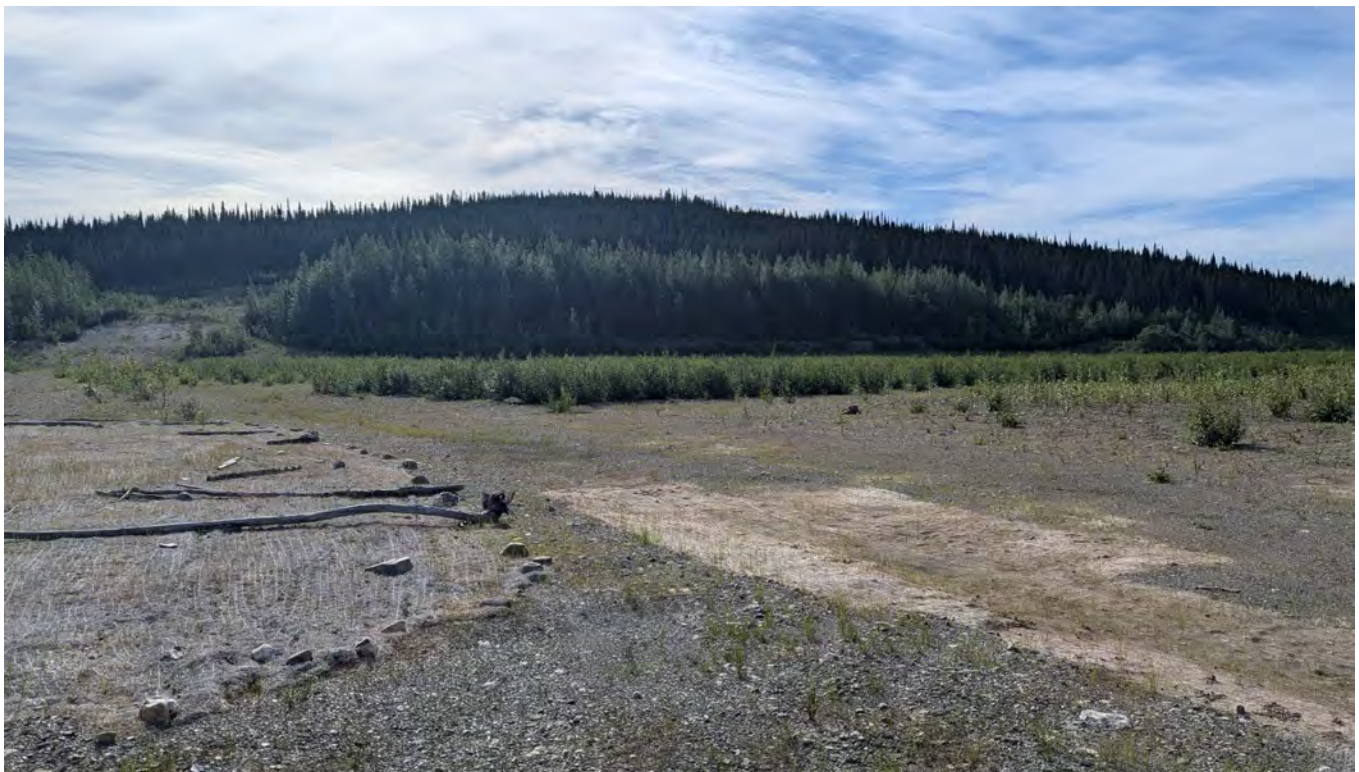
Photo NE-08: North Embankment gully repair erosion control blanket.
