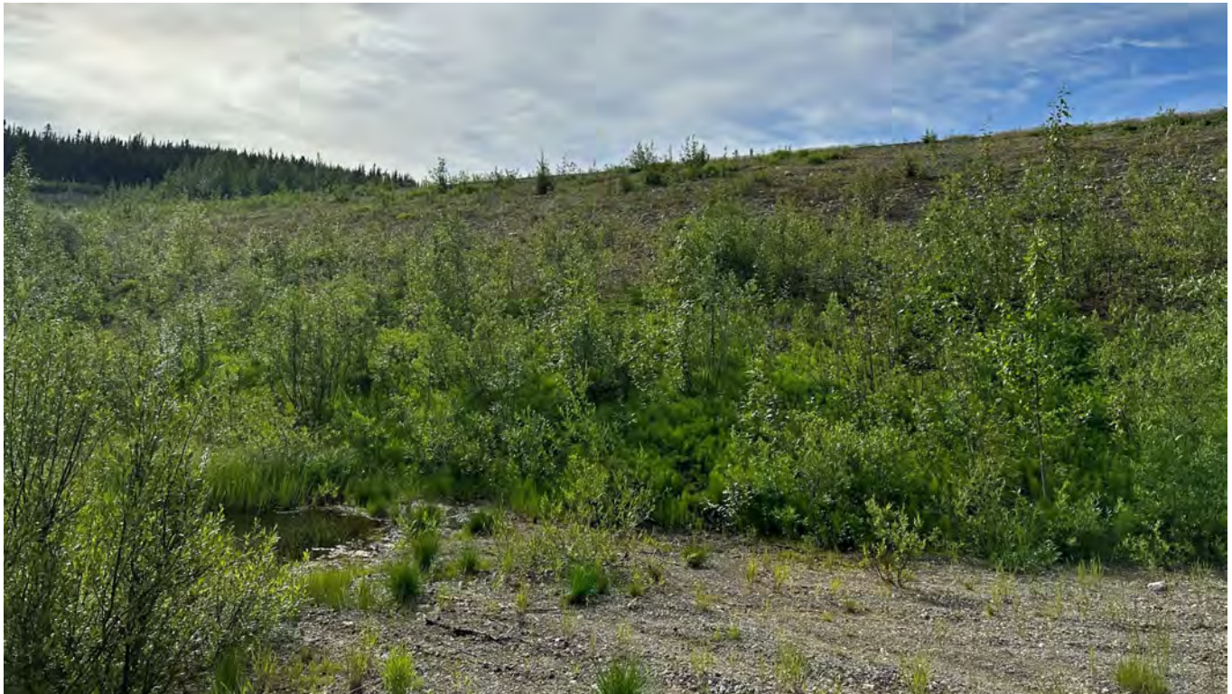
Photo NE-06: North Embankment downstream slope vegetation seen from the toe.
