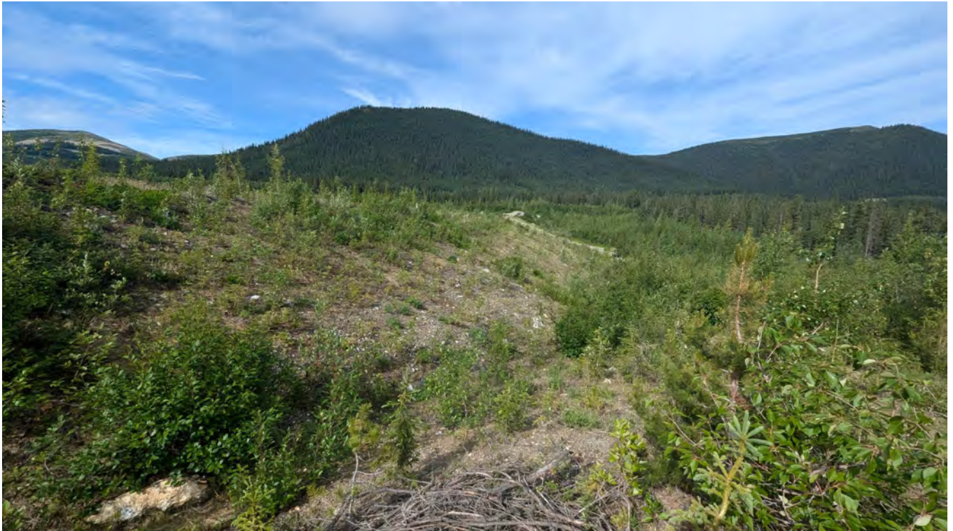
Photo NE-05: North Embankment downstream slope vegetation seen from the east abutment.
