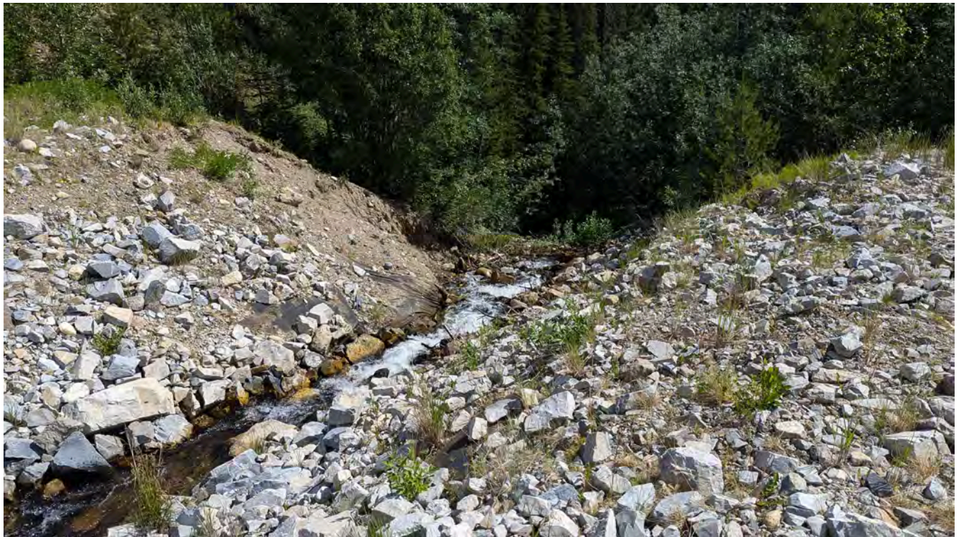
Photo NC-04: Downstream end of the decommissioned North Creek Dyke.
