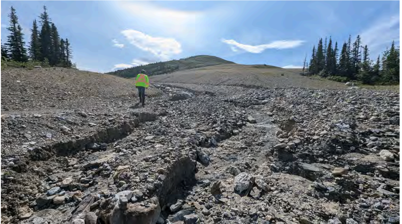
Photo WR-05: Erosion at the lowest point of the Jewelbox Waste Rock Dumps through the former Jewelbox Haul Road (looking southeast).
