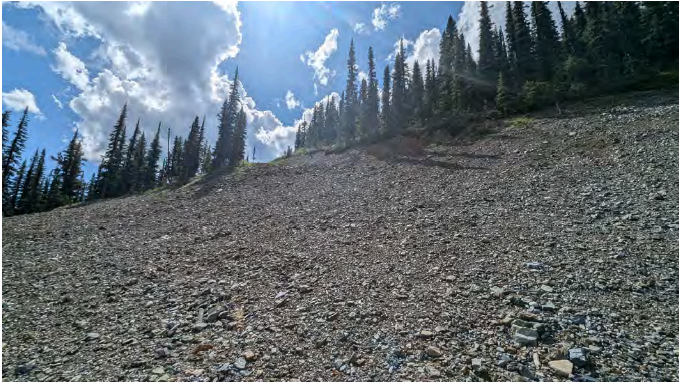
Photo WR-15: Regraded 1300 Portal Waste Rock Dump and 1300 Portal area.
