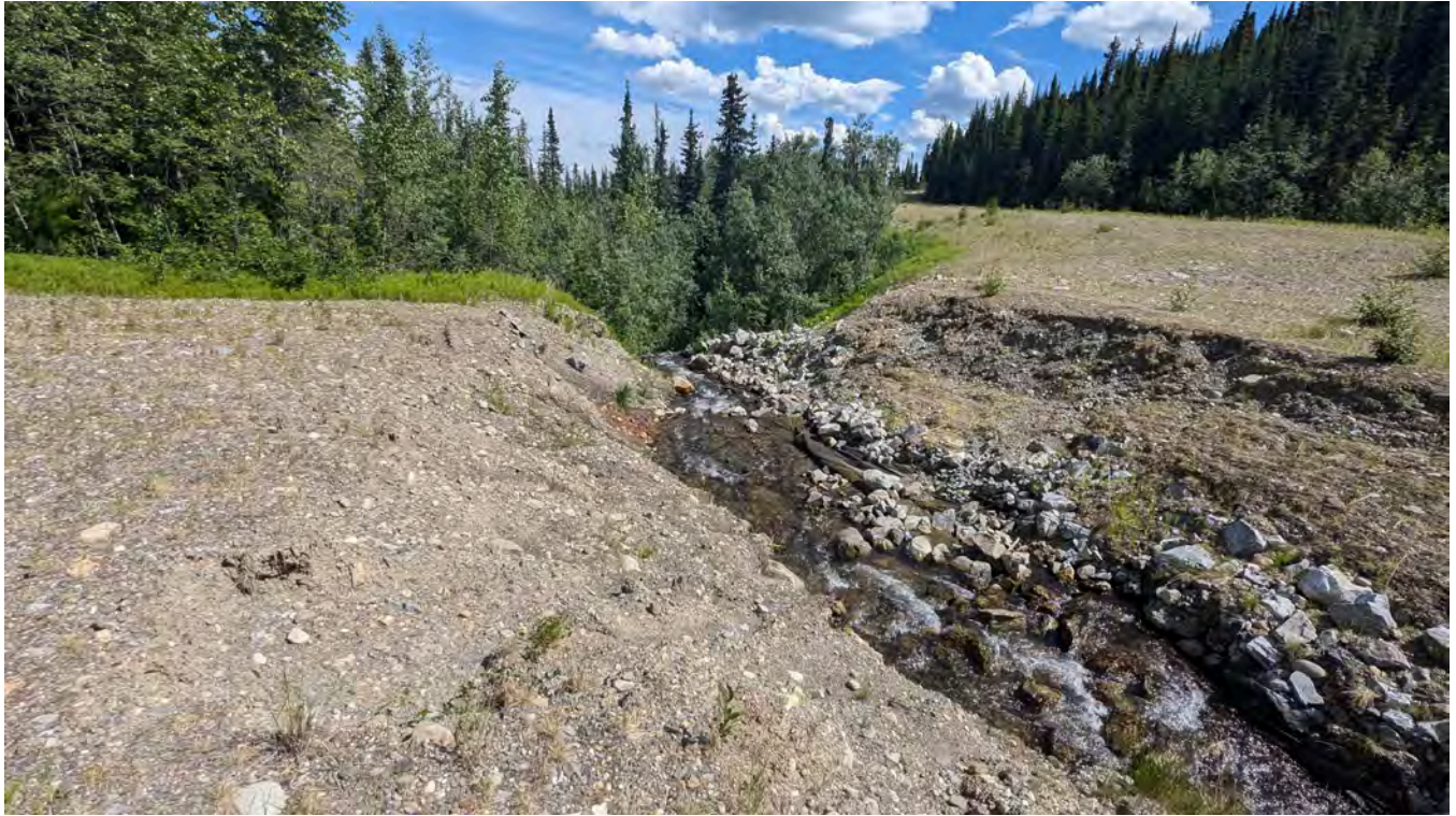
Photo NC-01: Decommissioned Access Road Crossing to Burnick Zone looking south.
