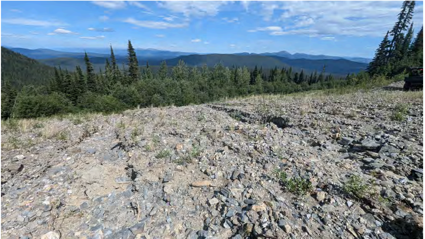
Photo WR-03: Erosion gullies crossing the decommissioned access road to the Jewelbox and Main Zone.
