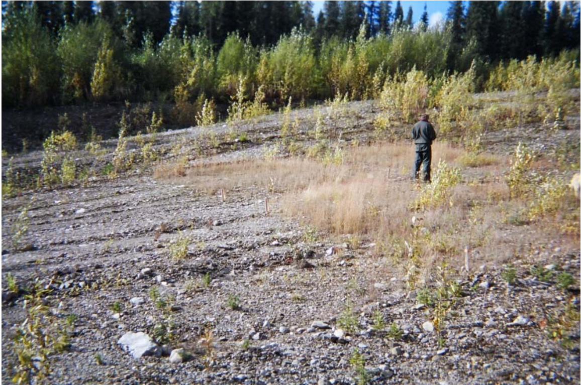
Km 22 Main Access Road
