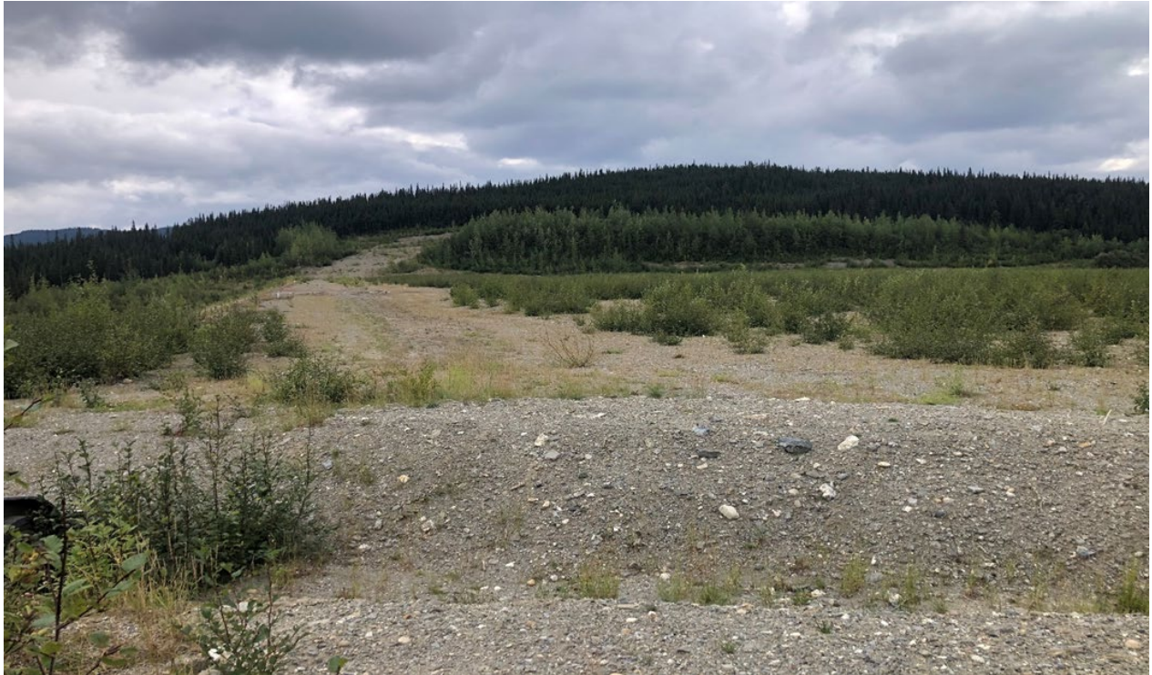
North Dam and Tailing area looking east: Latitude 60.53885° Longitude 128.85624°
