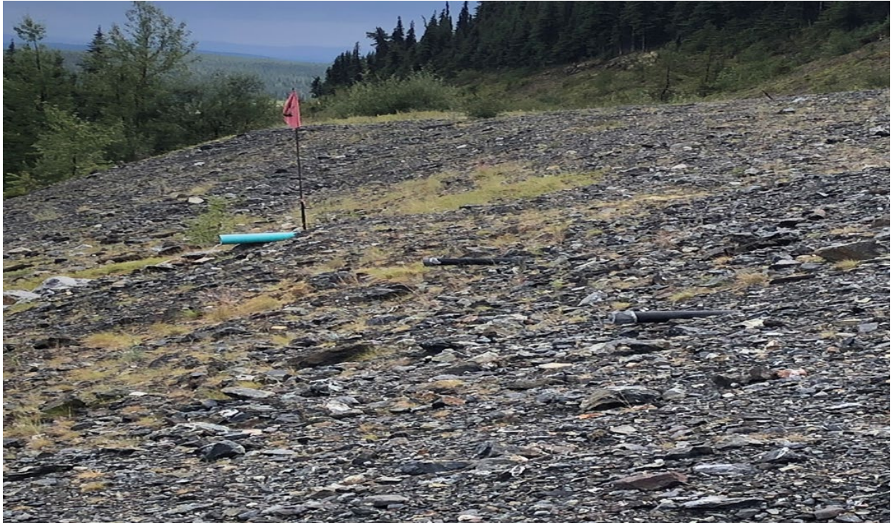
Looking East towards three portal drains
