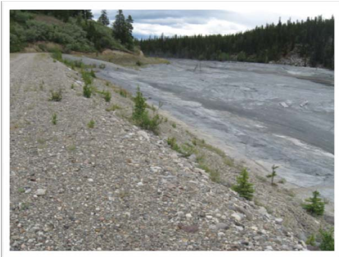
Figure 25 A-Valley Impoundment Upstream of A-Dam from WP 169
