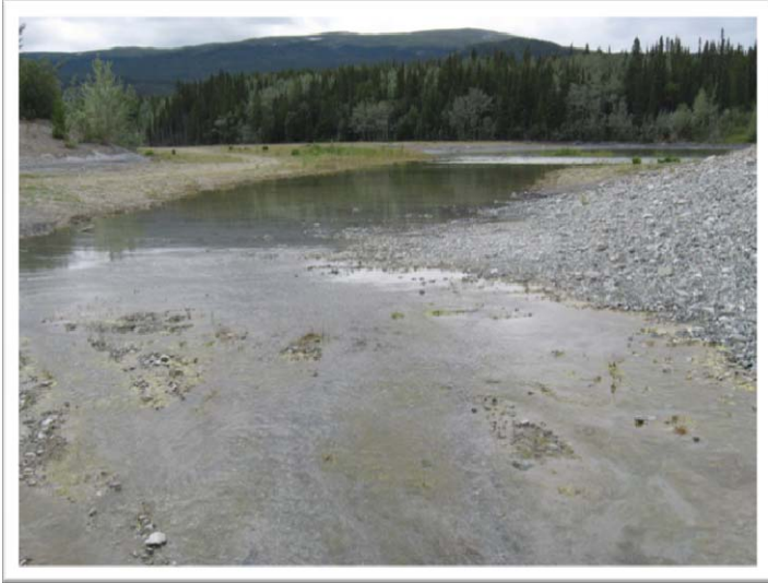
Figure 35 Entrance to Spillway from B Pond from WP 175
