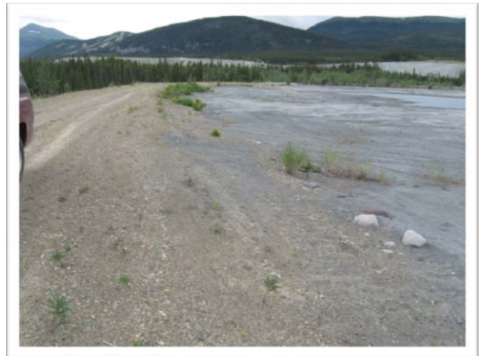
Figure 16 Dyke Crest and Upstream Tailings at WP 160
