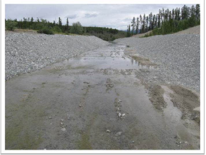
Figure 36 View D/S Along Spillway Chute from WP 175
