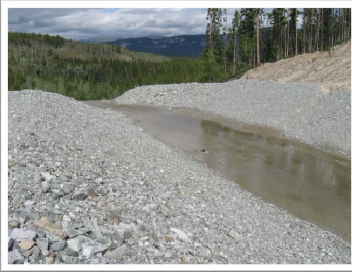
Figure 37 D/S End of Spillway Chute at Drop Section from WP 212
