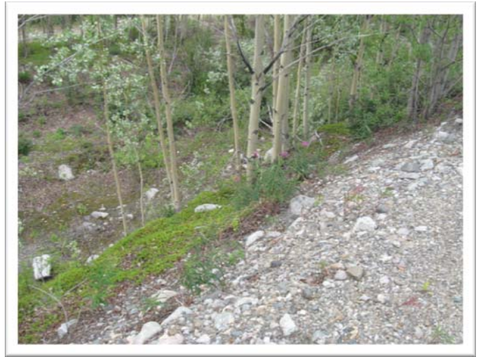
Figure 05 Berm Along D/S Toe at WP 117
