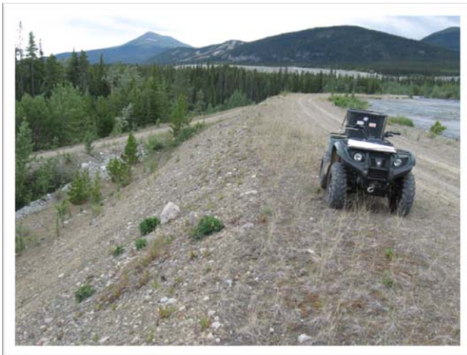
Figure 15 Downstream Face at WP 160
