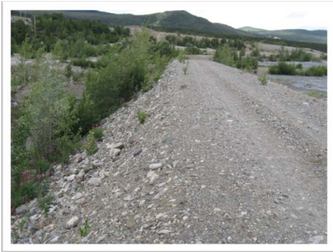
Figure 02 D/S Face at WP 116 (View NW)
