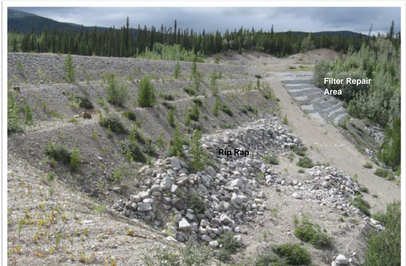
Figure 29 Downstream Side of B-Dam from WP 213, View SW
