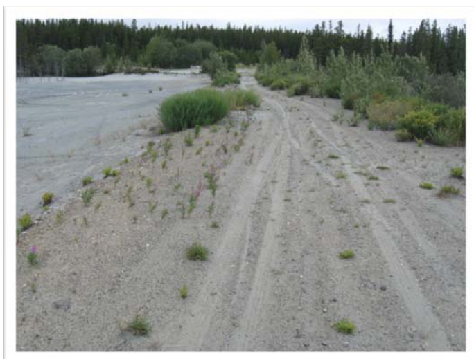
Figure 17 Dyke Crest and U/S Tailings at WP 168 (View NW)
