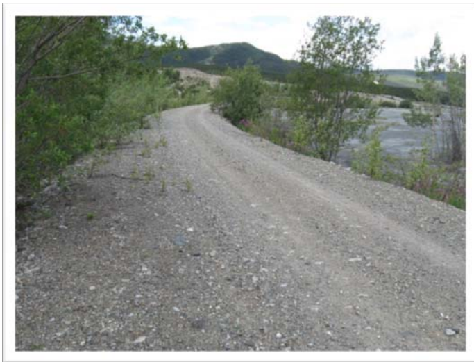
Figure 04 View W Along Dyke from WP 117
