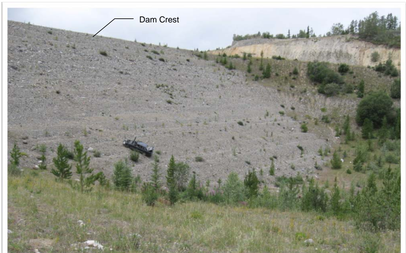
Figure 24 View at Downstream Slope from East Abutment at WP 170
