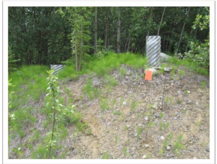
Figure 11 CMPs at Toe of Dyke
