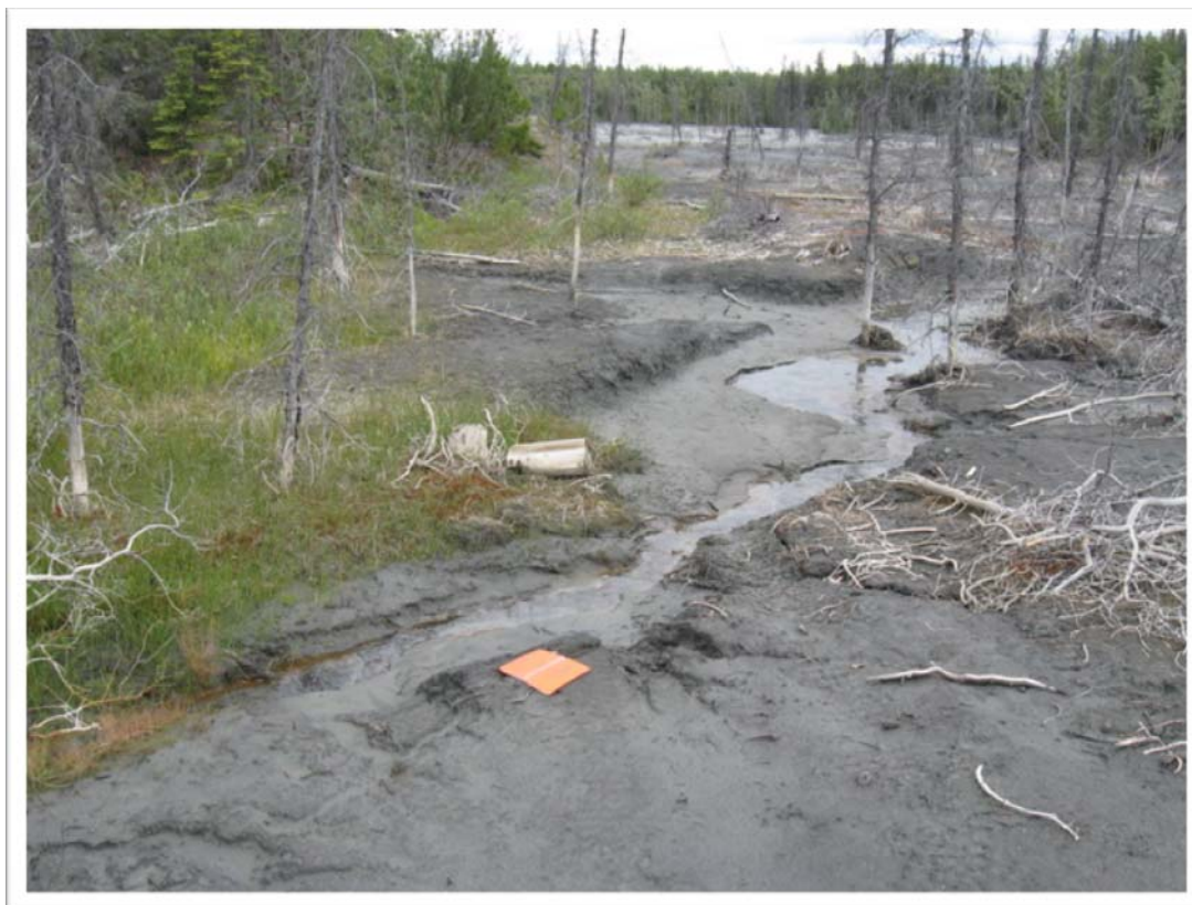
Figure 23 Seepage Water Downstream of Perimeter Dyke at WP 167, View N
