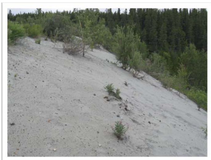
Figure 18 D/S Dyke Face at WP 168 (View NW)
