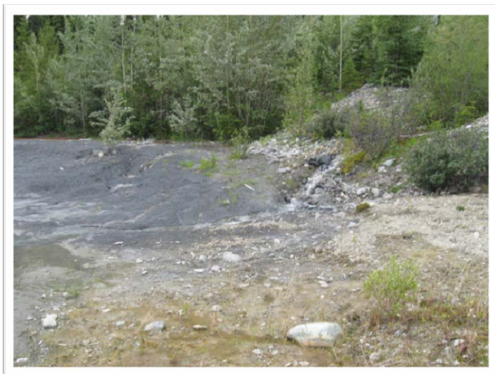
Figure 32 Drainage Ditch Outlet into Tailings Pond from WP 183
