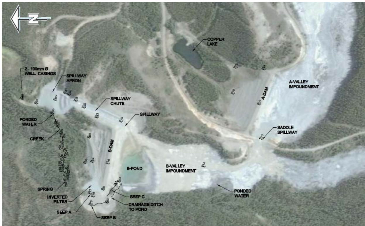
a. Aerial view
