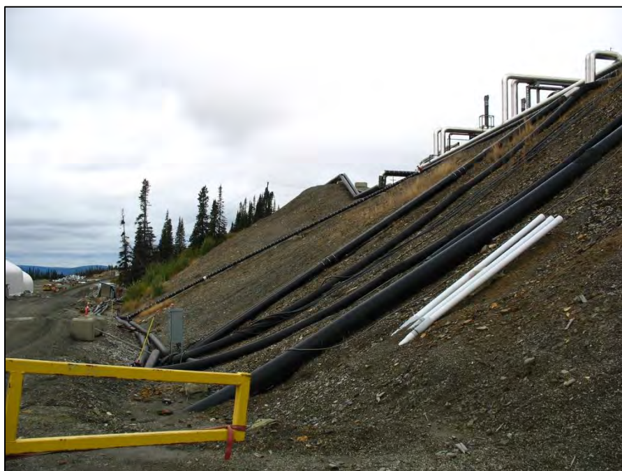
PHOTO 42 – Downstream Slope of the Genset Pad
