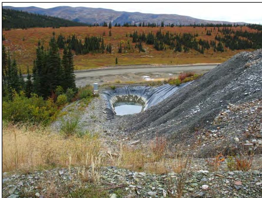
PHOTO 55 – Waste Rock and Ore Storage Facility runoff collection sump
