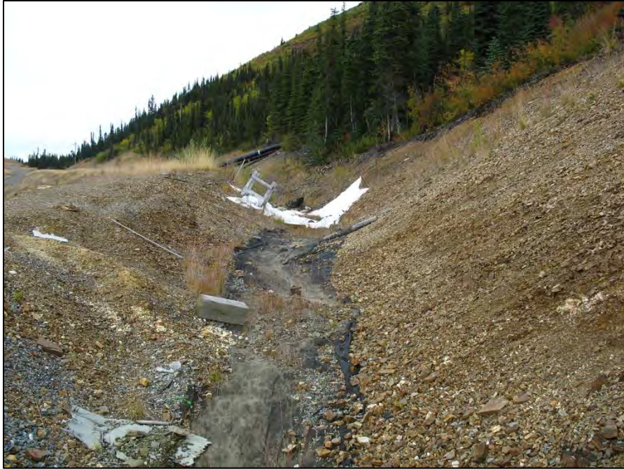
PHOTO 47 – Ditch 1 – Minor debris in ditch bottom.
