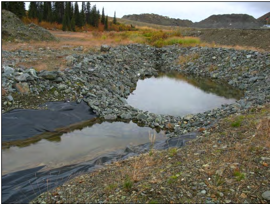
PHOTO 30 – Stilling Basin and upstream end of Ditch A.
