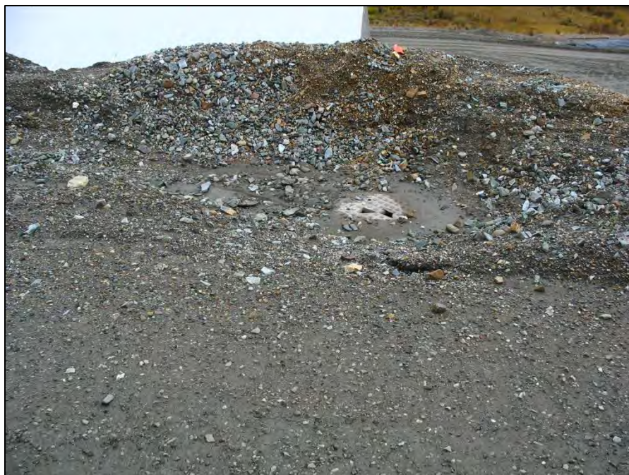
PHOTO 41 – Manhole upstream of MSE Wall
