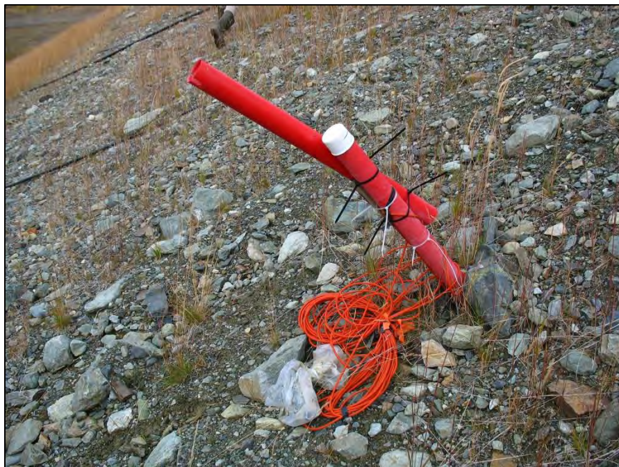
PHOTO 6 – TSF South Embankment – Damaged inclinometer – no longer functioning.
