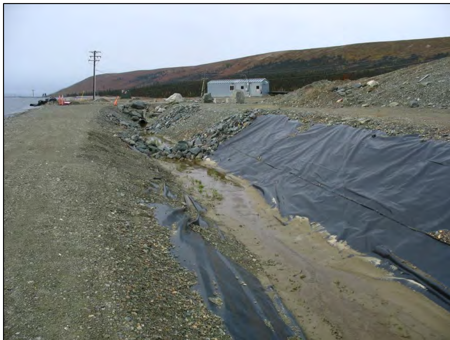
PHOTO 26 – Ditch A at north side of TSF – Looking west.
