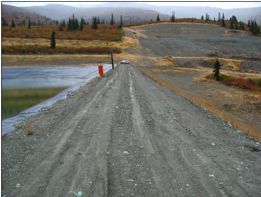
PHOTO 2 – TSF South Embankment – Looking east.
