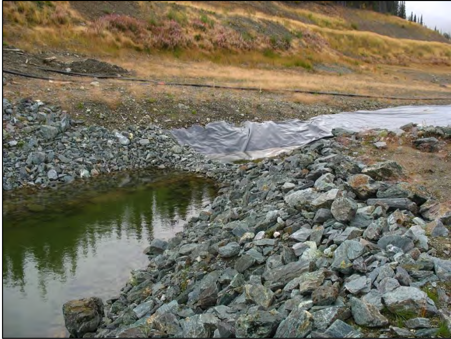
PHOTO 31 – Stilling Basin and upstream end of Ditch A. Stilling Basin unlined.
