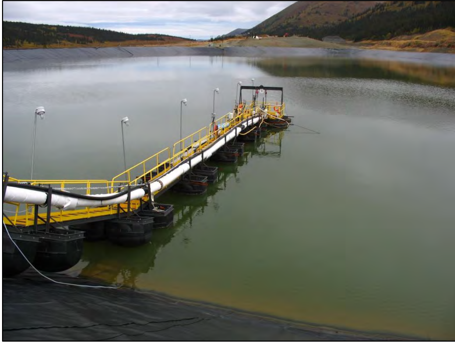
PHOTO 3 – TSF South Embankment – Reclaim barge.
