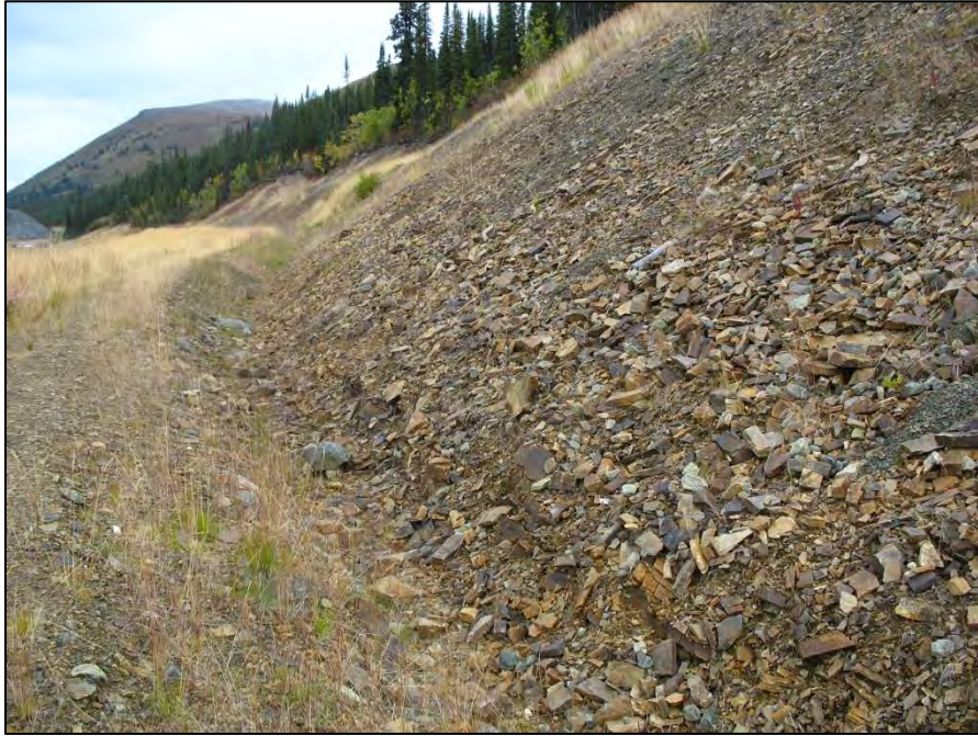
PHOTO 29 – Ditch B on east side of TSF - Looking north.
