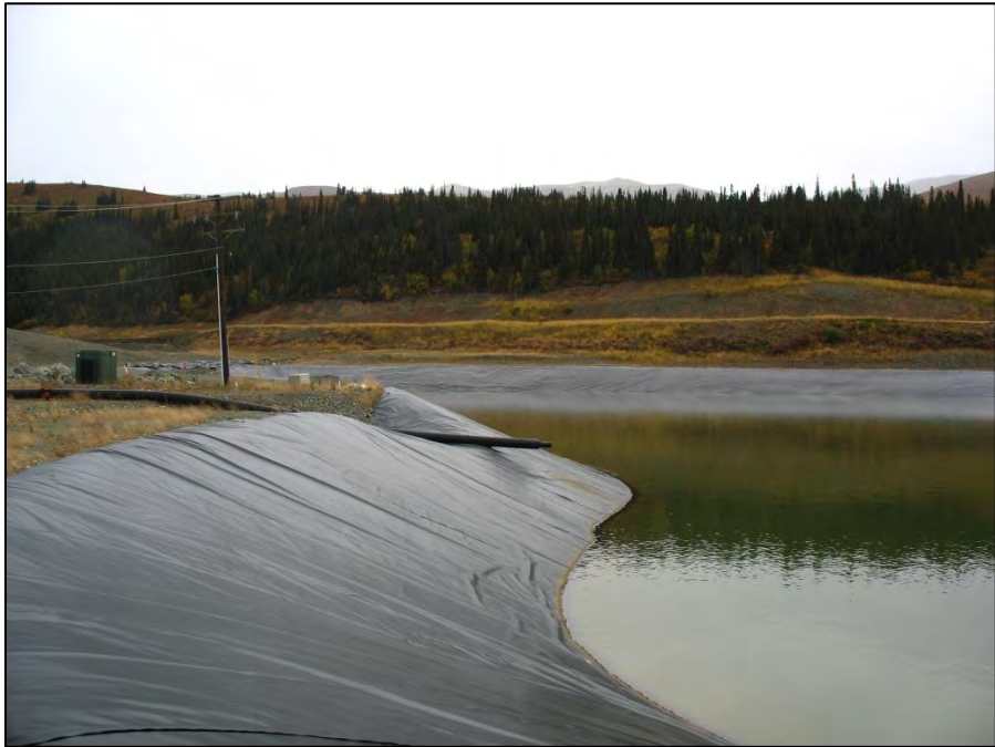
PHOTO 13 – TSF upstream slope near spillway.
