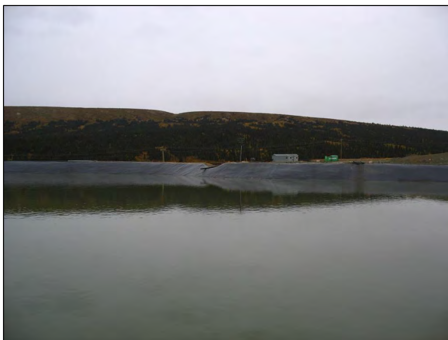
PHOTO 22 – TSF spillway looking west.
