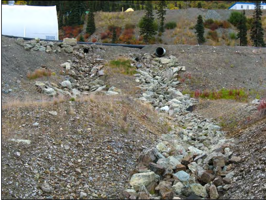
PHOTO 49 – Drainage from Mill Pad.
