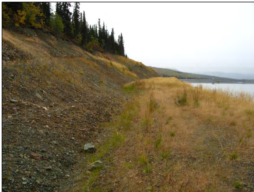
PHOTO 28 – Ditch B on east side of TSF - Looking south.
