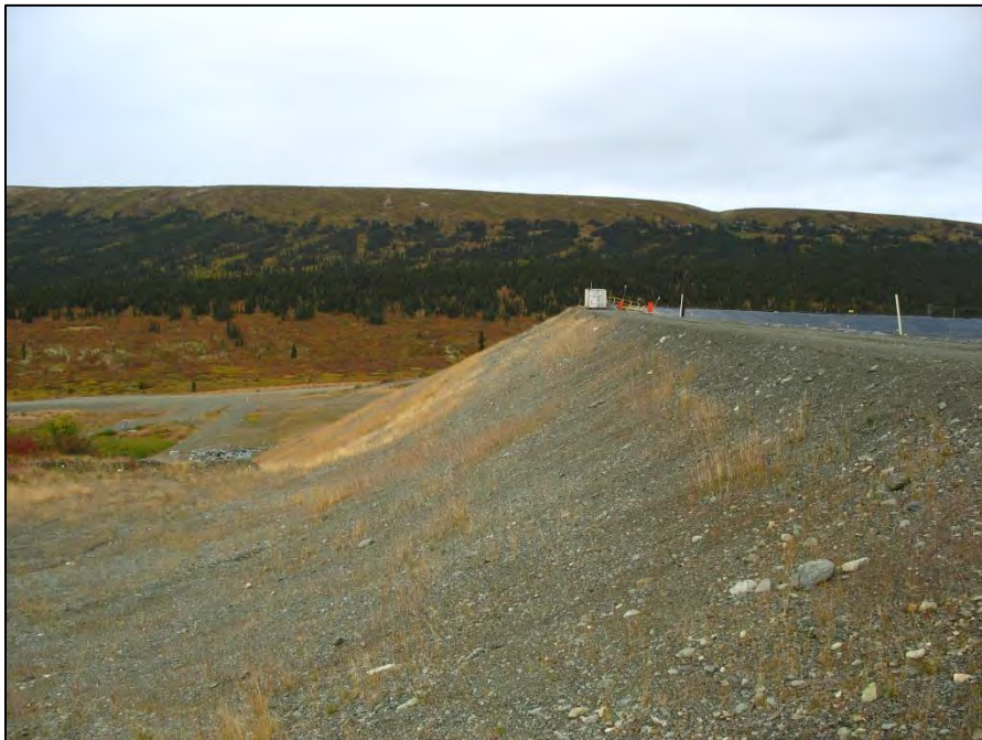
PHOTO 4 – TSF South Embankment – Downstream slope.
