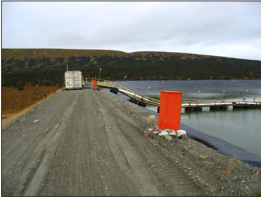
PHOTO 1 – TSF South Embankment – Looking west. Piezometer readout box in foreground.
