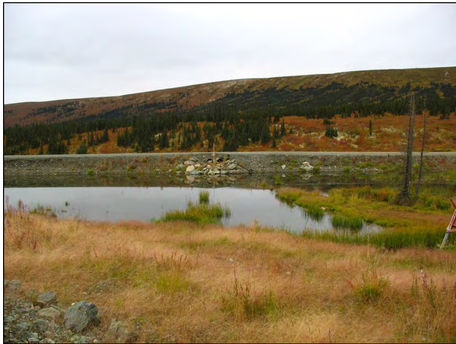
PHOTO 25 – TSF Seepage Collection Pond looking west towards culverts.
