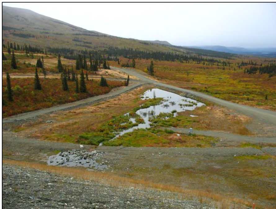
PHOTO 23 – TSF Seepage Collection Pond.
