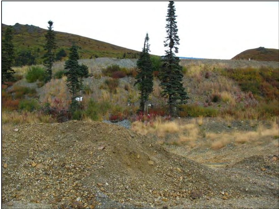
PHOTO 52 – Camp Pad with repaired erosion gully
