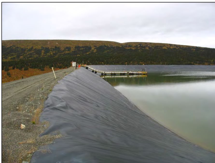
PHOTO 9 – TSF South Embankment – Upstream slope.
