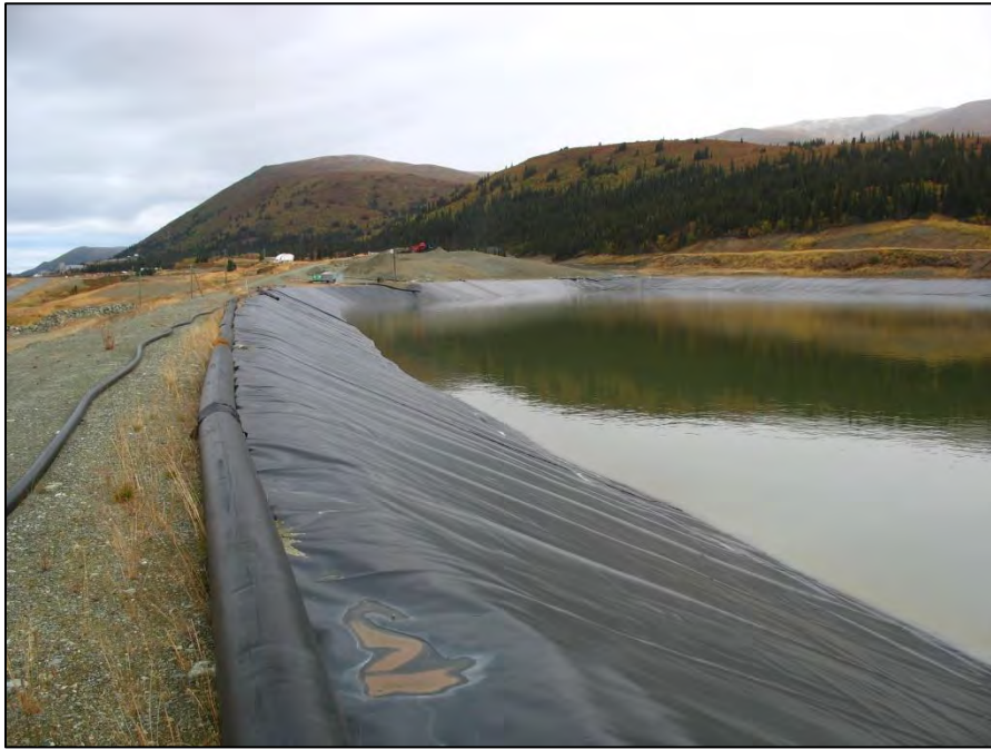
PHOTO 11 – West Side of TSF – Upstream slope.
