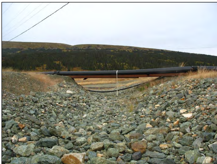
PHOTO 21 – TSF spillway channel looking downstream.
