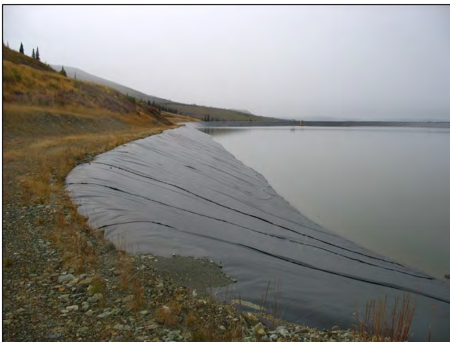
PHOTO 20 – East side of TSF - Looking south.
