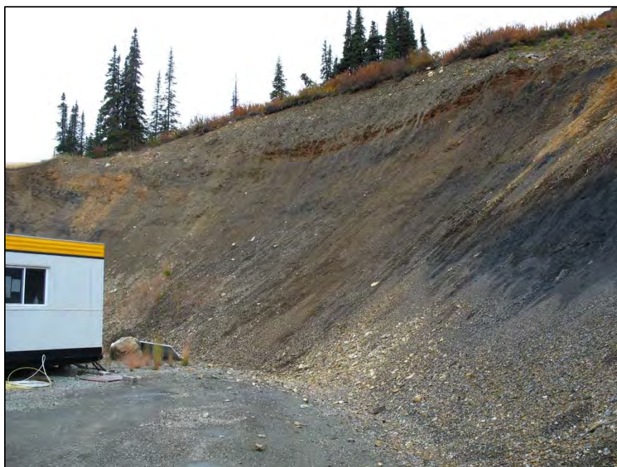
PHOTO 56 – Slope behind Vent Raise and Underground Office
