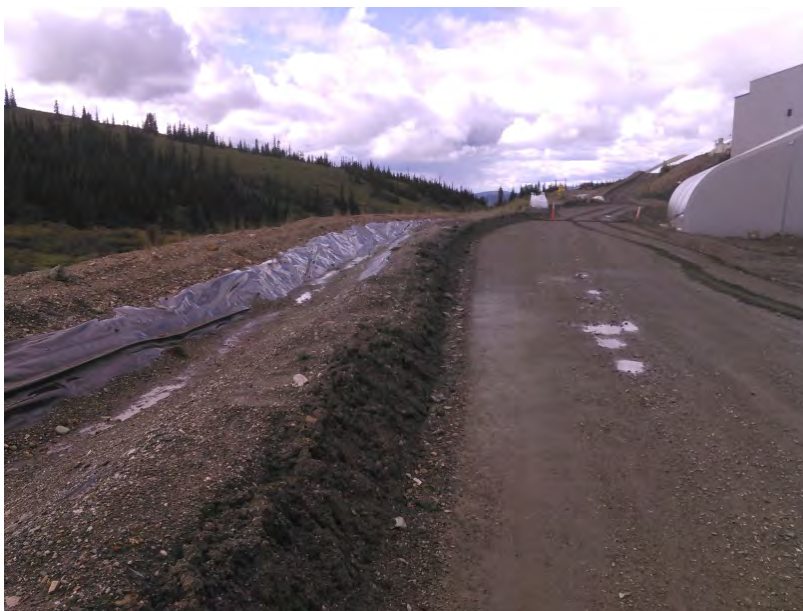
Figure 16 – Ditch #3 looking west towards Sump #2.
