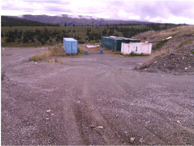
Figure 23 – Sewage Treatment Facility looking west.
