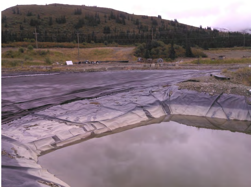
Figure 34 – Land Treatment Facility (LTF) Pad and sump looking east.
