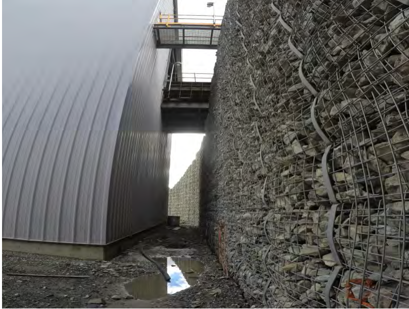
Figure 7 – MSE wall behind crusher.
