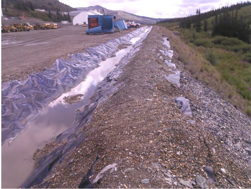
Figure 17 – Ditch #4 at the edge of site storage pad looking east.
