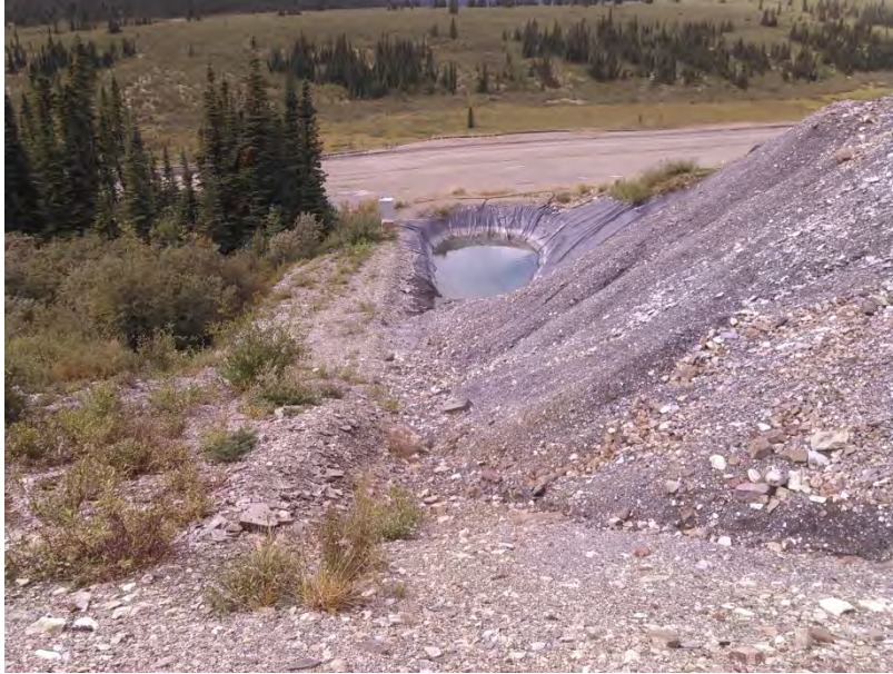
Figure 25 – Waste Rock Pad #1 sump and liner located in the South West corner of the pad. Sump level is controlled by a float and pump system.
