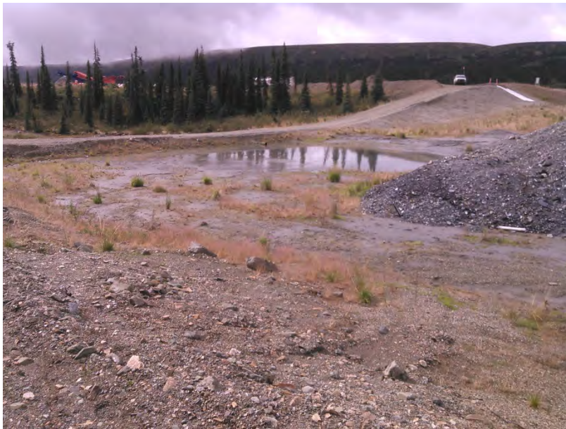
Figure 28 – Waste Rock Pad #2 settling pond located at the south end of the pad. Settling pond is discharged through the Bio Reactor.
