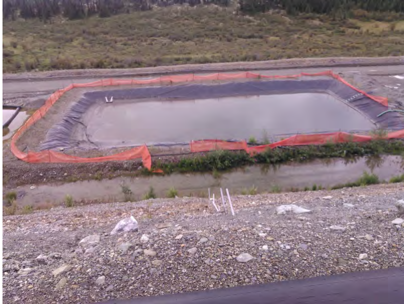
Figure 13 –Sump #5 as seen above from the Mill Pad.
