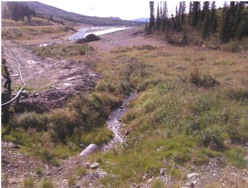
Figure 32 – Diversion Ditch A head waters parallels bio-reactor channel and drainage from Waste Rock Pad #2.
