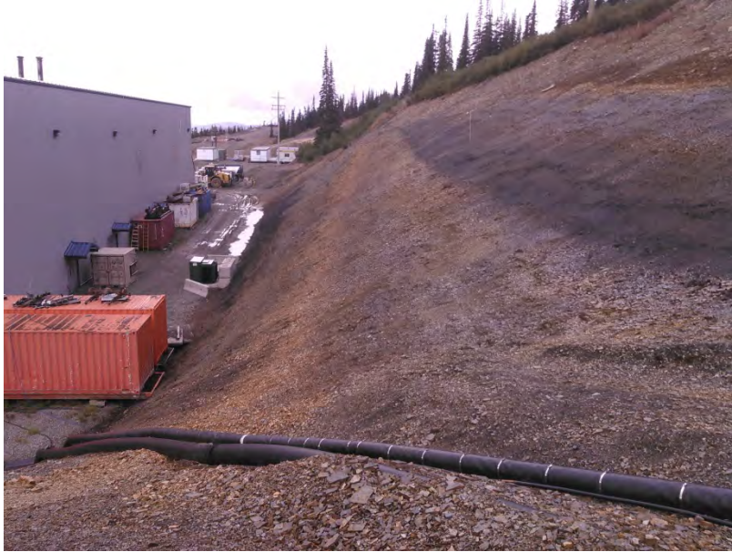
Figure 35 – Cut slope behind Truck Shop looking north.
