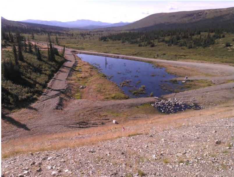
Figure 30 – Seepage Pond as seen from the TSF facing south.
