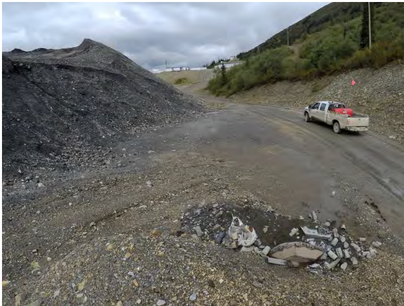
Figure 26 – Waste Rock Pad #1 berm isn't continued past the waste pad access ramp.
