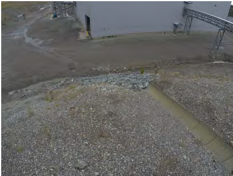
Figure 8 – Culverts and rip rap leading from Generator Pad to Ditch #5.
