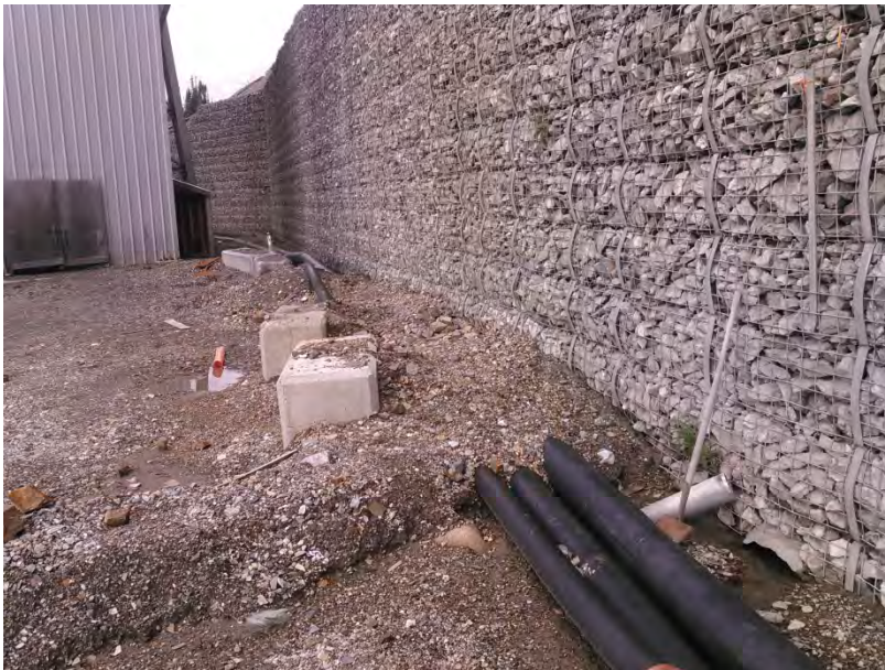
Figure 18 – Outfall of Ditch #5 at base of MSE wall.
