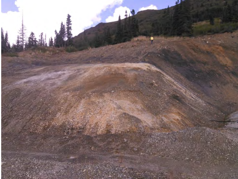
Figure 37 – Cut slope above the Vent Raise looking North East.
