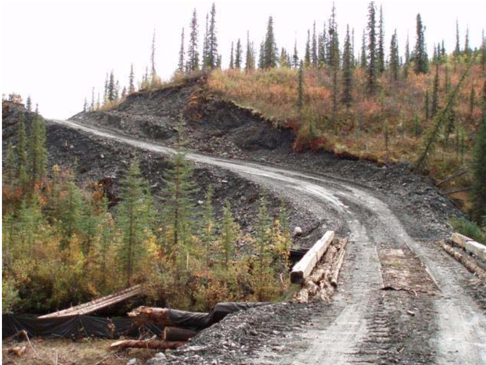
Picture 2-11 Bunker Creek temporary bridge, looking south.
