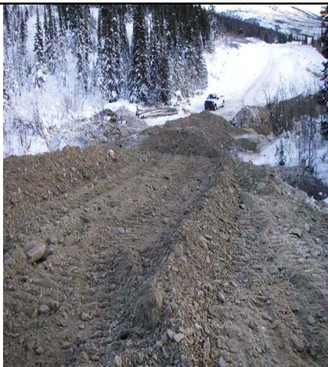
Photo 3 - 12/06/07 - Grading road and fill on culverts; looking SE
