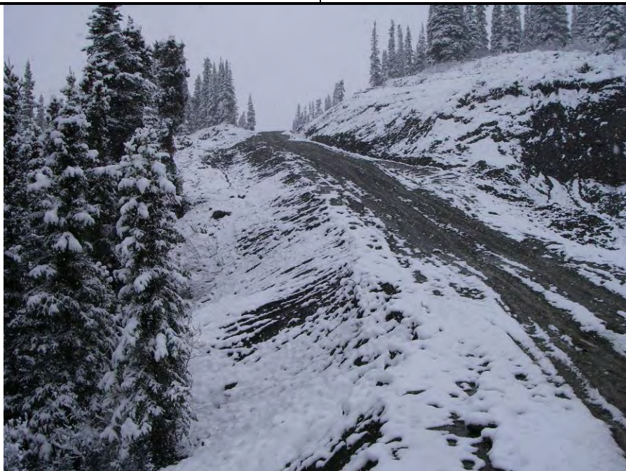
17/05/07 Bank on lower side of road leading into exploration camp; facing NW
