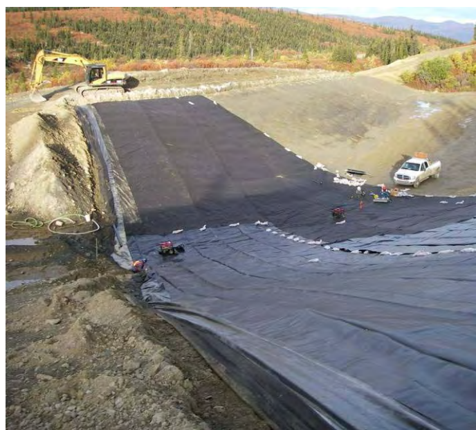
09/09/07 Rolling out the Enviro Liner over the geotextile fabric (facing W)
