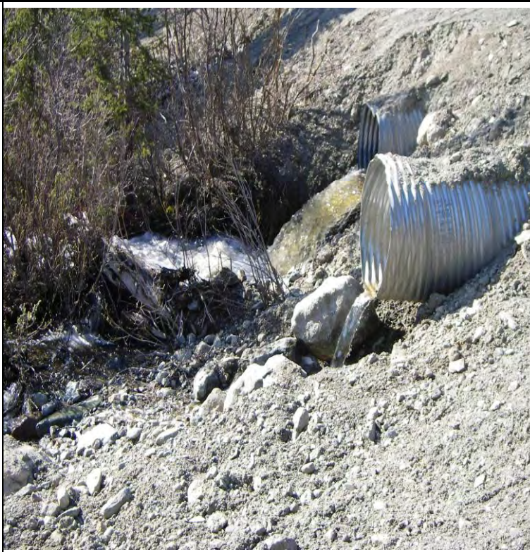
05/26/07 Culvert flow from Campbell Creek; facing N
