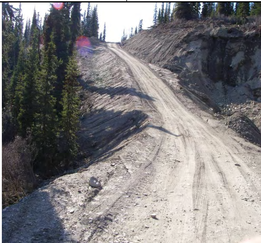
27/05/07 Bank on lower side of road leading into exploration camp; facing NW
