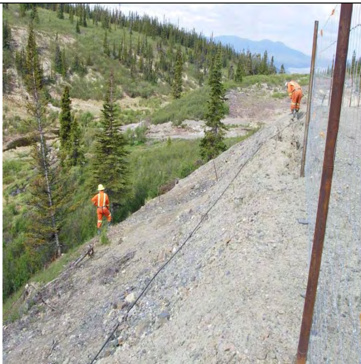
06/21/07 West bank being investigated by geotechnical engineer (below); facing NNE
