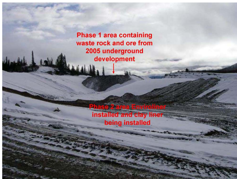
Picture 2-15 Temporary waste rock and ore storage facility (October 2007)
