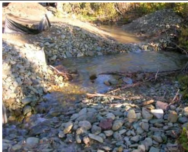
08/27/07 Cobble installed at Campbell Creek; facing N
