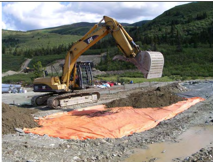
Photo 2 07/26/07 Placing clean soil over the flattened and tarped contaminated material; facing north
