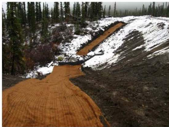
Image 1277. View of the outlet channel during installation of erosion control matting on northwest bank.
