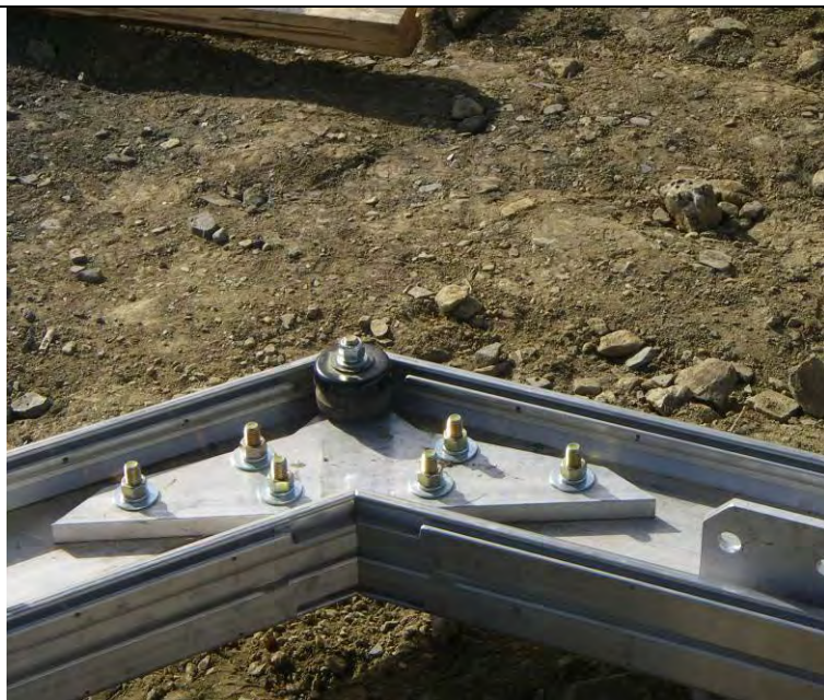
09/13/07 Corner brace nut & bolt assembly
