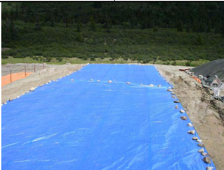
Photo 3 07/26/07 Final tarped cell; facing east
