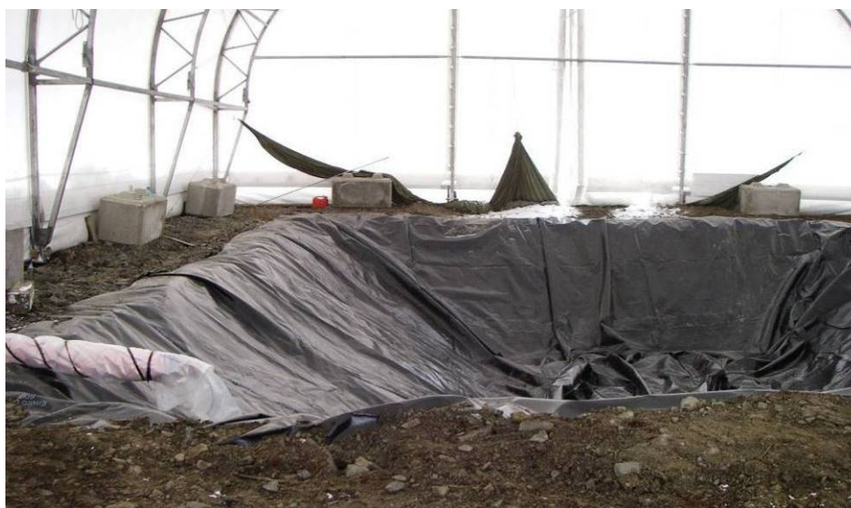
Picture 2-12 Completed CDS (September 24 th , 2007)
