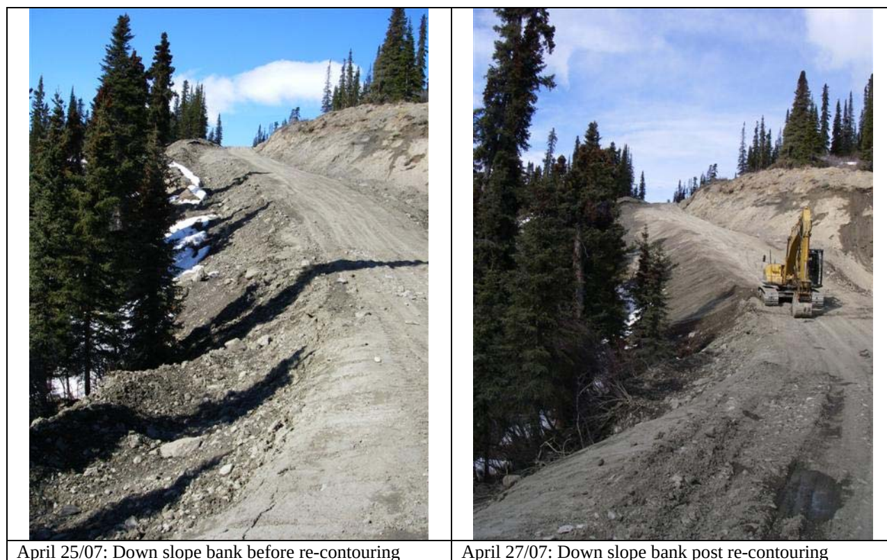
Picture 4-2 Bank re-contouring down slope of the road through the Campbell Creek gorge (west side)
