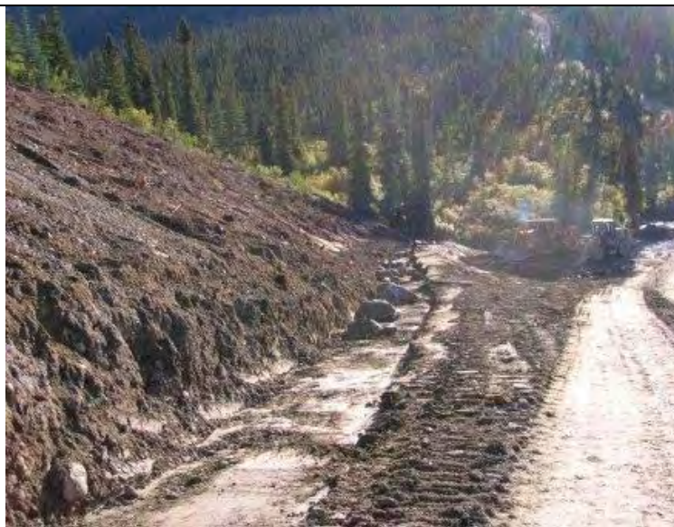
08/27/07 Ditching and organic placement at borrow source at gorge; facing SE
