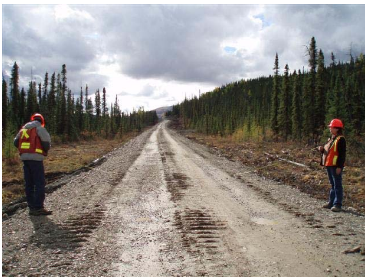
Picture 2-1 Access Road near km 3, heading south towards the mine site.
