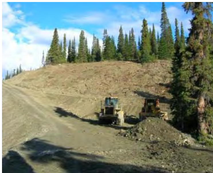
08/27/07 Re-contouring of borrow source; facing N
