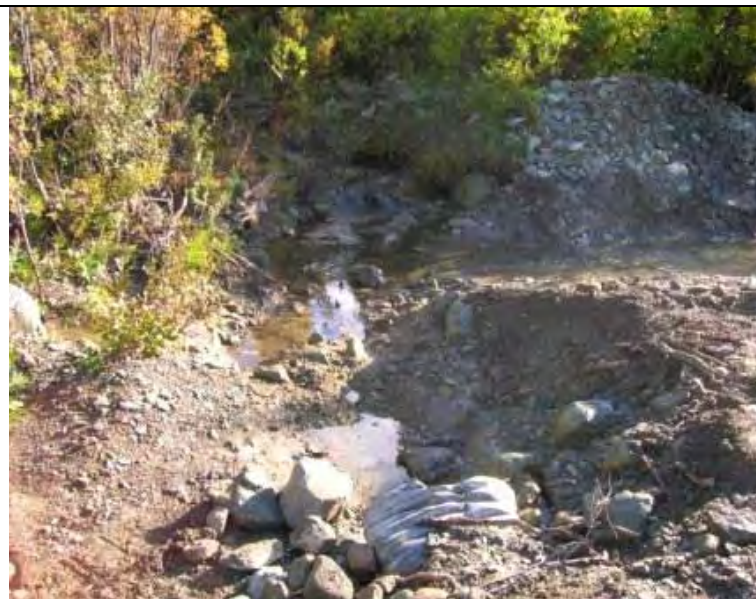
08/27/07 Culvert inlet at Campbell Creek prior to cobble placement
