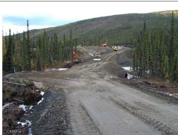
Image 1220. Final view of Putt Creek crossing, facing east.
