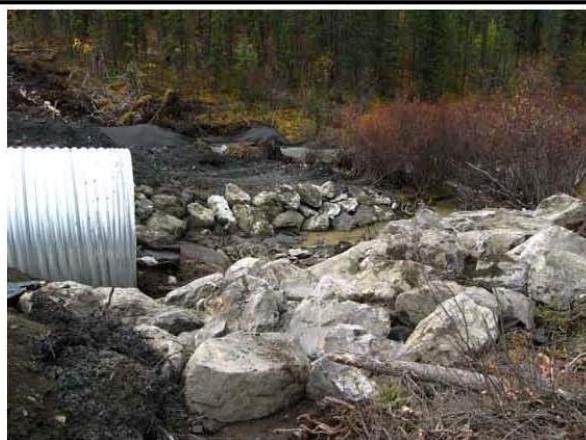
Image 1166. Completion of riprap work around outlet of culvert prior to release of creek water.
