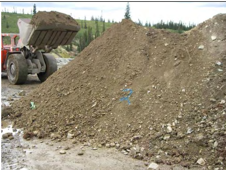
07/26/07 Stock piling the removed soil; facing W
