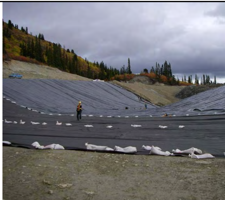
09/10/07 Laying the geotextile and Liner (facing E)
