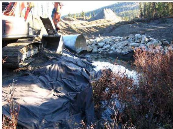
Image 1201. Culvert inlet channel following release of creek. West bank being prepped for riprap.
