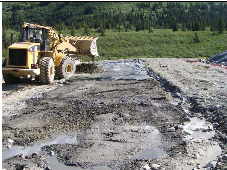
Photo 1 07/26/07 Placing clean soil over the flattened and tarped contaminated material; facing east
