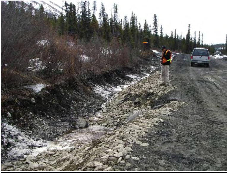
Installation in progress, view looking east
