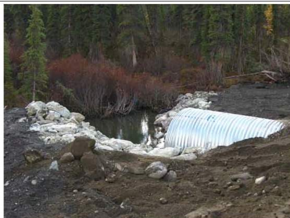
Image 1217. Final riprapped inlet channel.
