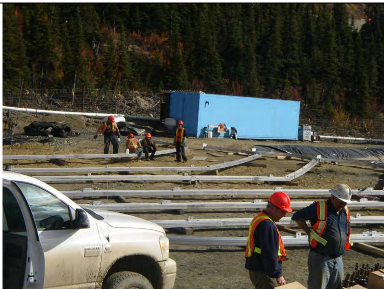
09/13/07 Initial set-up of 80' x 90' frame (facing E)
