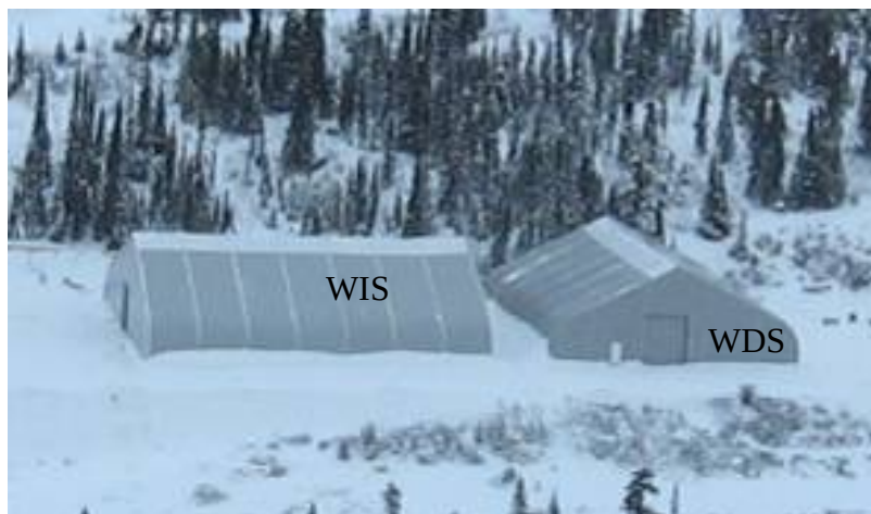
Picture 2-13 Completed Sprung Structures over the WIS and WDS (October 2007)
