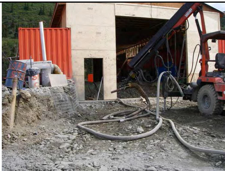
07/28/07 Shotcreting the maintenance shop floor; facing W
