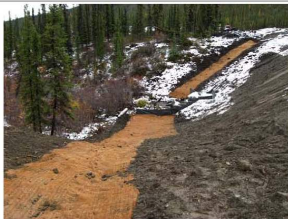
Image 1297. View of the outlet channel from the west bank, fully isolated with fencing and erosion control matting stapled in place.
