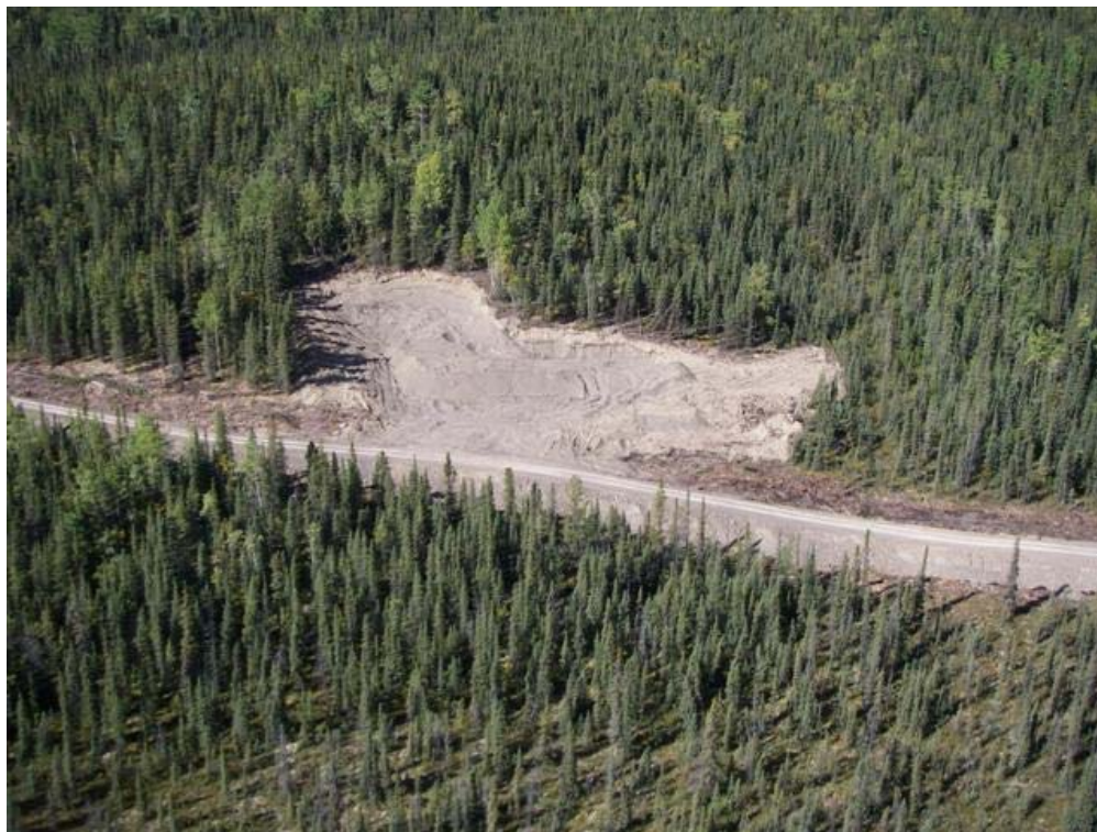
Picture 2-3 Borrow pit near km 4+00.
