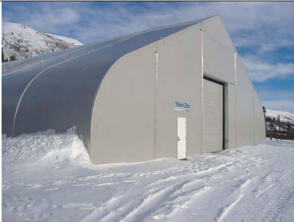
10/13/07 Completed WDS Structure (facing E)
