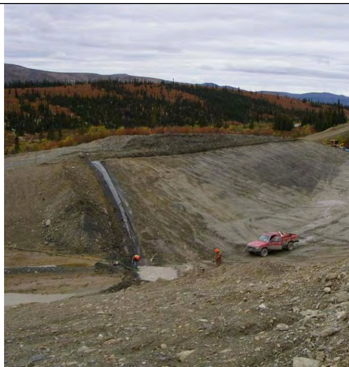
09/07/07 Exposing the Phase I liner in preparation for welding (facing W)
