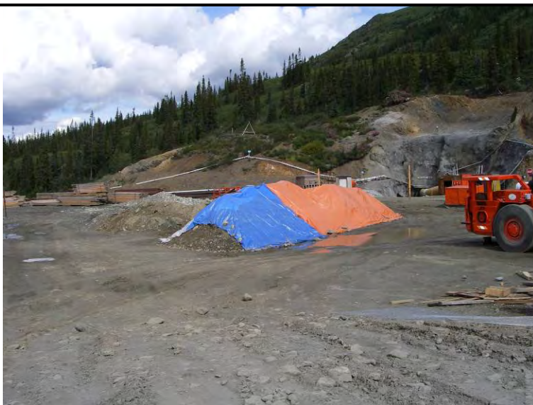
07/28/07 The piled and tarped soil after removal; facing N
