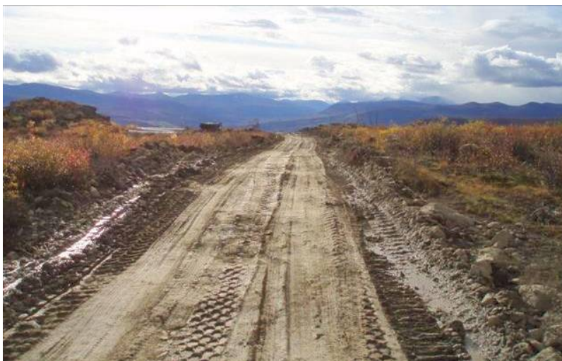
Picture 2-2 Access Road near km 18, heading south towards the mine site.
