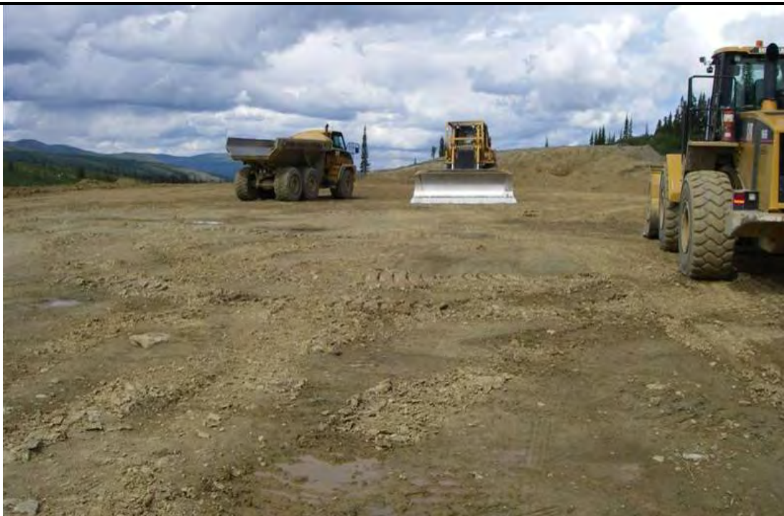
28/07/07 Progress of camp pad; facing N
