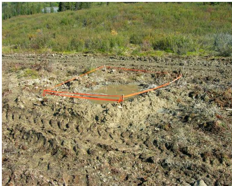
08/28/07 Sump for drill cuttings
