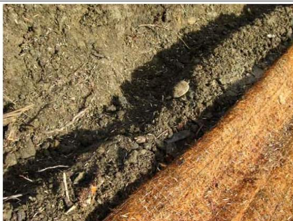
Image 1295. Seeding on top of erosion control matting installed on the northeast bank of the culvert outlet. Note trench for securing edge of matting.
