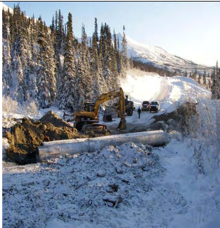
Photo 2 - 12/04/07 - Placing culverts looking SE
