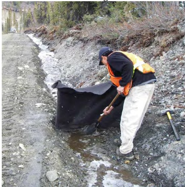
Geo-tech fence installation
