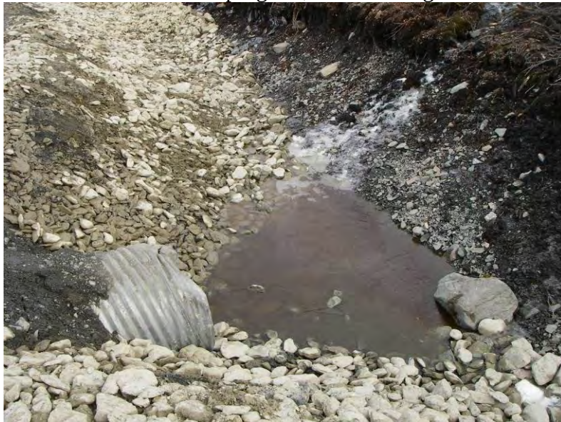
Completed north side, looking northwest
