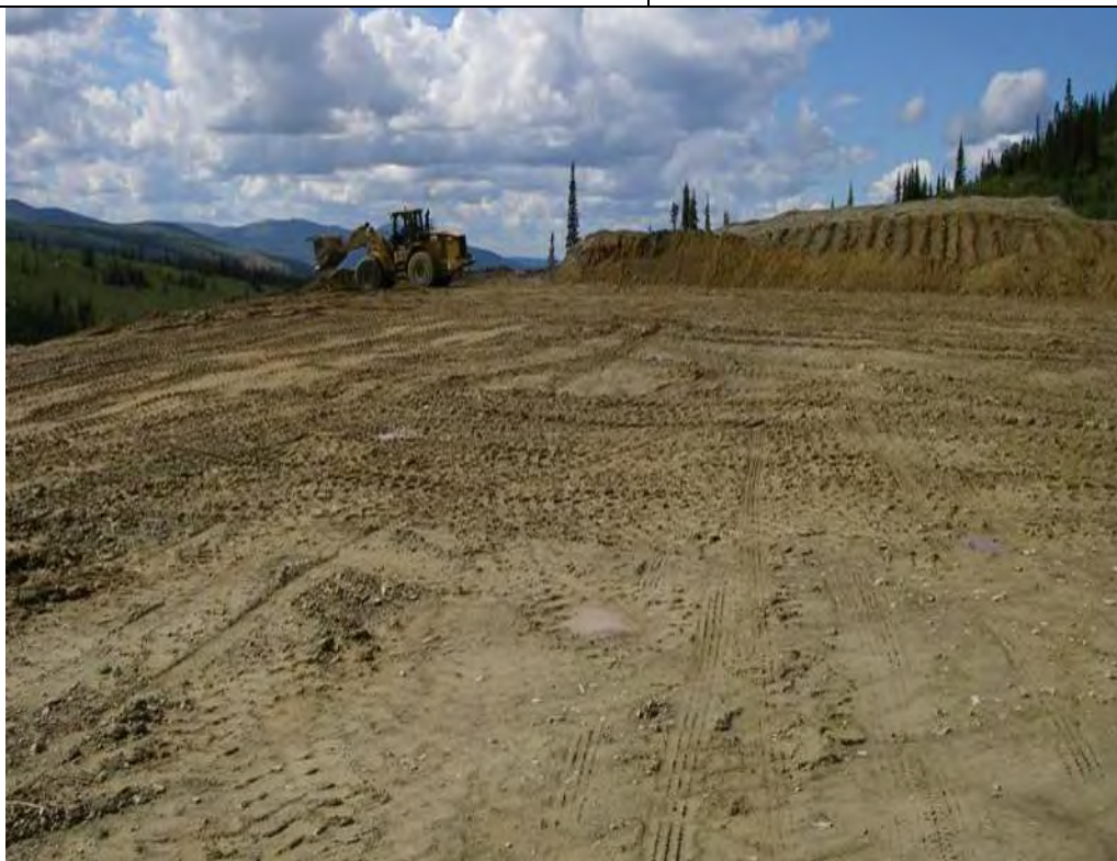
25/07/07 Progress of camp pad; facing N
