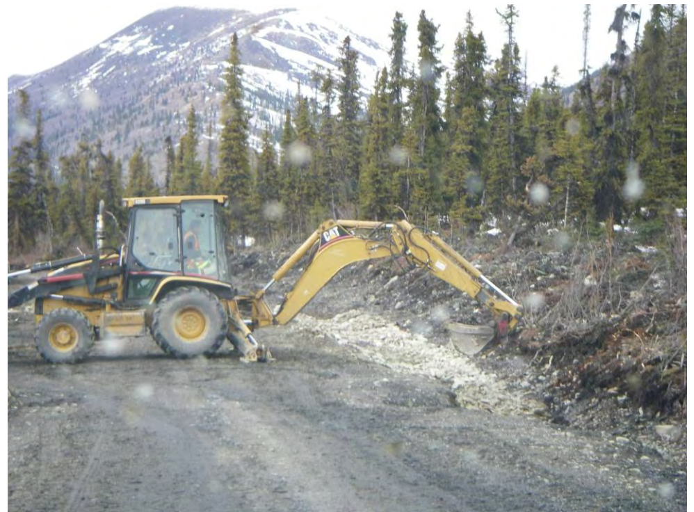
Rip-rap installation (looking North-West)
