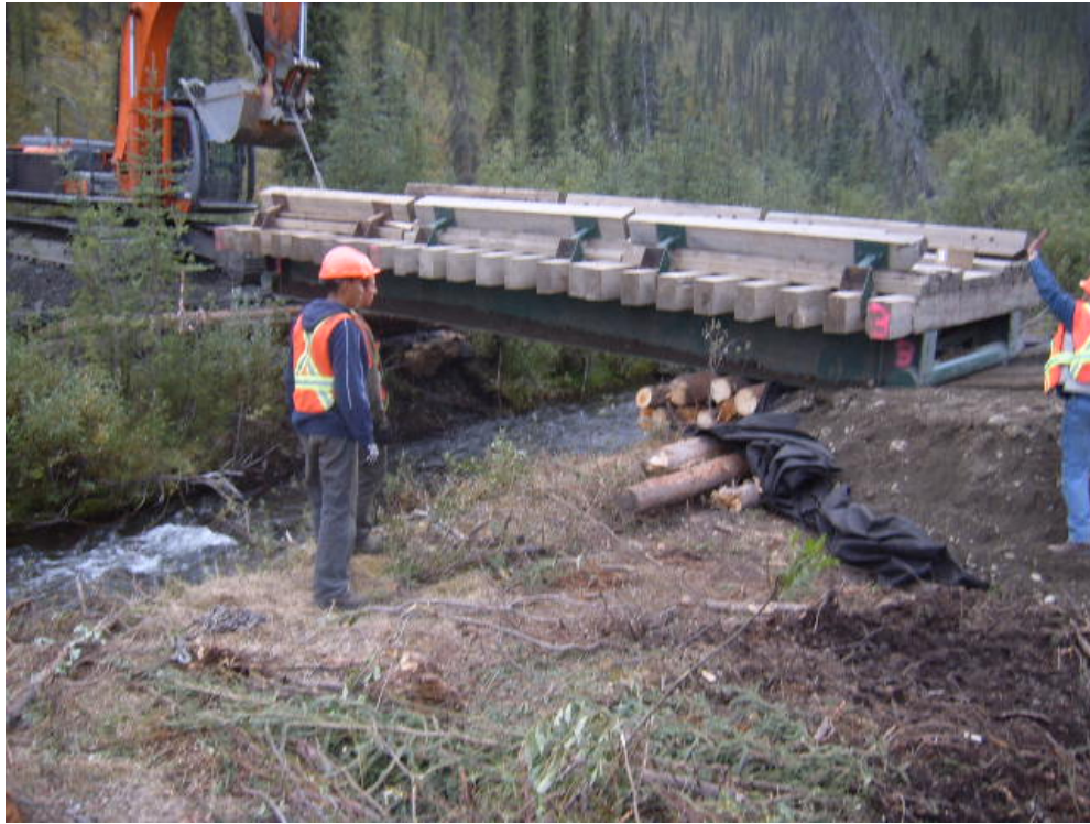
Picture 2-10 Installation of a 30 ft temporary bridge on timber abutments at Bunker Creek.
