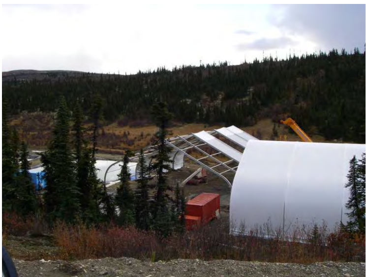
09/17/07 80' x 90' assembly (facing W)
