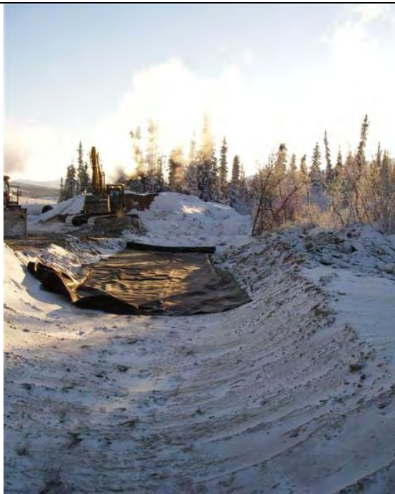
Photo 1 - 12/04/07 – Semi-circular excavation Go Creek; looking south
