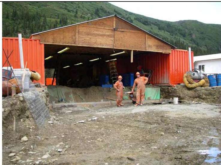
07/26/07 Area of removed soil (behind the miners, in the maintenance shop); facing W
