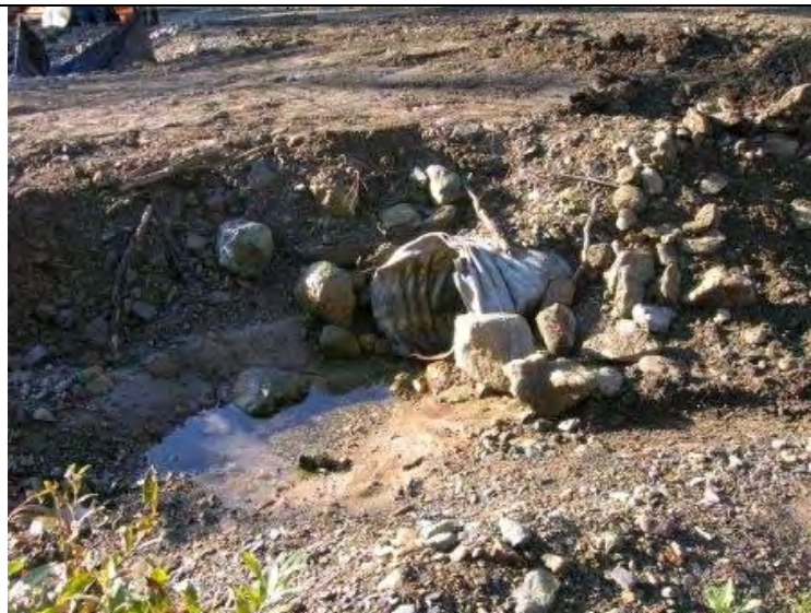
08/27/07 Culvert inlet at Campbell Creek
