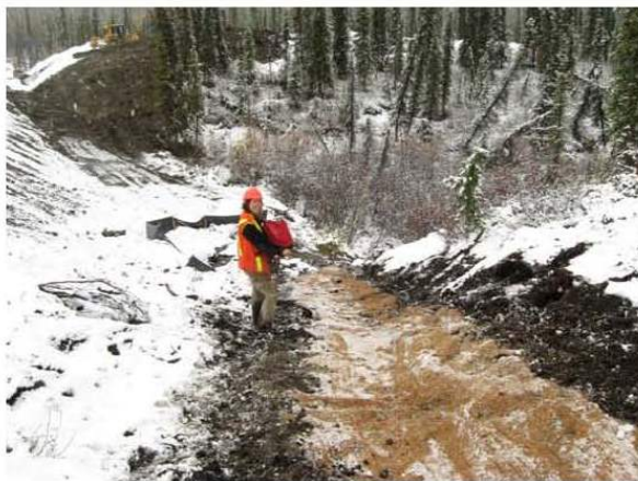
Image 1266. Seeding on top of erosion control matting installed on the northeast bank of the culvert outlet.
