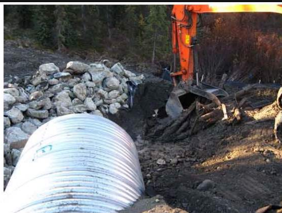
Image 1191. Excavation of inlet channel. Visible logs are from earlier corduroy bypass road.
