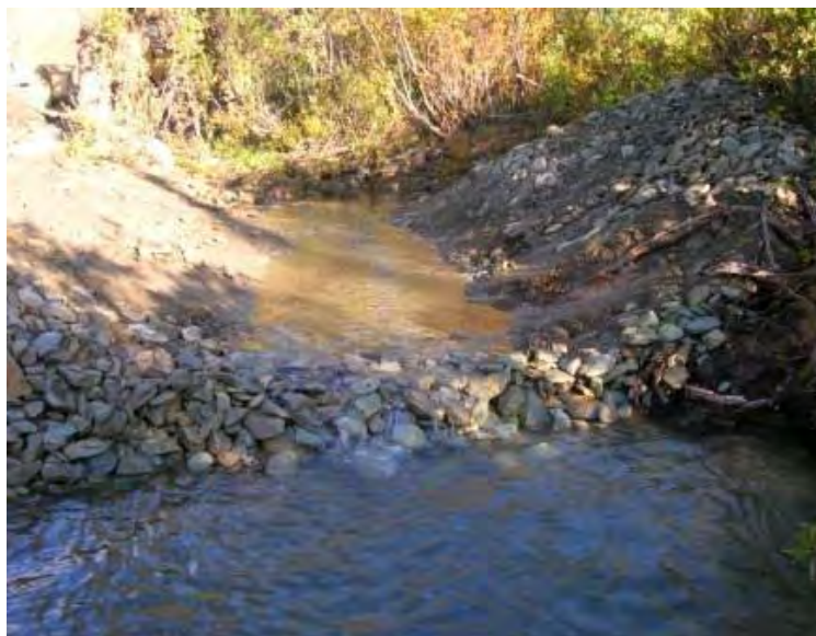
08/27/07 Cobble installed at Campbell Creek; facing N
