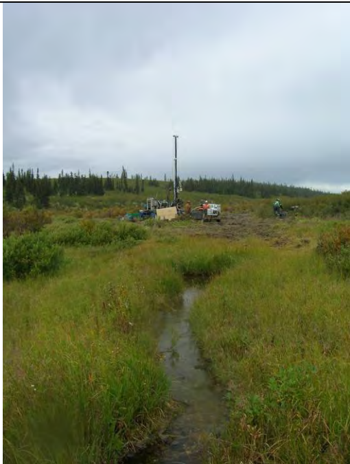
08/21/07 Site B facing West
