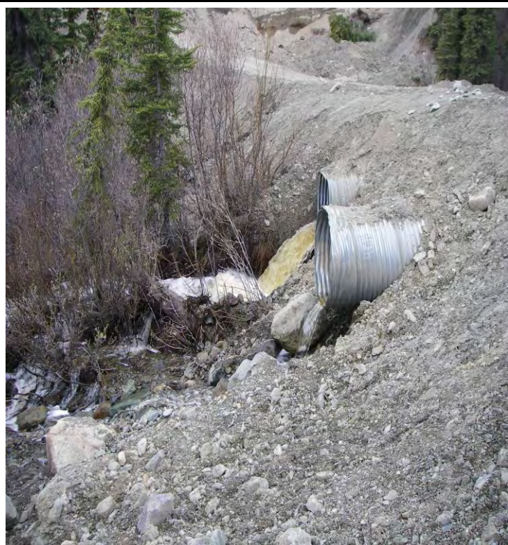
05/26/07 Culvert flow from Campbell Creek; facing N
