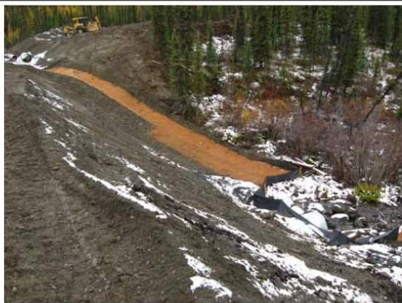
Image 1298. View of the outlet channel from the east bank, fully isolated with fencing and erosion control matting stapled in place on the west bank.
