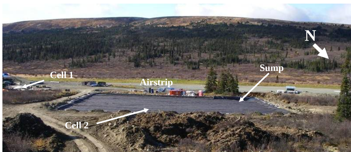
Picture 2-16 Completed land treatment facility cell 2 prior to acceptance of soil (September 18th, 2007)
