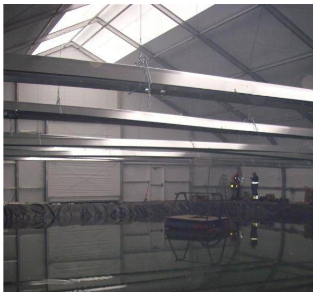
Picture 2-14 Radiant heaters within the Sprung Structure over the WDS sump (September 2007)
