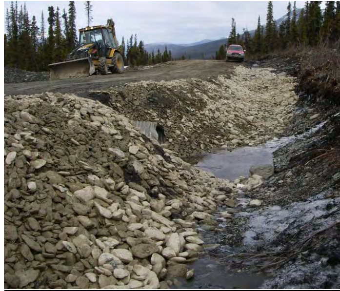
Completed north side; view looking west
