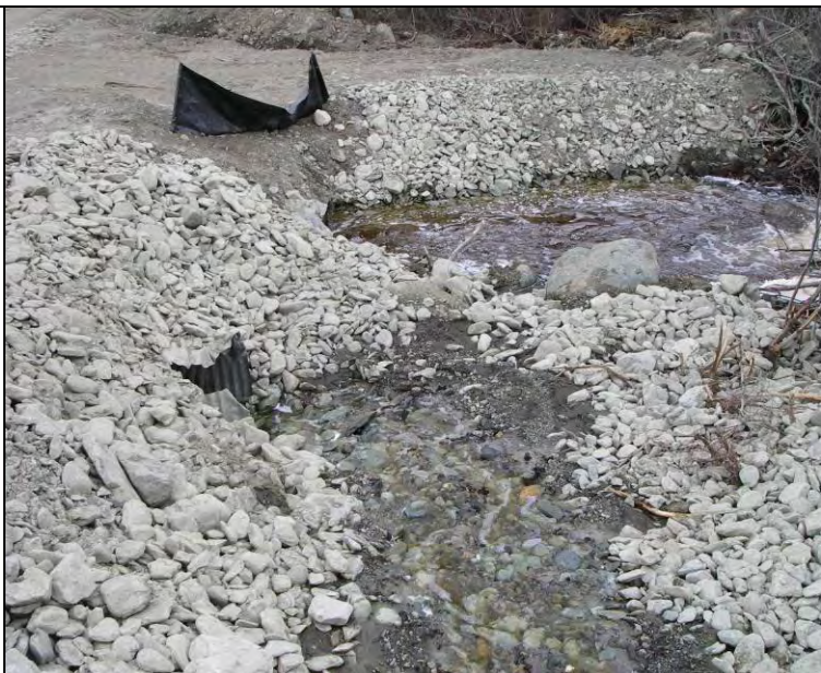
05/26/07 Ditch flow into Campbell Creek; facing N
