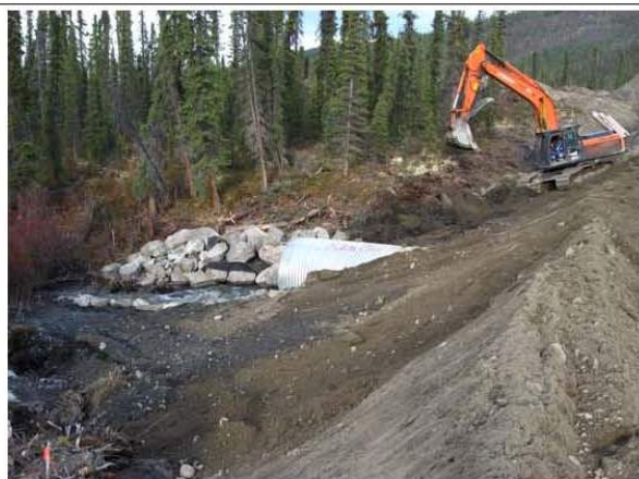
Image 1227. Final riprapped outlet channel following release. Excavator is cleaning up drainage ditch.
