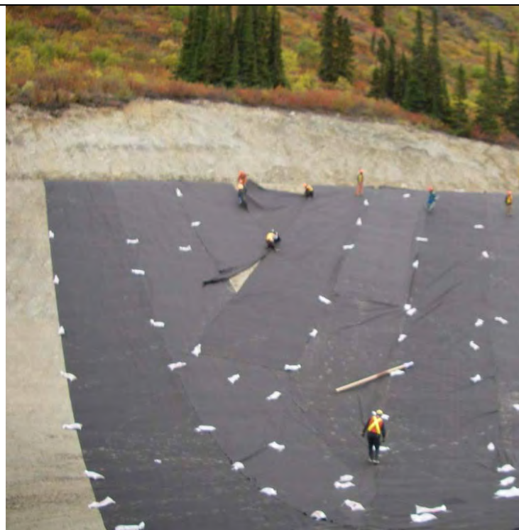
09/08/07 Laying down geotextile fabric (facing N)
