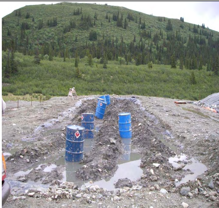
Photo 1 07/07/07 Water containment in drums: facing east
