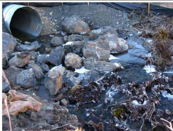
Image 1376. View of the culvert outlet channel. Note abundant ice as hard overnight frosts are becoming common.
