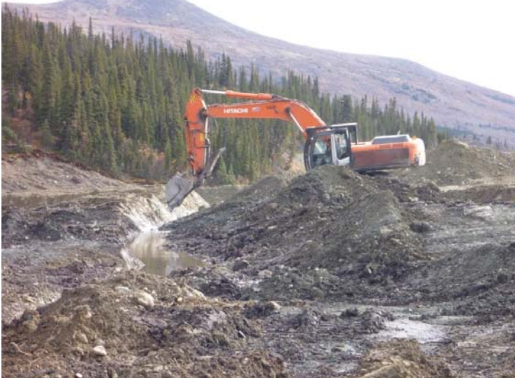
Photo 7 (11/09/19) Showing construction of diversion ditch within the New WRP area.
