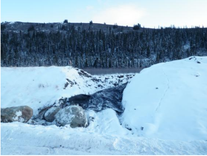
Photo 1 (11/10/21) Lining the original diversion ditch with geotach and riprap.
