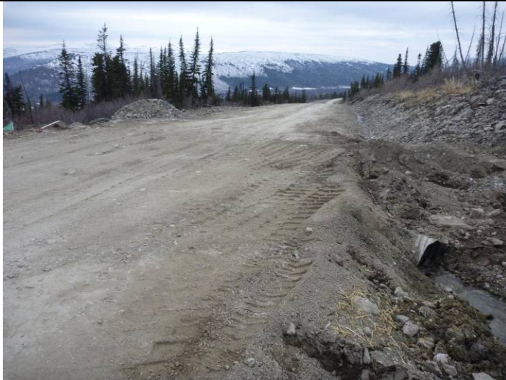
Photo 9 (11/05/18) Culvert repair at KM 19.5 completed
