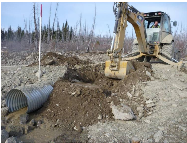
Photo 7 (11/05/18) Initiation of excavation and backfill to support culvert repair at KM 19.5
