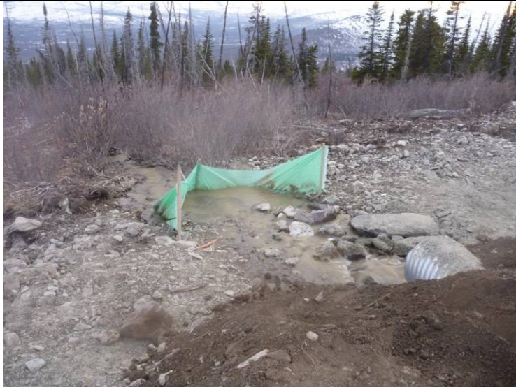
Photo 1 (11/05/18) Diversion ditch at KM 19.5 before erosion control measures installed – straw placed along space below silt fence to filter sediment
