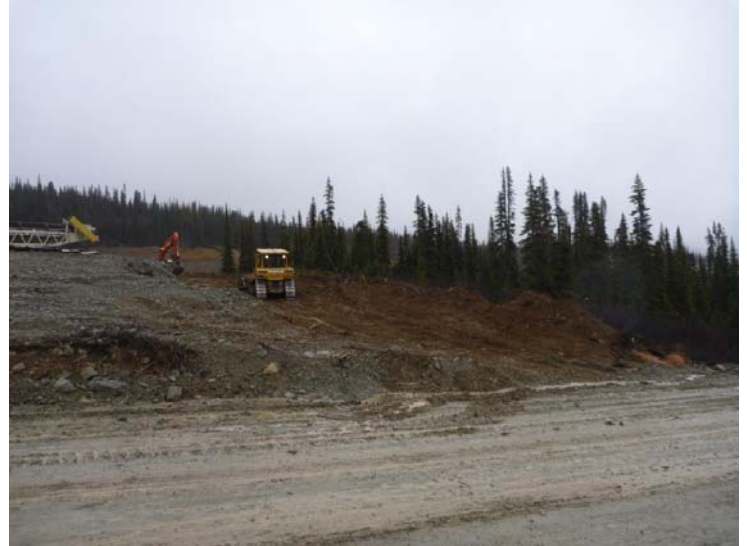
Photo 8 (11/09/22) Stripping of organics at future borrow site (for ultimate dam lift) to make room for WRP backfill.
