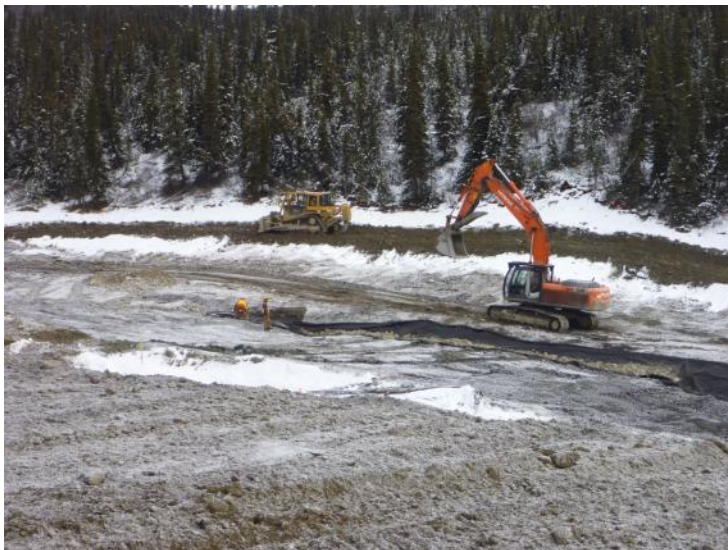
Photo 3 (11/10/15) D8 installing berm around the perimeter of pad.
