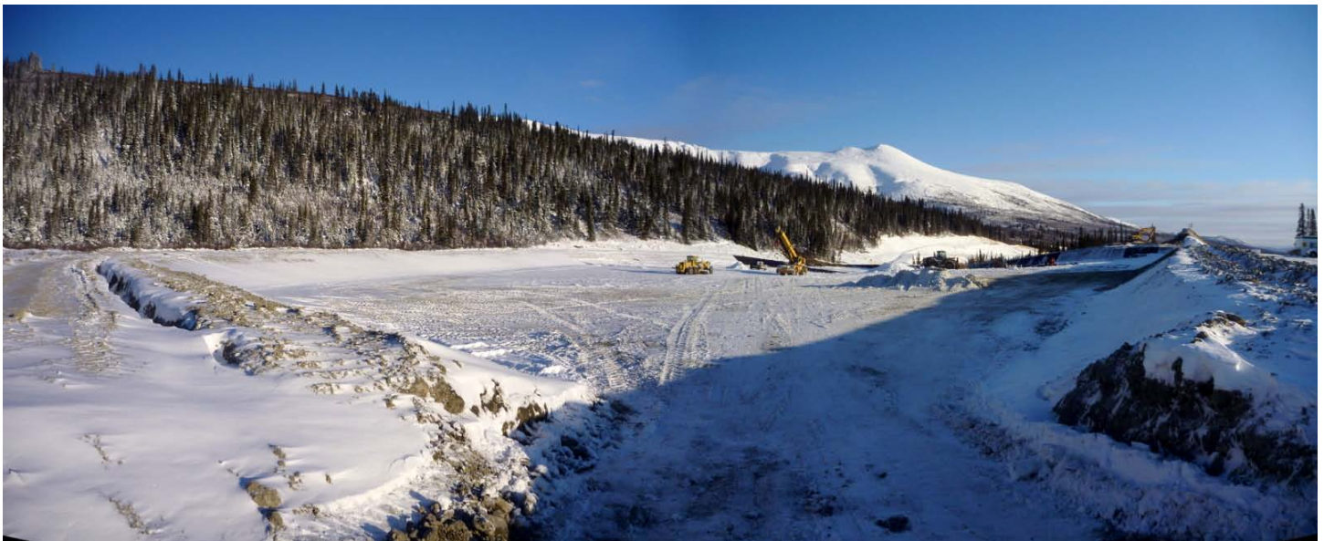
Photo 11 (11/11/03): .Looking east – Working continuing to place liners within the pad. Continuing with removal of snow within the pad.
