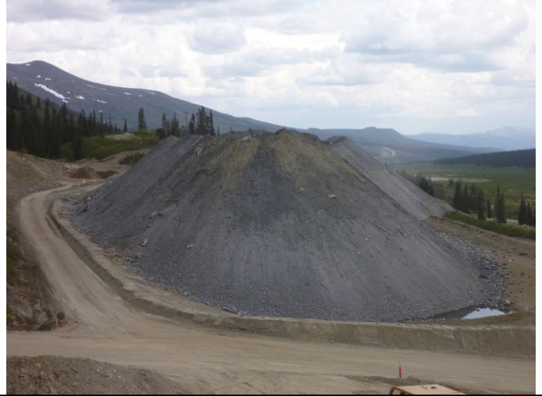
Photo 2 11/06/17 Berm is to allow proper drainage.
