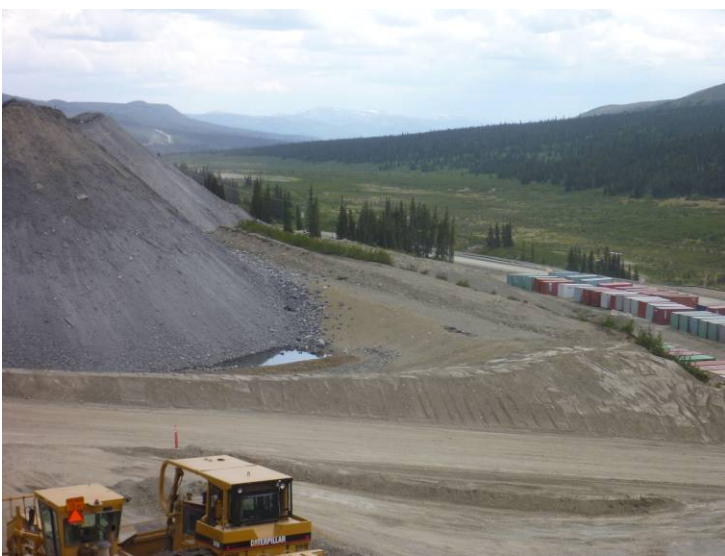
Photo 3 11/06/17 WRP with completed west wall.
