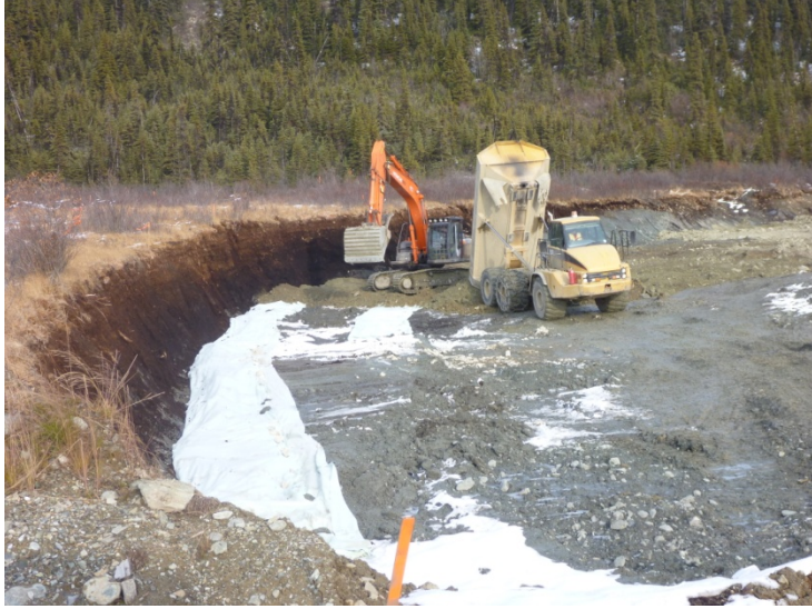
Photo 1 (11/10/02) French Drain insalation started at north end of pad.
