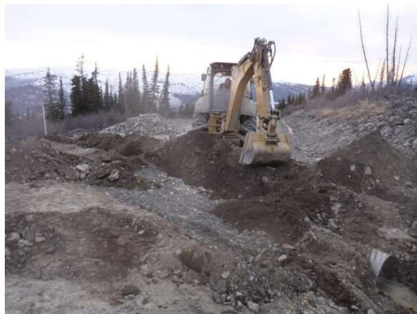
Picture 7-4: Repair of undermined culvert at KM 21
