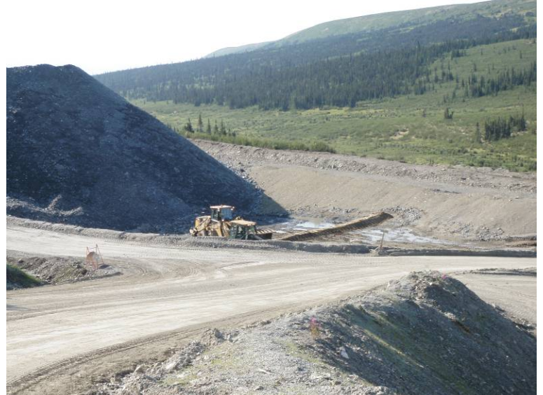
Photo 4 10/07/28 Picture taken of WRP prior to work (i.e., No west wall).
