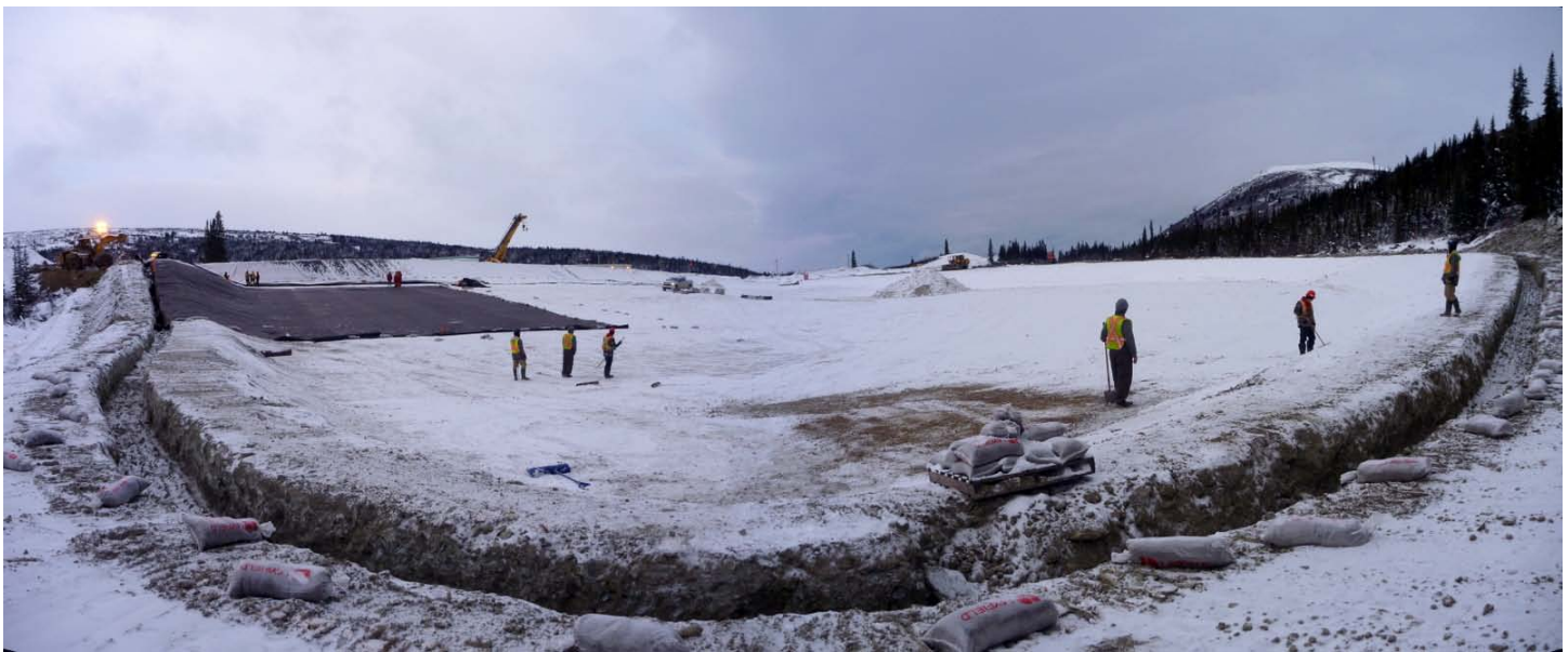
Photo 7 (11/11/01): .Looking west – Mid morning 3 rd liner panel installed along the southwest wall; snow removal within the pad and trenching the anchor trench along the perimeter of the pad.
