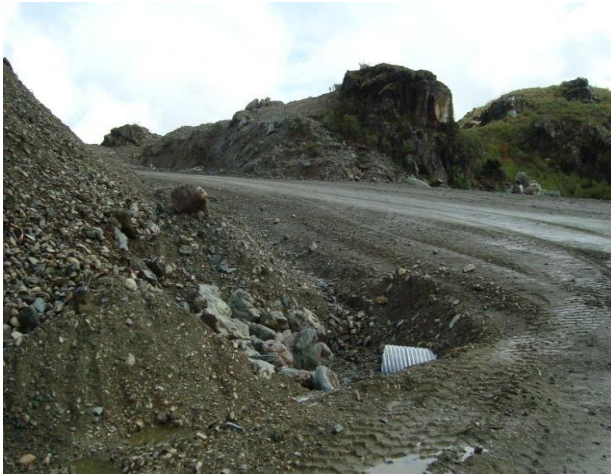
Picture 7-3: Installation of a culvert at KM 19 to divert heavy flow
