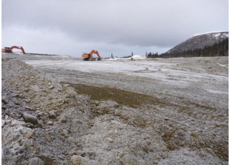
Photo 2 (11/10/15) Pad being leveled out in preparation for liner.
