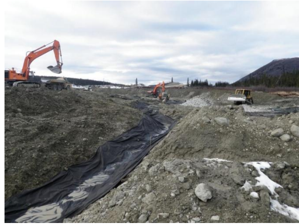
Picture 8-2: French drains installed under waste rock pad to control water flow and stabilize surrounding soil.
