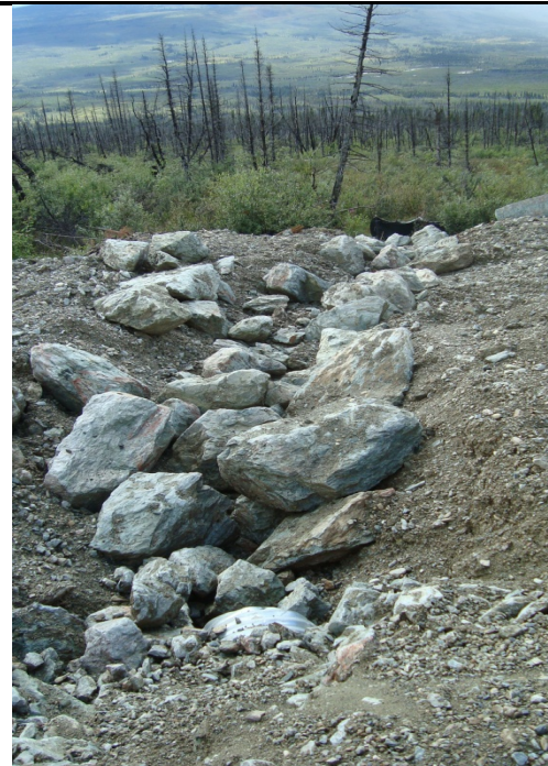
Photo 12 (August 17, 2011): KM 19 Looking west - down slope rip rap and silt fencing installed after the culvert.
