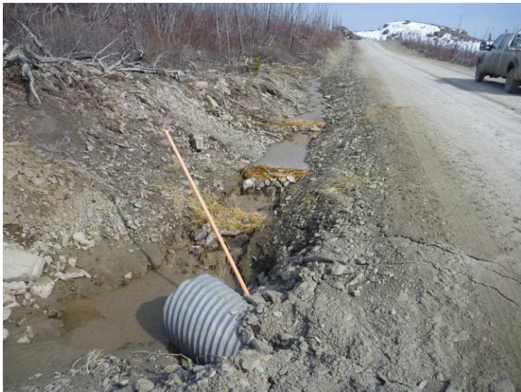
Photo 3 (11/05/18) Rock blocks with straw installed upstream of culvert inlet at KM 19.5
