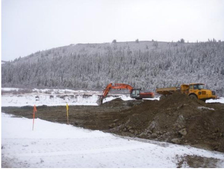
Photo 1 (11/09/26) Excavating overburden material (south)
