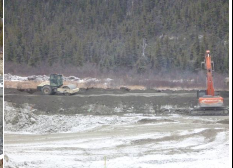
Photo 2 (11/10/04) ) The French Drain is now located under this thick layer of overburnden along the west end of the pad.
