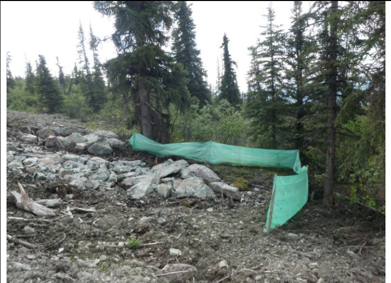
Photo 2 (11/06/17) After (silt fence has been repaired)
