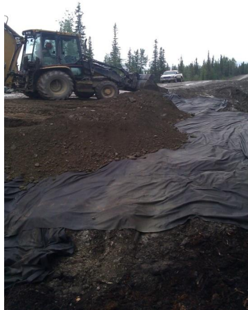
Picture 7-2: Installation of geotextile and re-grading at KM 4.5 where permafrost was an issue
