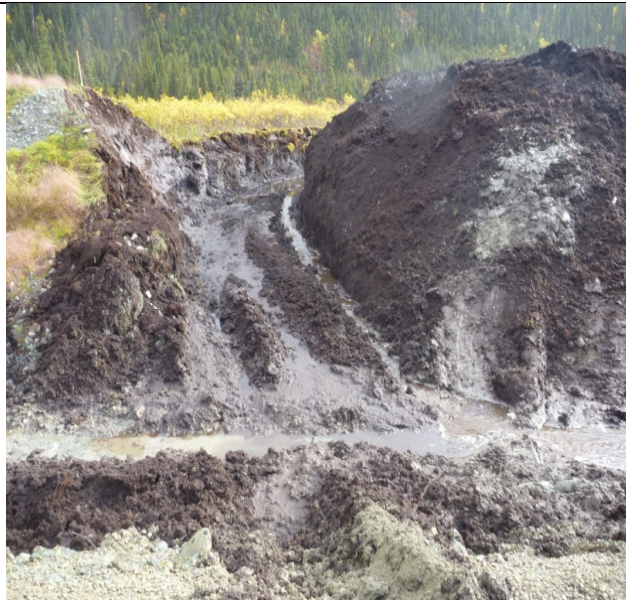
Photo 1 (11/09/04) Result of diversion ditch excavation and removal of organics.
