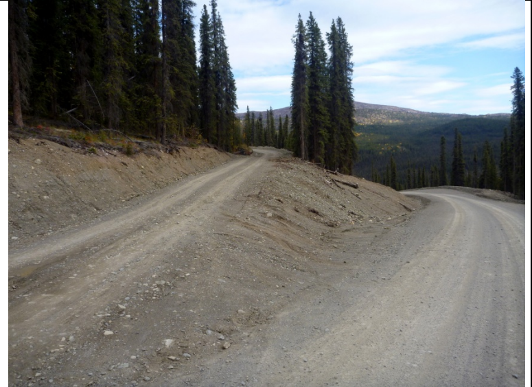
Photo 10 (September 13, 2011): KM 11.5 Looking south - packed cut and fill slope of the borrow source access road
