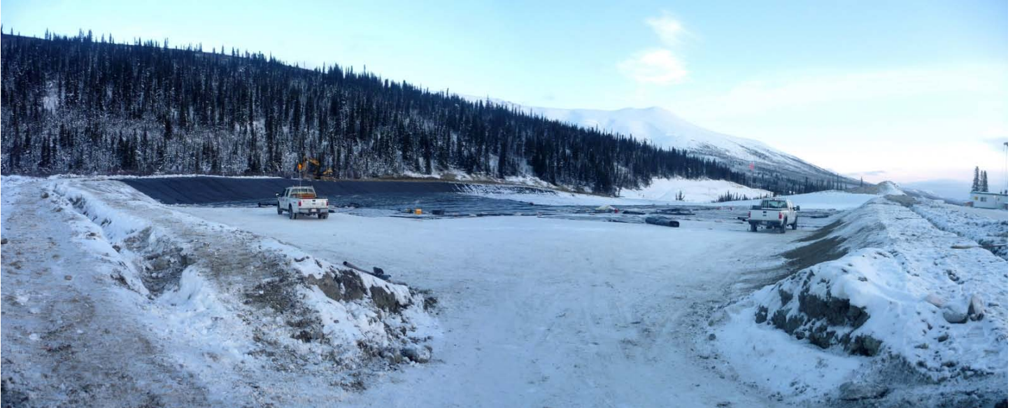
Photo 5 (11/11/10): Looking east (pm) – Day 13 - Laying protective geomembrane cloths within the pad.
