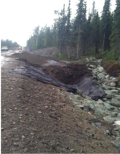
Picture 7-1: Re-contouring/widening of road and installation of geotextile and rocks to stabilize slopes and reduce high energy flows
