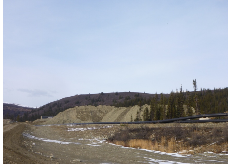
Photo 4 (11/10/02) The overburden stock pile has increased in size as construction is ongoing. (stock piled for ultimate dam lift)
