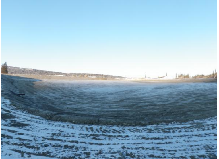
Photo 2 (11/10/21) Pad has been back filled and leveled in preparation for the geotech and liner.
