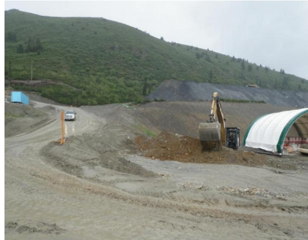
Picture 7-6: Final stages of road improvement measures at KM 27 + 200
