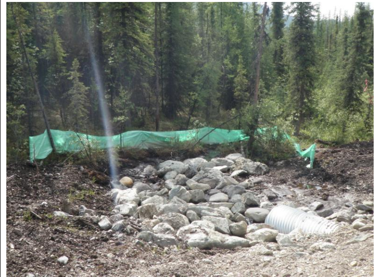
Photo 4 (11/06/17) Sediment Control at a large drainage point along the access road.
