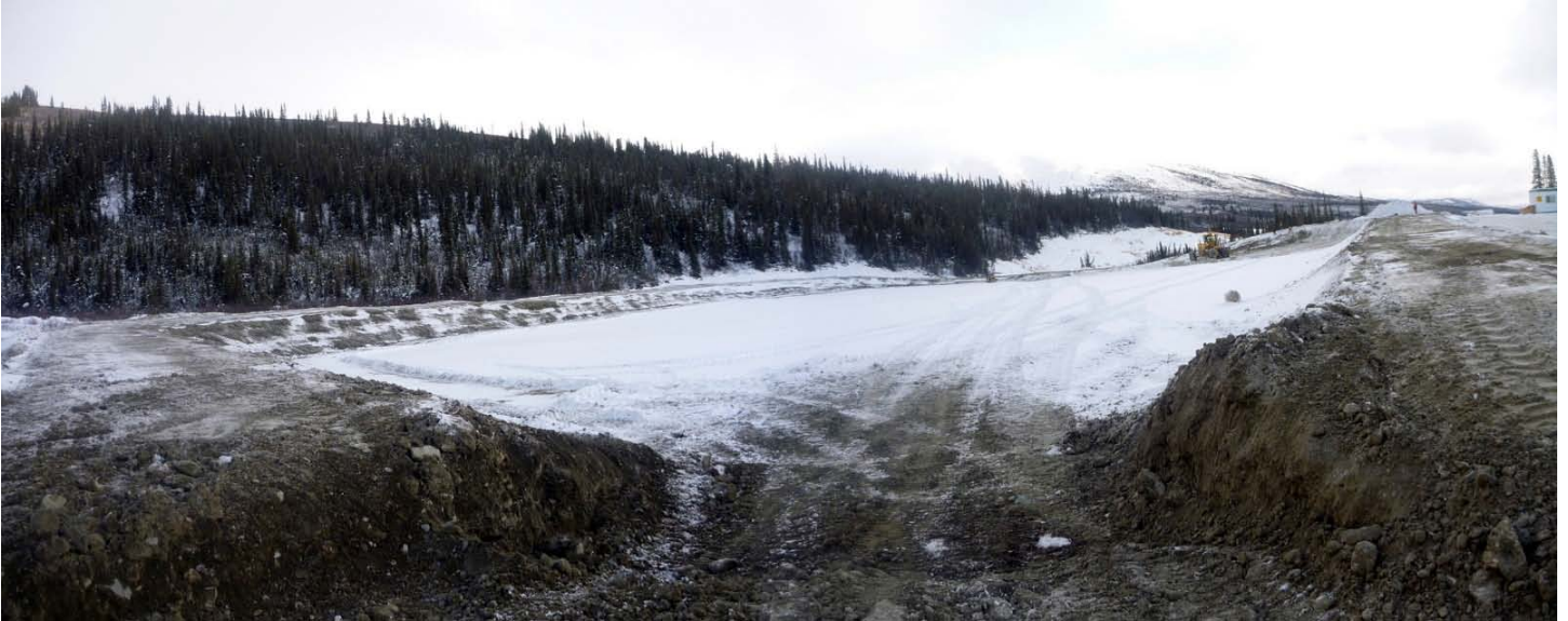
Photo 3 (11/10/29): Looking east – removing loose rocks along southeast berm.
