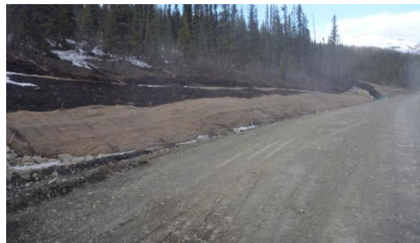
Picture 8-4: Installation of coconut matting and seeding along side of road where permafrost was evident
