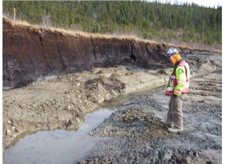
Photo 6 (11/09/19) Ditching was required to divert water while excavation was carried out.
