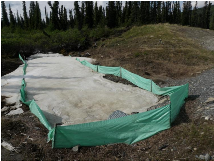
Photo 3 (11/06/17) Sediment control at Pitch Creek.
