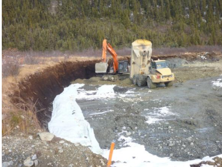
Photo 1 (11/10/02) French Drain instalation has begun at the West end of the pad. Currently being covered with overburden materiel.
