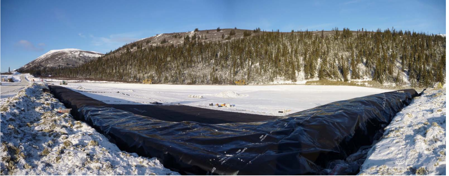
Photo 5 (11/10/31): Looking north – installing A-panel liner along the southeast wall.
