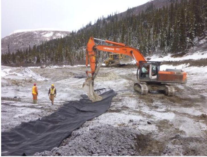
Photo 1 (11/10/15) French drain and finger drains being installed to divert water.
