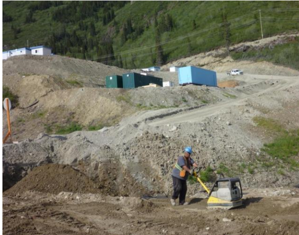
Picture 7-5: Initial stages of road improvement measures at KM 27 + 200
