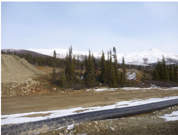
Photo 3 (11/10/02) Material has been stripped to make room for overburden stockpile at south end of ACL lay down.
