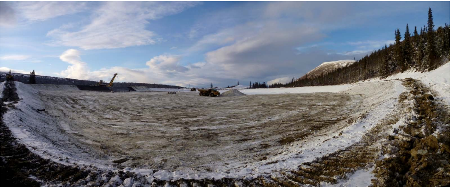
Photo 7 (11/10/30): .Looking west – installing geo-membrane cloth and G-panel liner along the southwest wall; snow removal within the pad and trenching the anchor trench along the perimeter of the pad.
