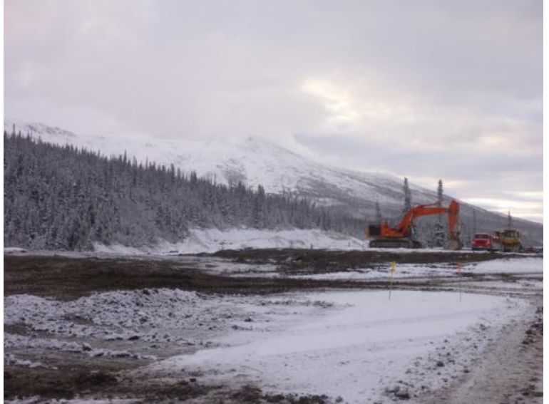
Photo 2 (11/09/26) Excavating overburden material (north)
