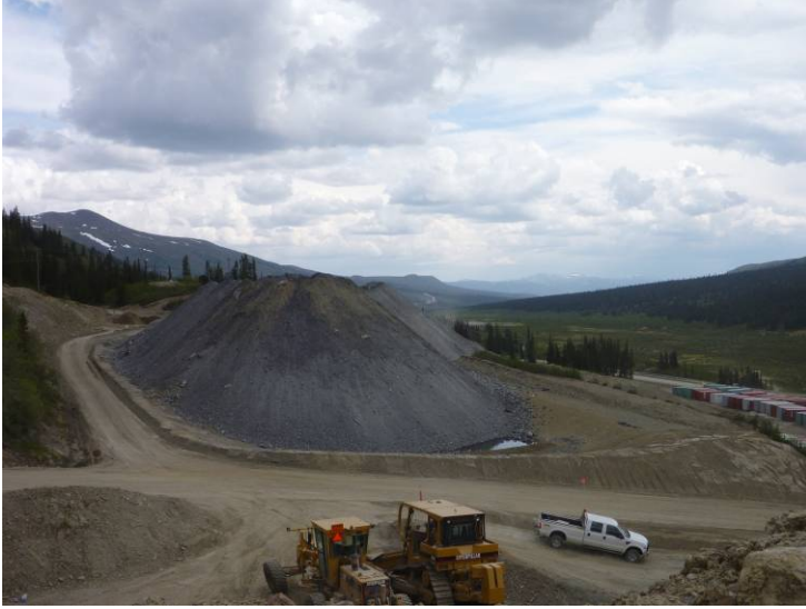
Photo 1 11/06/17 WRP now has a west wall and larger surrounding berm.
