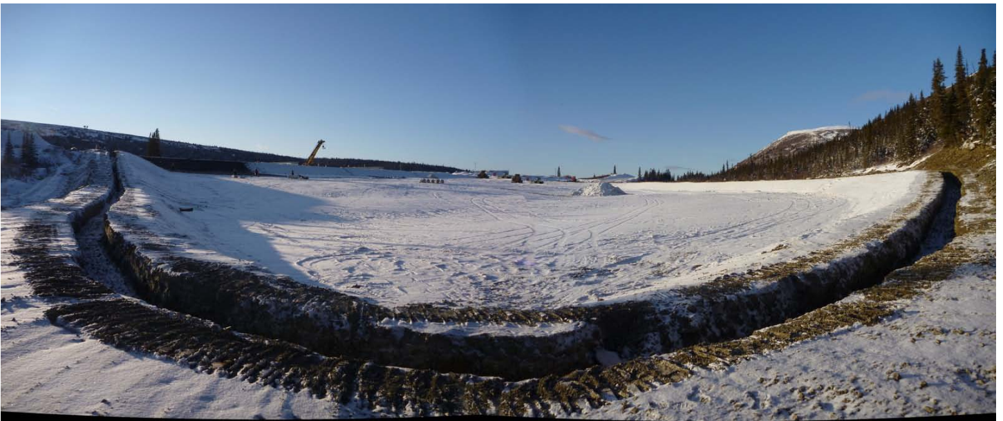
Photo 6 (11/10/31): Looking west – installing geo-membrane cloth and A-panel liner along the southwest wall; completed trenching of anchor trench along the southeast and northeast perimeter of the pad.
