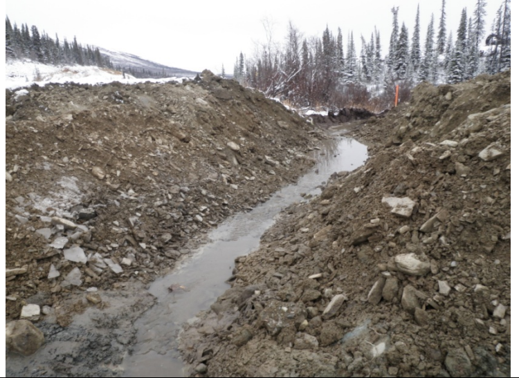
Photo 4 (11/10/08) old pipe was dug out water not plugged anymore.
