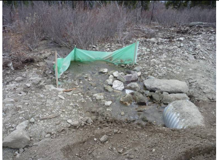
Photo 2 (11/05/19) Diversion ditch at KM 19.5 after erosion control measures
