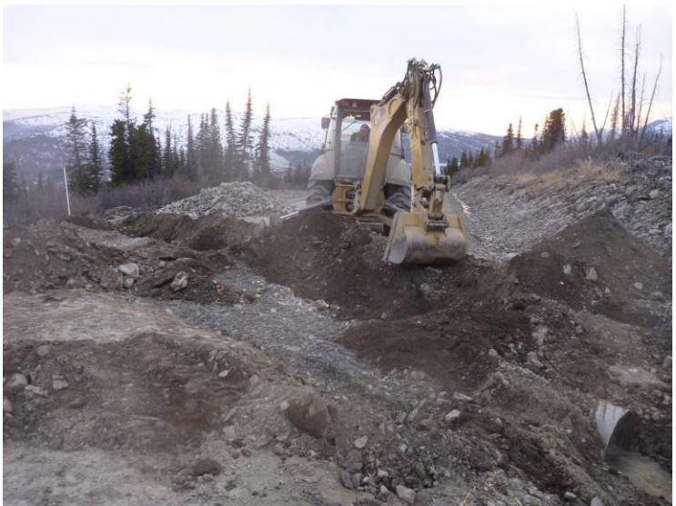
Photo 8 (11/05/18) Excavation and backfill to support culvert repair at KM 19.5
