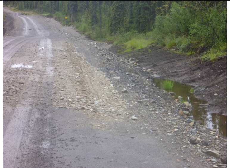
KM6.2 Repairs to the road
