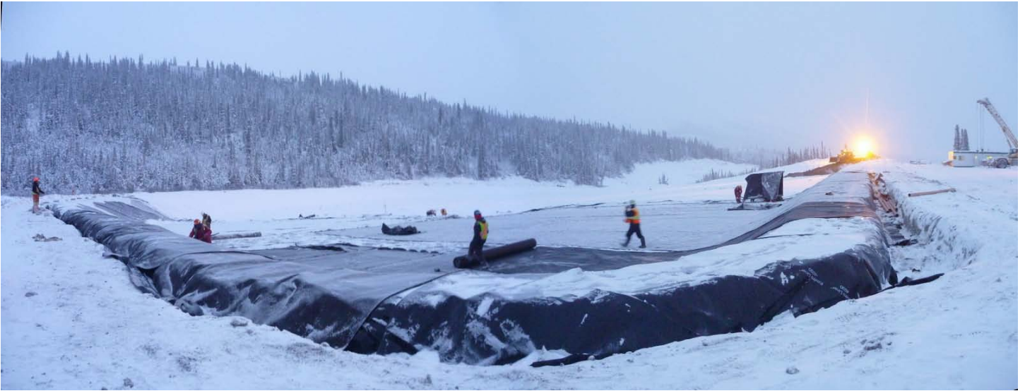
Photo 7 (11/11/12): Looking east (pm) – Day 15 – Layfield personnel seaming liner panels together over the protective geomembrane cloths. Second protective geomembrane cloths rolled over the final liner panel.
