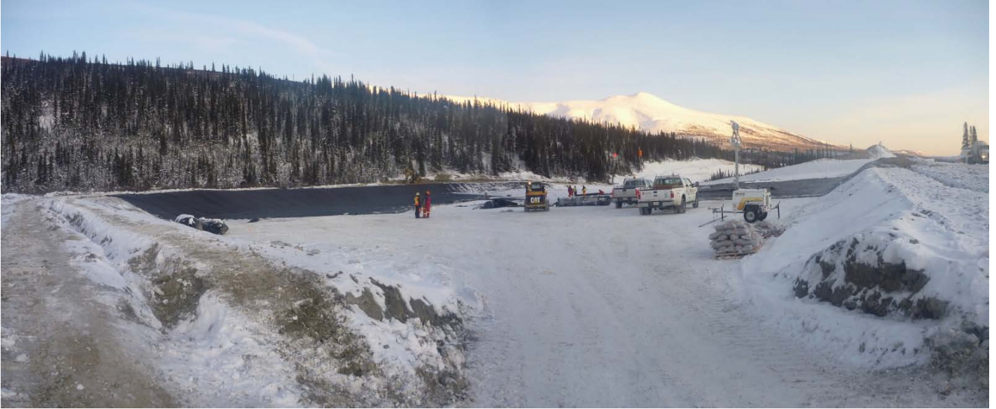
Photo 5 (11/11/09): Looking east – Laying more geomembrane along the northeast berm.
