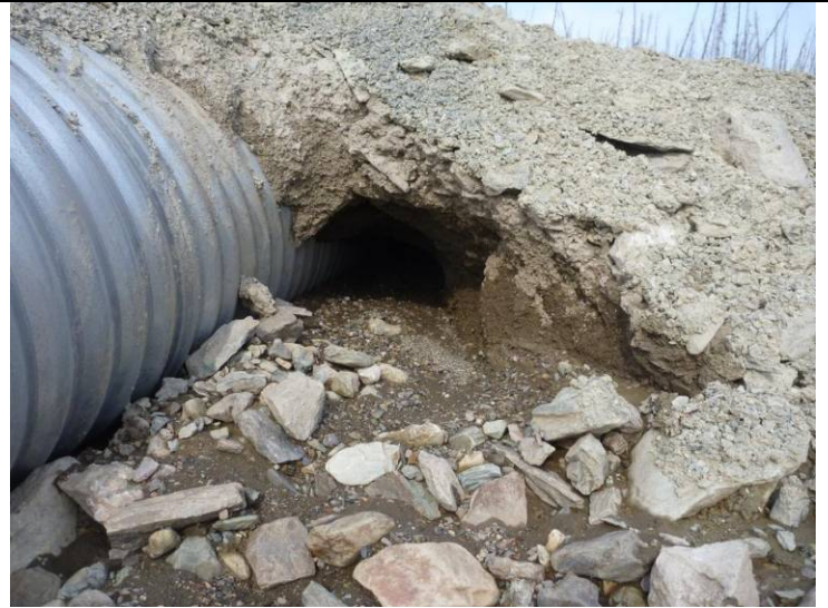
Photo 6 (11/05/18) Downstream side of culvert at KM 19.5 showing tunnel
