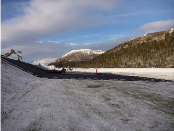
Photo 5 (11/10/30): Looking north – laying 2 nd LP16 geo-membrane cloth over the G-panel.
