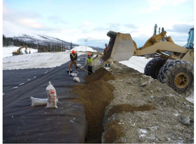
Photo 6 (11/10/30): .Looking southeast – G-panel completed. Anchor trench backfilled with materials.
