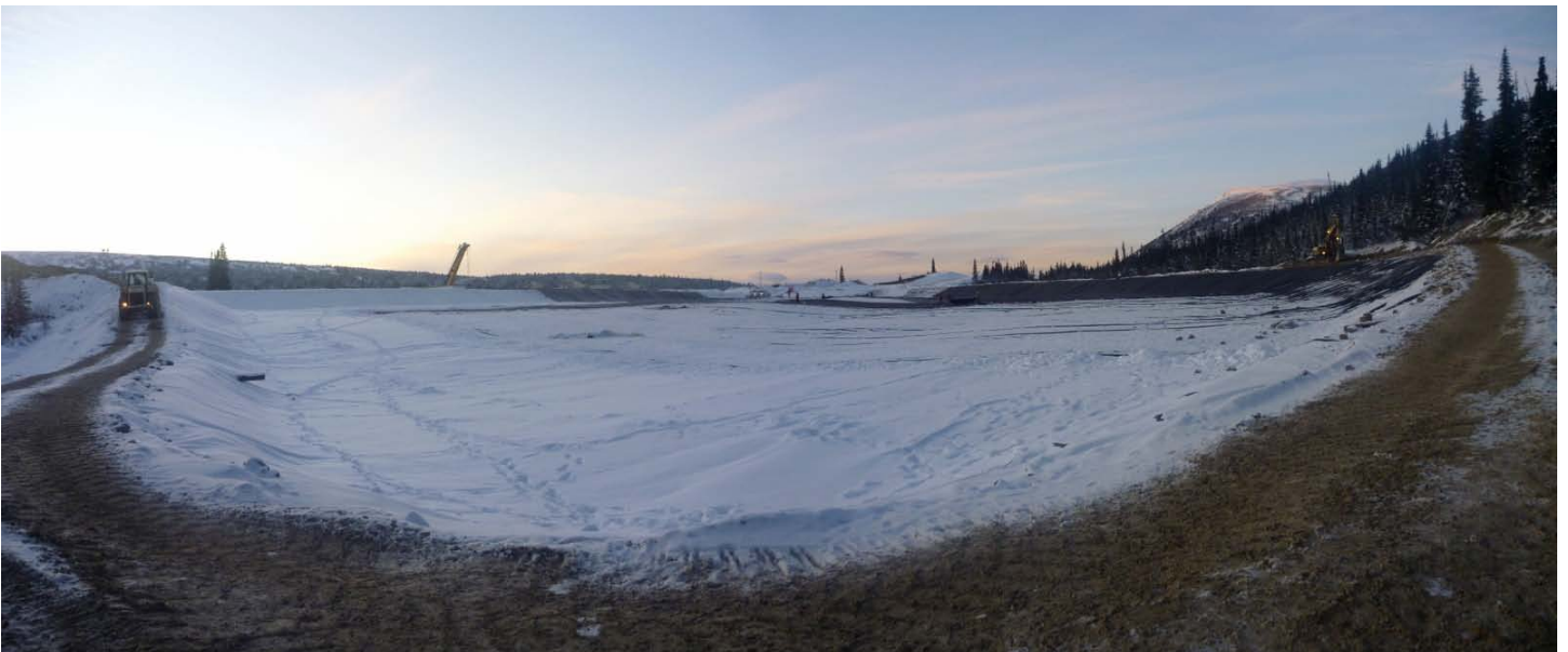
Photo 7 (11/11/09): Looking west – Laying more panels and geomembrane cloths; anchoring geomembrane cloths and liner within the anchor trench along the northeast berm.
