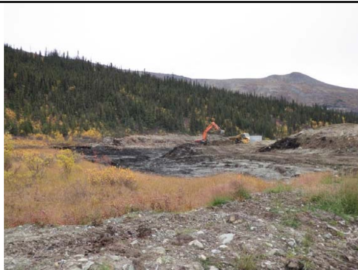
Photo 4 (11/09/05) Initial stages of excavation for the preparation of the New WRP.
