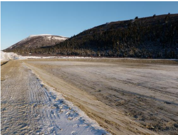
Photo 3 (11/10/21) The berm has been completed around the perimeter of the pad.
