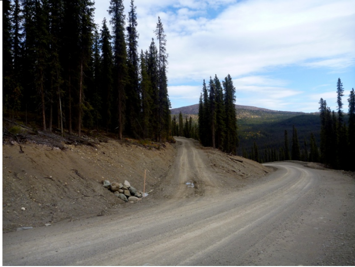
Photo 9 (September 13, 2011): KM 11.5 Looking south - extension to the culvert and rip rap placed before the culvert.
