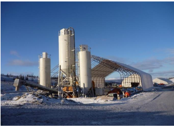
Picture 2-2: Wet shotcrete plant under construction
