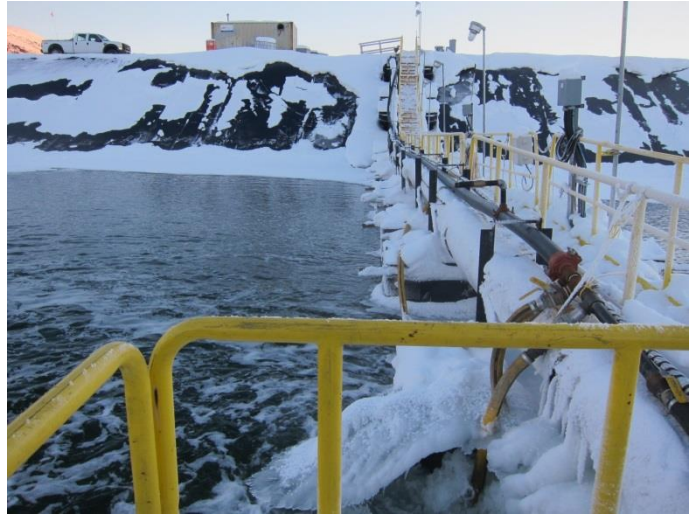
Photo 6: East side of TSF view from barge pumps.
