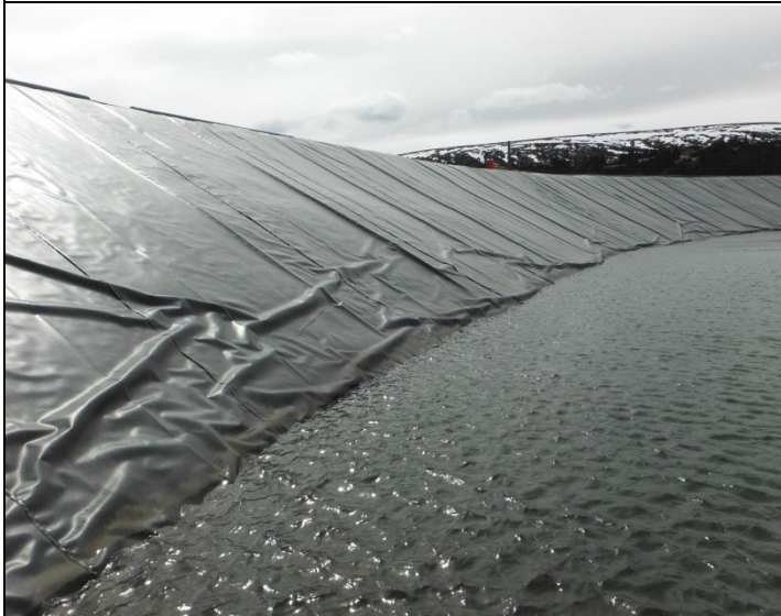
Photo 7: looking at south west corner of TSF.
