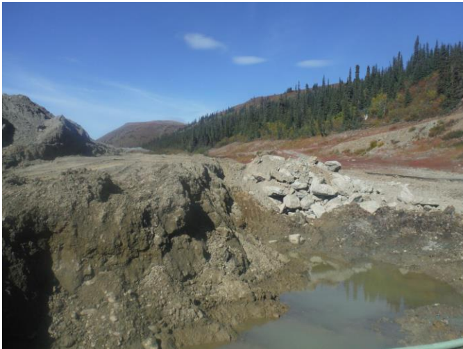
Photo 7: Current construction/rehabilitation of Ditch A on the North end of TSF.
