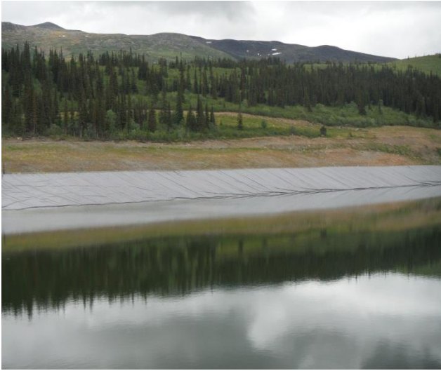
Photo 5: looking at the north wall.
