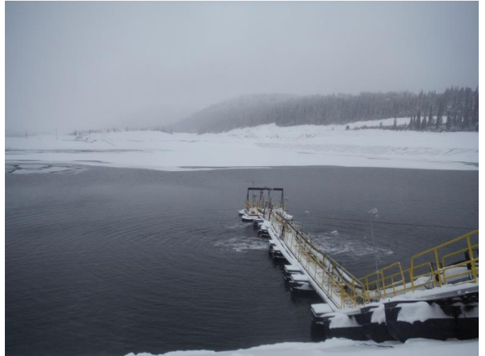
Photo 6: Closer view of barge pump system.
