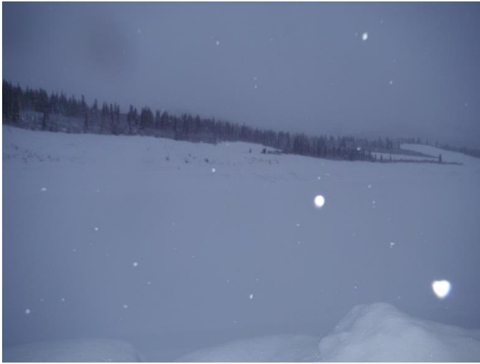
Photo 5: View of east slope from the north side of the TSF.
