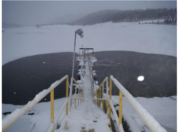
Photo 2: Looking over the barge station towards the north side.
