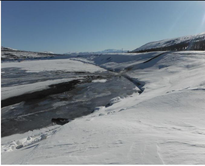
Photo 1: Looking at mill tailings discharge line with pump reclaim water pump house overflow line in foreground
