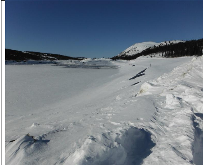
Photo 5: looking at East wall from South East corner of TSF
