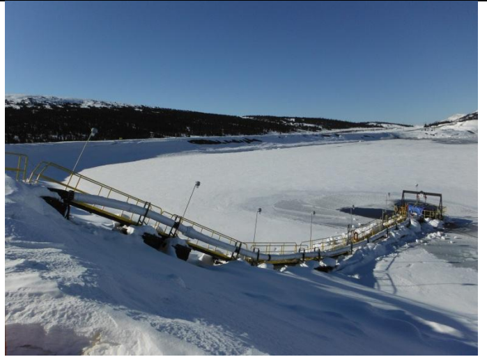
Photo 6: looking at west wall from South wall of TSF
