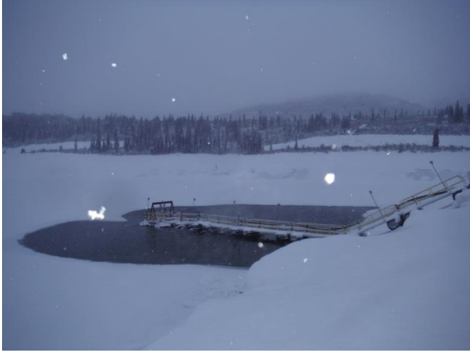
Photo 1: Looking at south east corner side of TSF and barge station.
