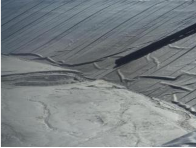
Photo 1: Looking at original discharge location on east side of TSF.
