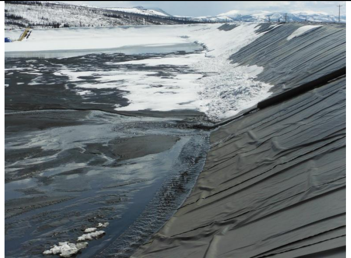
Photo 2: Looking at south wall from North West corner of TSF
