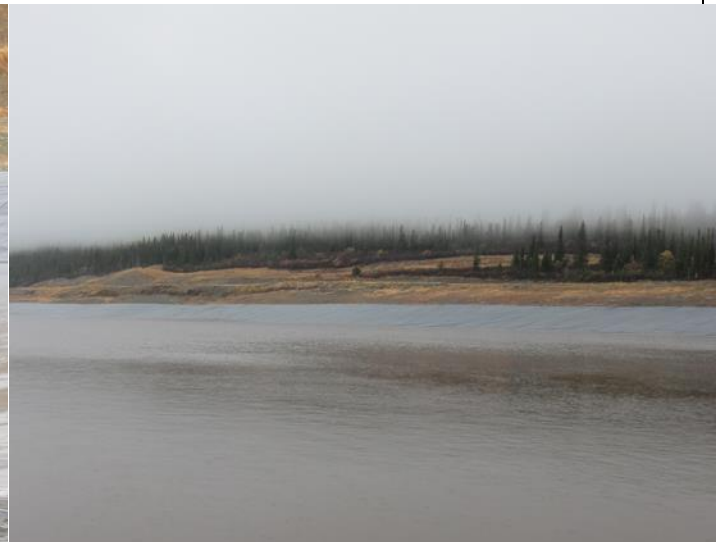
Photo 4: View of North wall of TFS.
