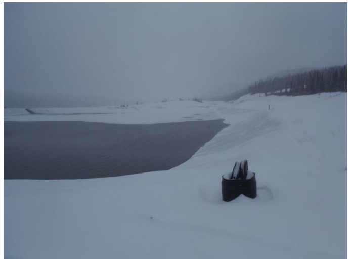
Photo 4: View of North wall of TSF.
