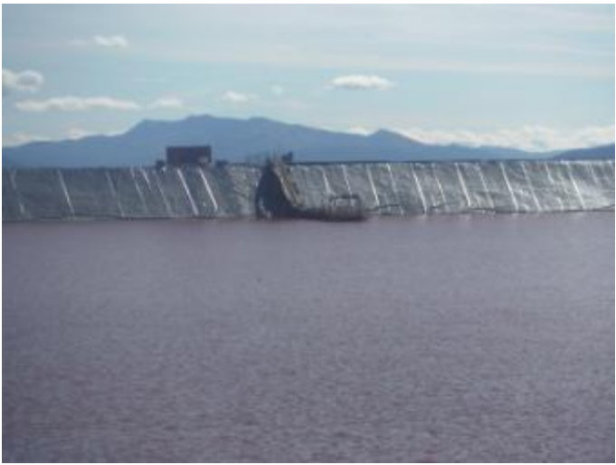
Photo 3: View of Barge for North-east side of TSF.
