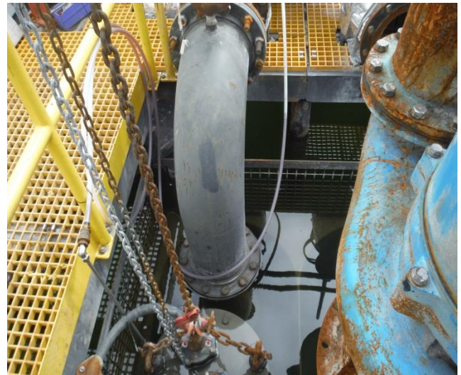
Photo 8: looking barge pump 1 with Winterhib anti-scalent line being added & tested.
