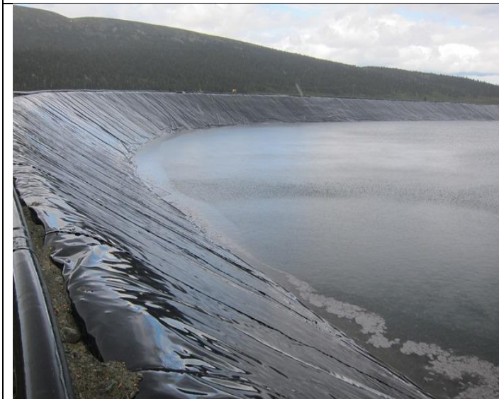
Photo 3: South-east corner view from east side of TSF.
