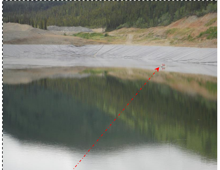
Photo 6: looking at Northwest corner from barge bathometric survey being performed.
