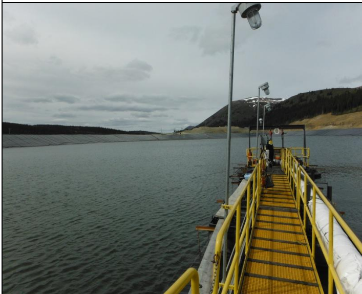
Photo 3: South wall view with walk way to the barge.
