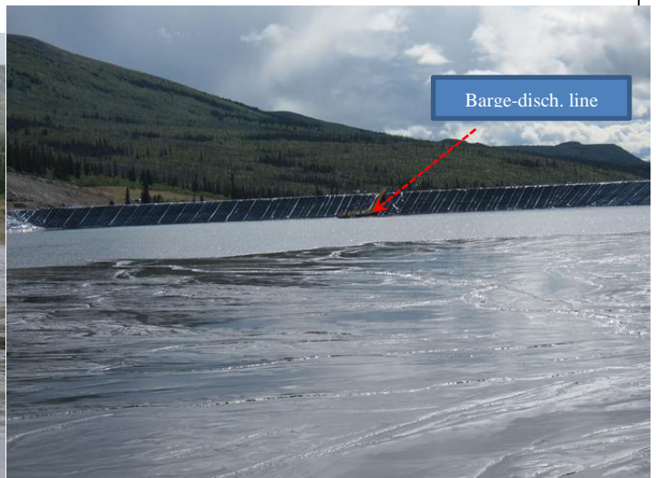
Photo 8: looking east from transfer station.
