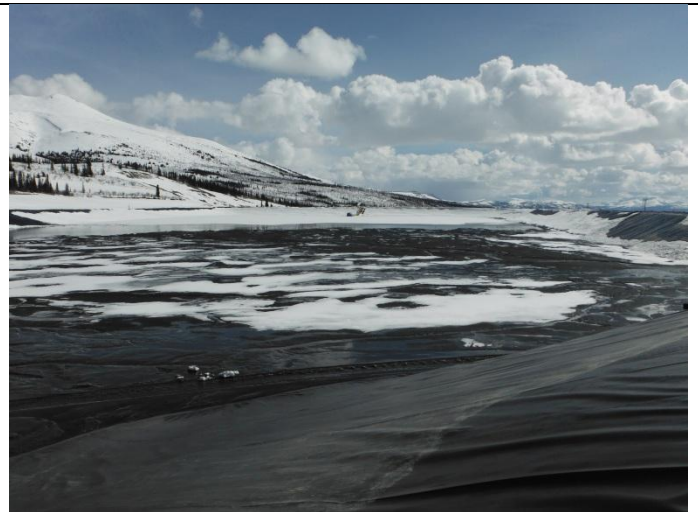
Photo 4: View of South Wall from North Wall
