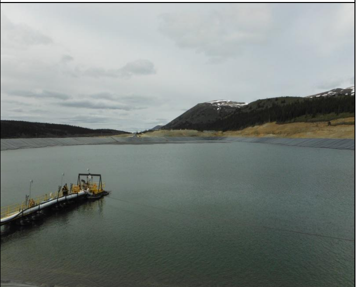
Photo 4: View of South Wall from North Wall
