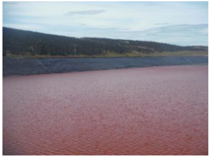
Photo 4: View of South-west wall from the South side of TSF.
