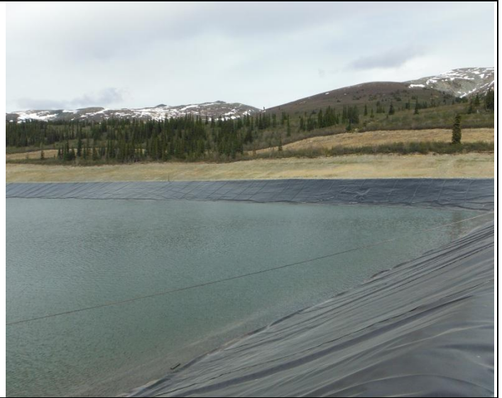
Photo 6: looking at east wall from South wall.
