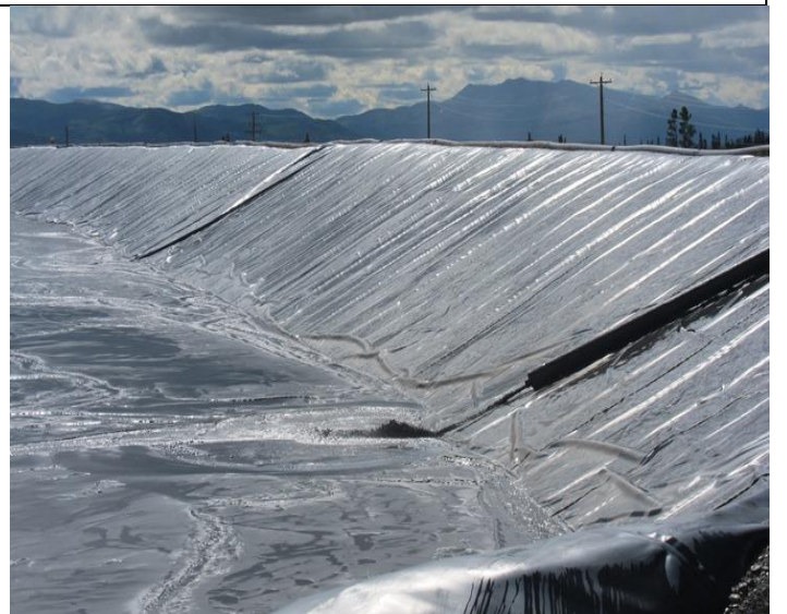
Photo 4: View of South Wall with tailing slurry discharging- enough room for the tailings.
