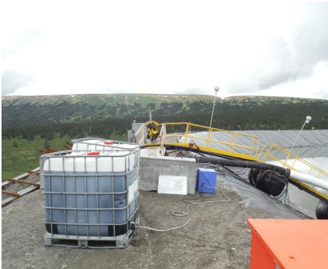
Photo 7: looking at Winterhib anti-scalent at east dam of TFS.
