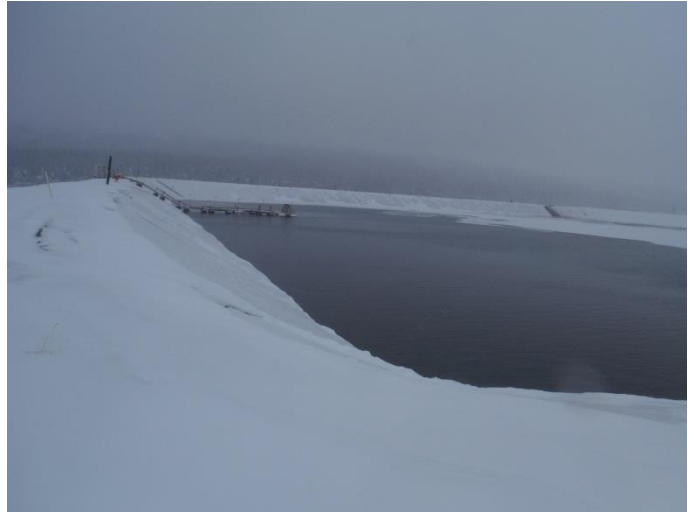
Photo 2: Looking at the south wall of TSF.
