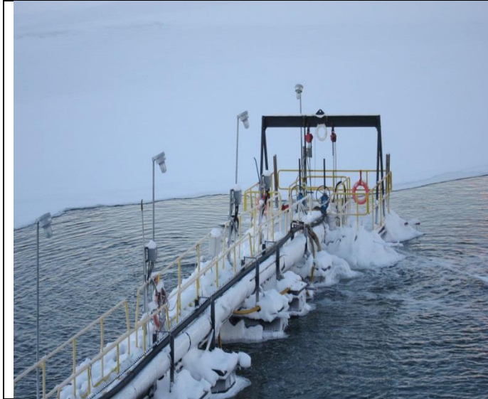
Photo 1: Looking at barge station.
