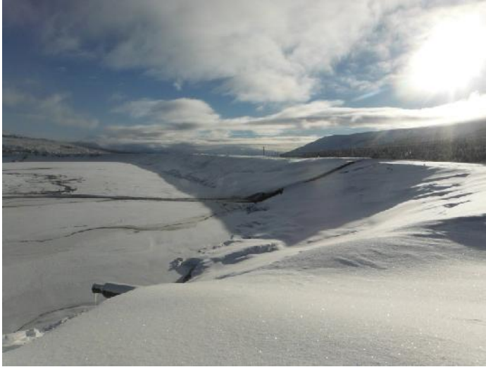
Photo 1: Looking at mill tailings discharge line with pump reclaim water pump house overflow line in foreground
