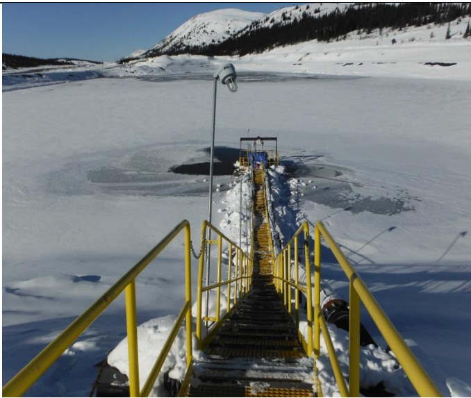
Photo 3: South wall view with walk way to the barge.
