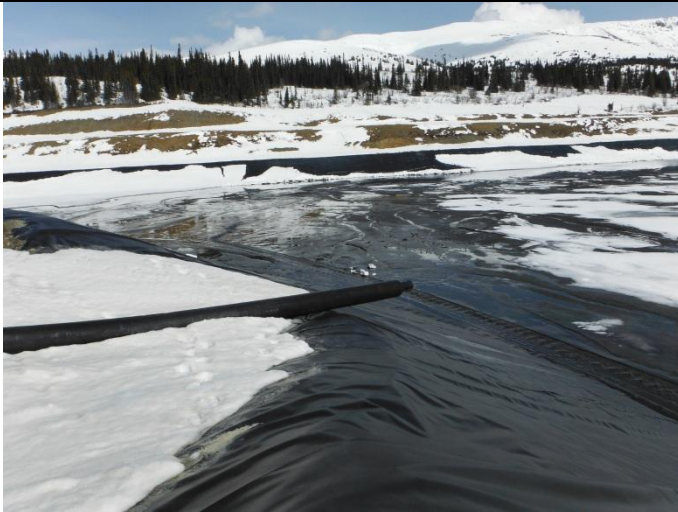
Photo 1: Looking at transfer station over flow line from North West corner of TSF
