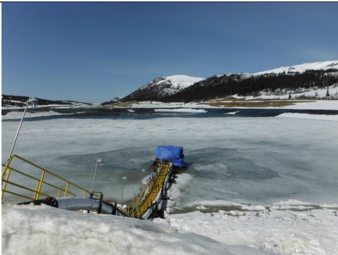
Photo 3: South wall view with walk way to the barge.
