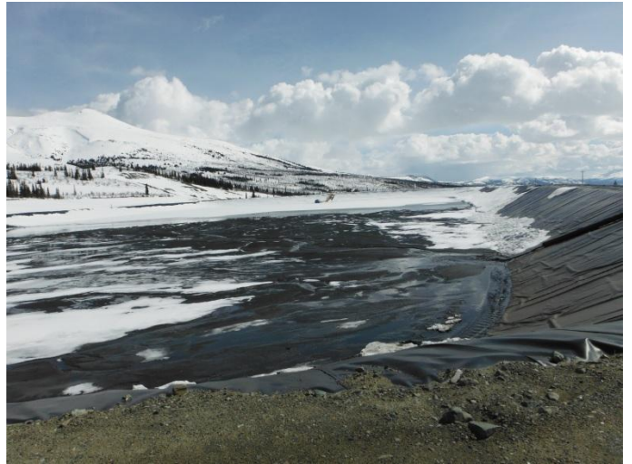
Photo 8: looking south east from transfer station.
