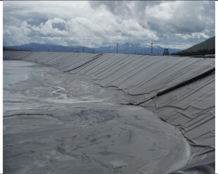
Photo 2: Looking at south wall from North West corner of TSF with Tailing discharge line in foreground.
