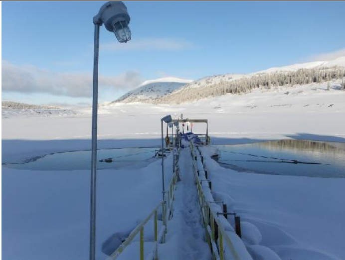
Photo 7: looking north from barge ramp
