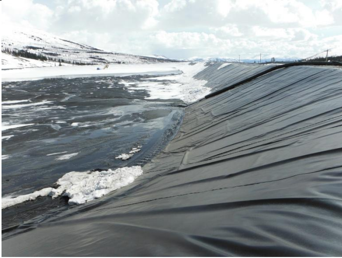
Photo 7: looking at tailings discharge from north west corner of TSF.
