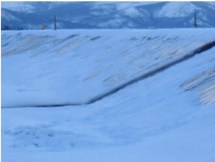
Photo 7: View of tails discharge pipe at center south of TSF.
