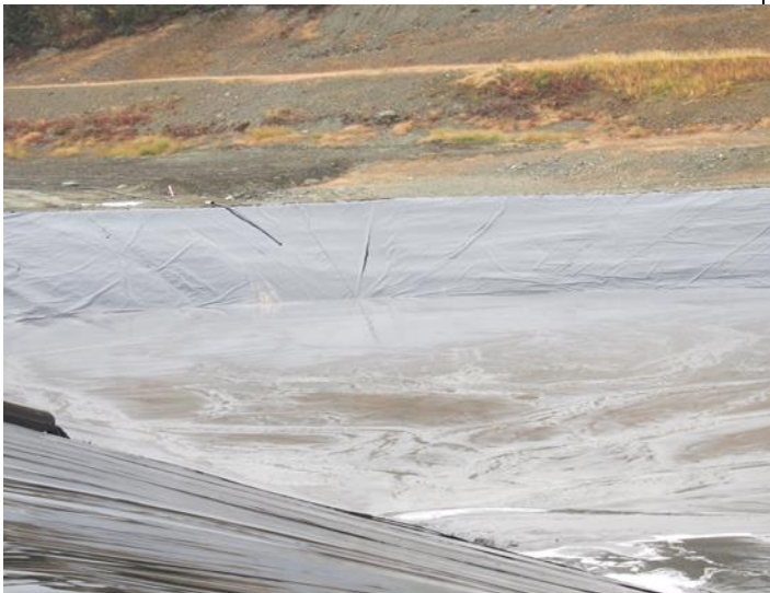
Photo 3: Closer view of discharge pipe location North-west corner of TFS.
