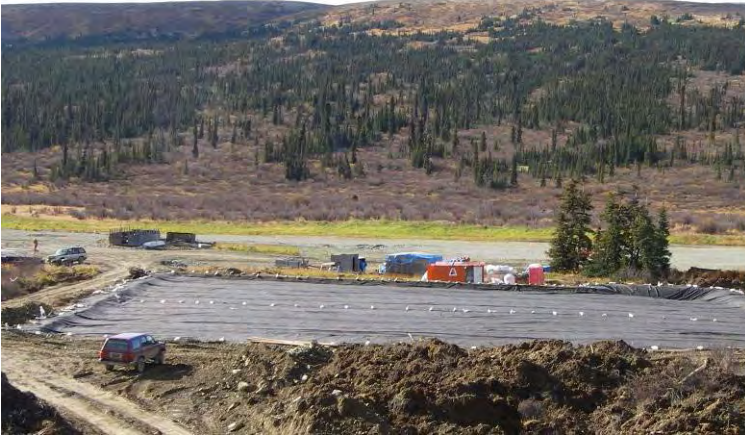
16/09/07 Geotech lined LTF cell, prior to liner installation (W)
