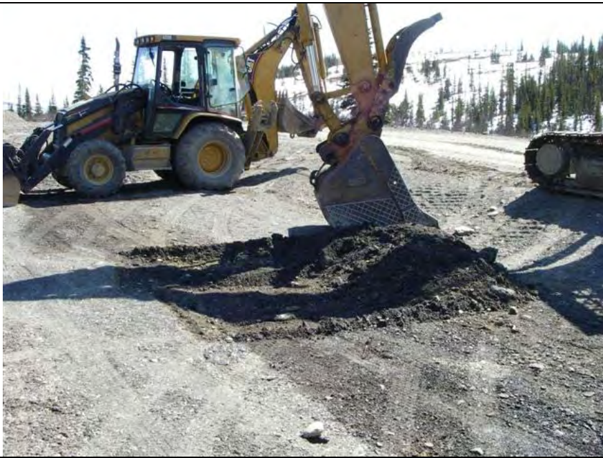
Photo 4. Start of contaminated soil excavation (approx. 30 cm deep). Taken May 23, 2007
