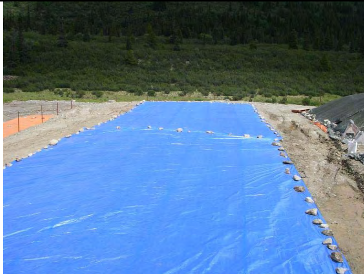
Photo 3 07/26/07 Final tarped cell; facing east
