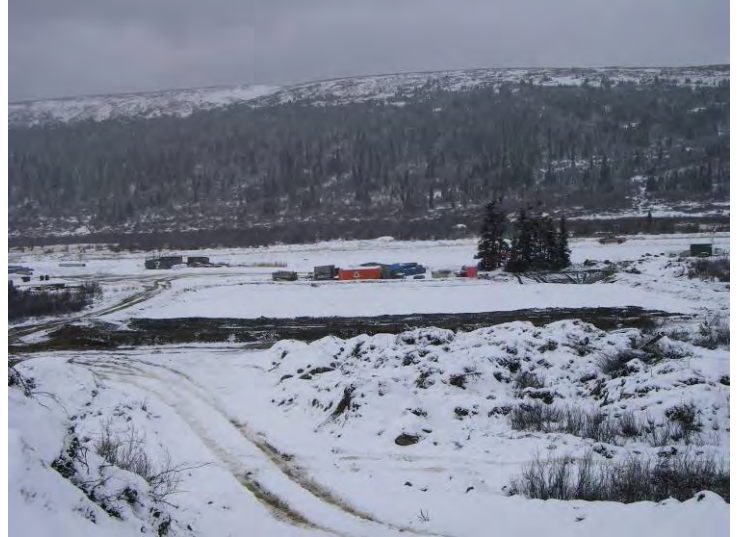
09/27/07 Soil moved into the LTF (~15" height) facing west
