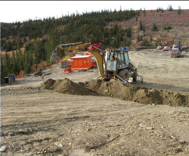
14/09/07 Sloping the cell to drain into the sump (N)
