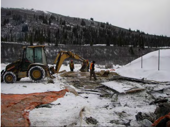
10/07/07 Moving plywood on soil storage berm
