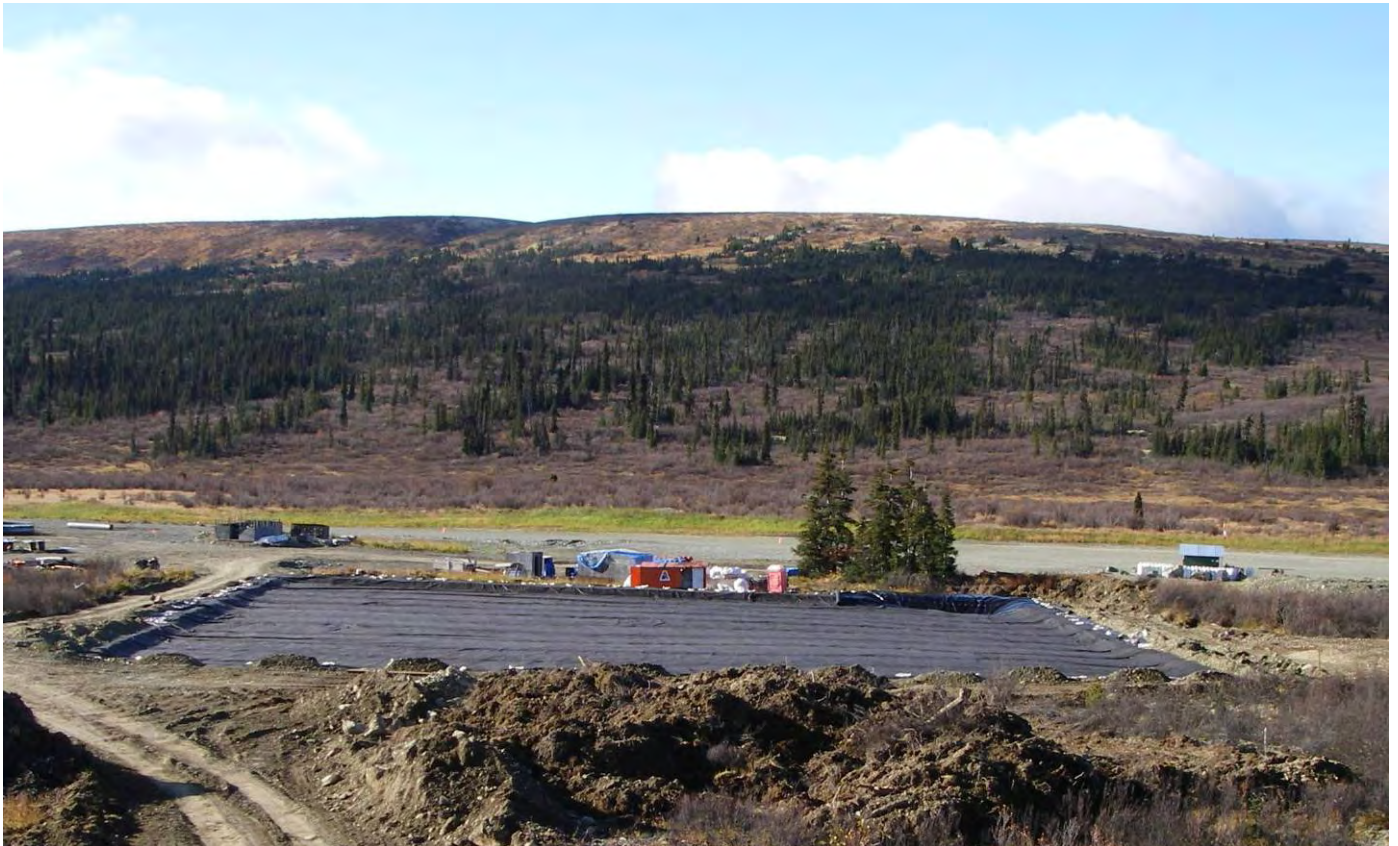
18/09/07 Completed LTF cell (W)
