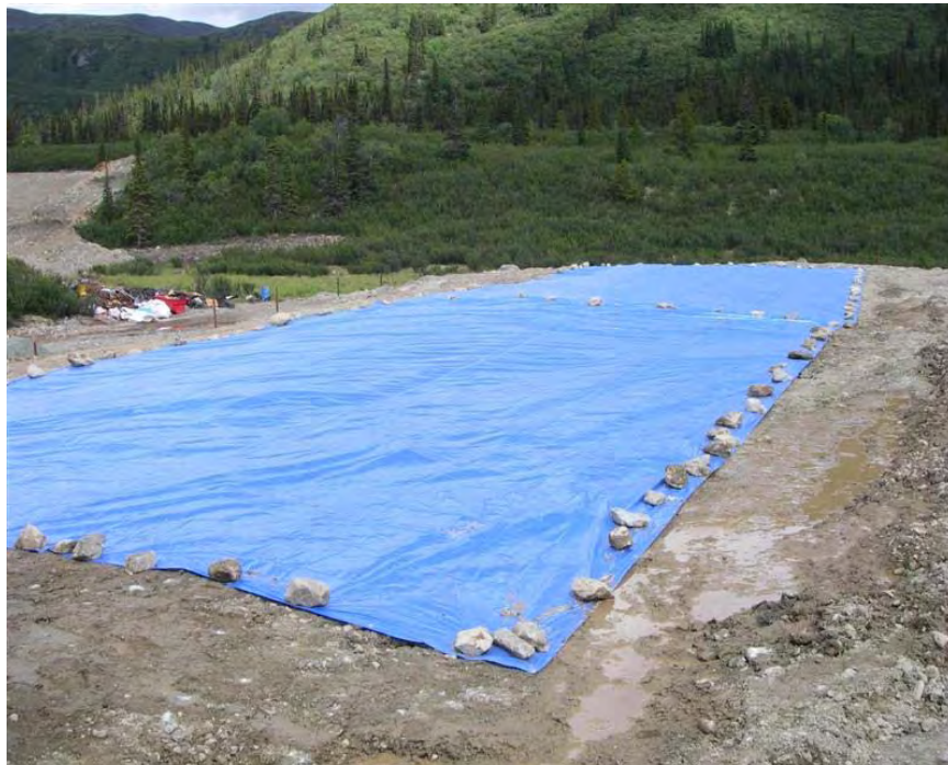
Picture 3-1 Tarped Cell 1 (July 26 th , 2007)
