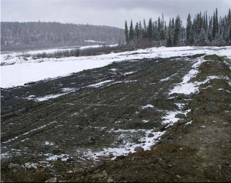
09/27/07 Soil moved into the LTF (~15" height) facing north west
