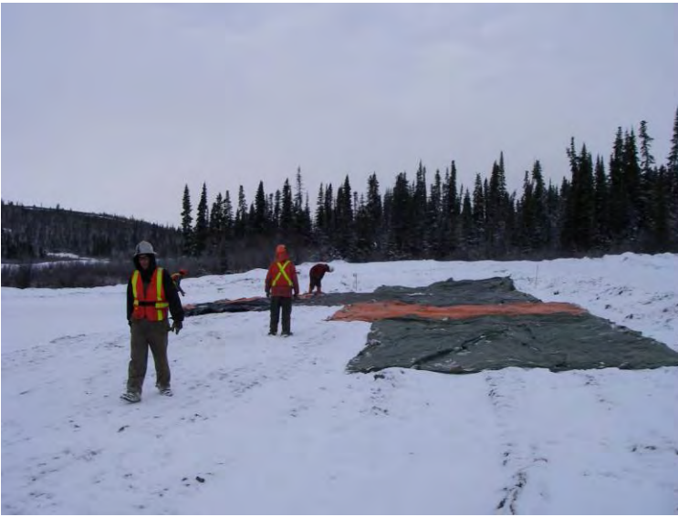
10/07/07 Tarp over ½ of the stored soil in the LTF
