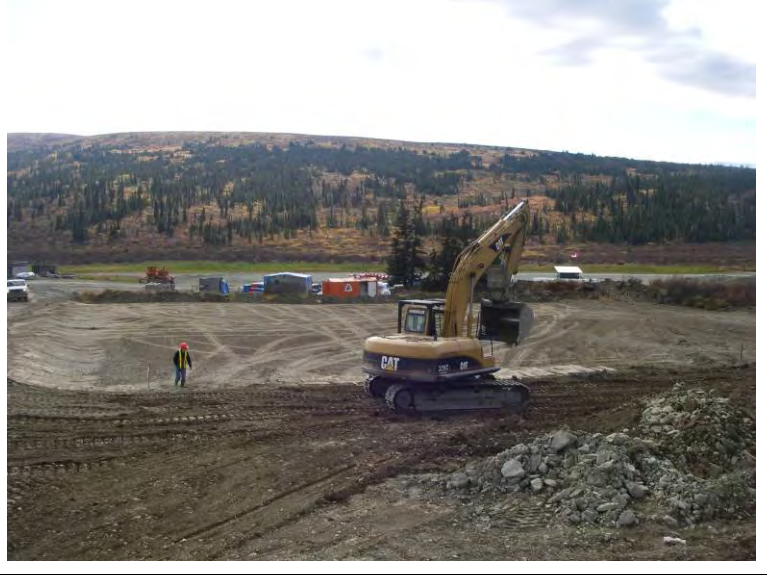
13/09/07 Cleared and grubbing of site (facing W)
