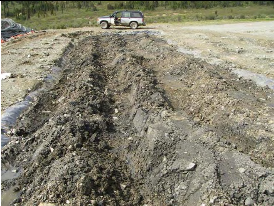
Photo 3 06/18/07 Containment cell after windrowing; facing south-west
