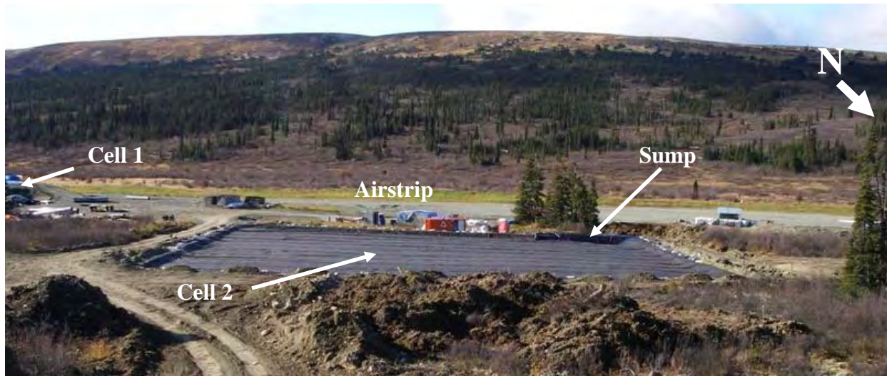
Picture 3-2 Completed Cell 2, prior to acceptance of soil (Sept 18 th , 2007)
