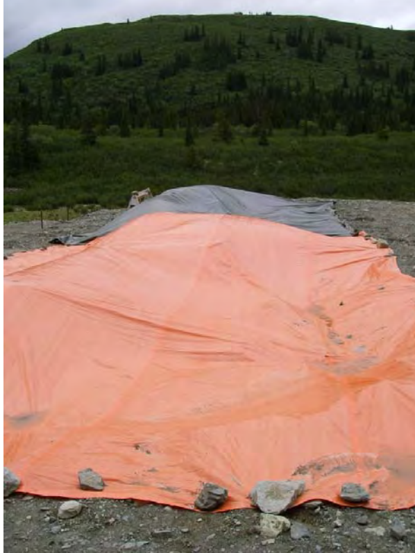
Photo 1 07/10/2007 Tarpred LTF cell: facing east
