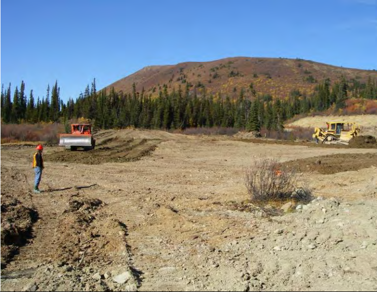
12/09/07 Clearing and grubbing of site (facing N)
