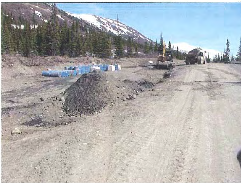
Figure 3: Excavation of Contaminated Soils with “Smear Zone” Soils in the Foreground.
