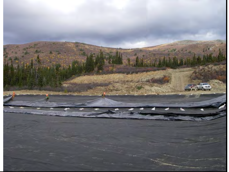
16/09/07 Liner installation (NNE)
