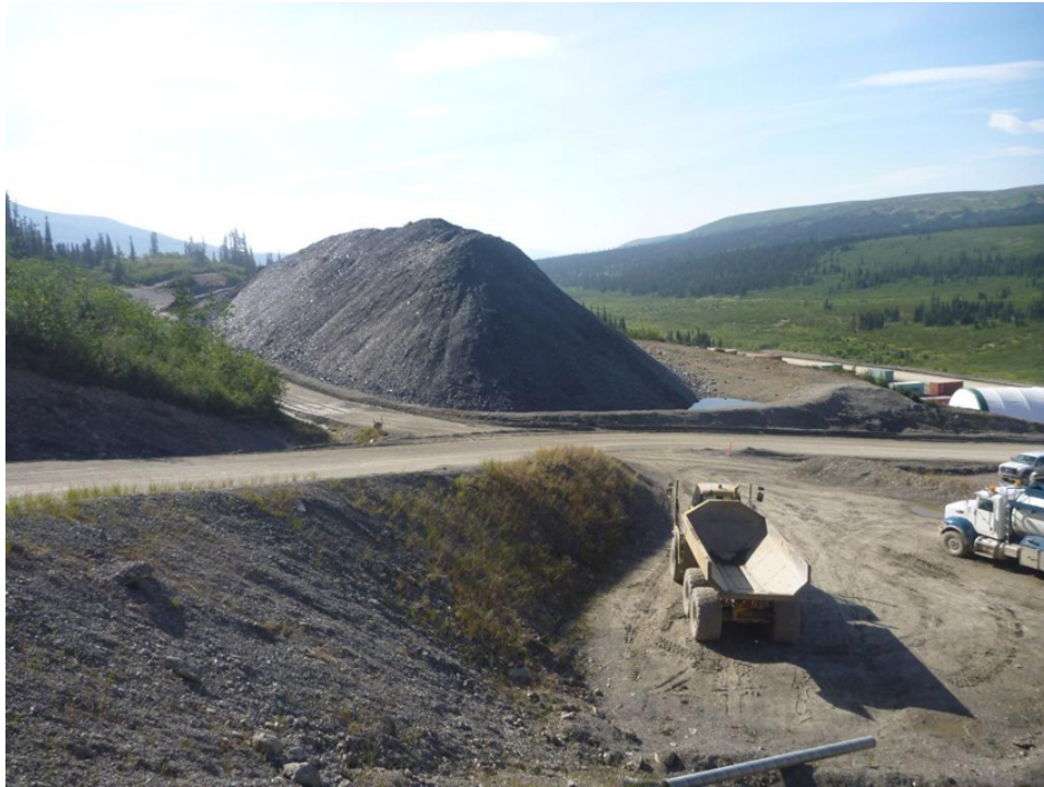
Photo 5-1: Waste Rock Pad #1, East of the Camp (July 2013)
