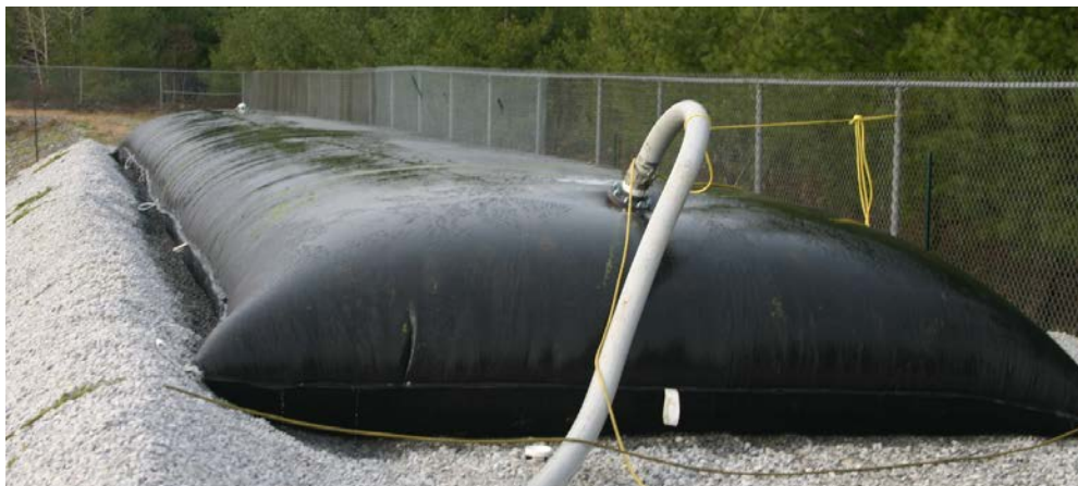
Figure 8 Example of a Geotube in Operation
