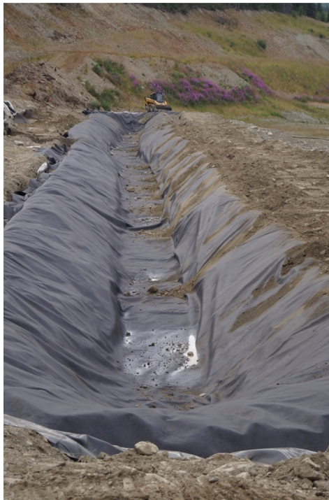
Photo 2-1: Bioreactor Trench (July 12, 2016)
