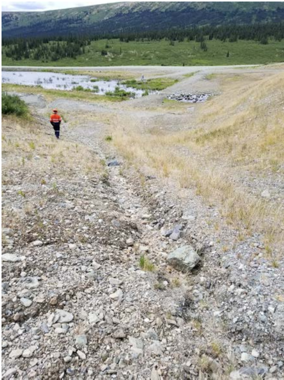
Photo 18 Minor erosion gullies on downstream slope
