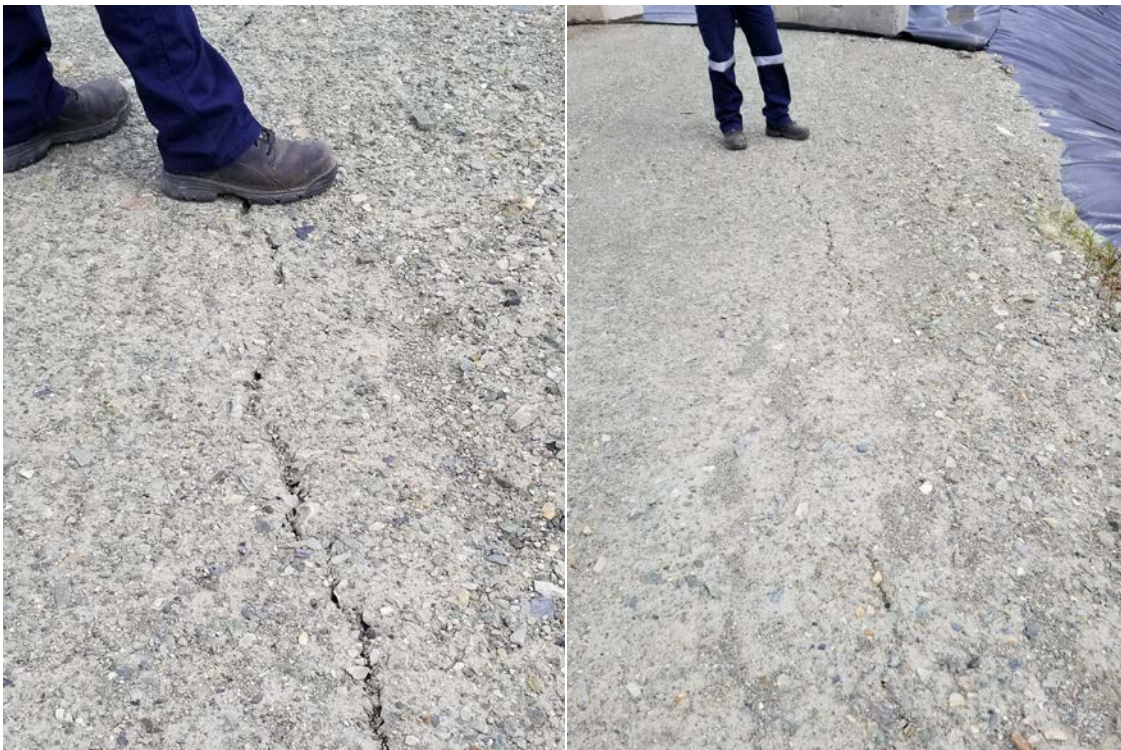
Photo 24 Cracking in dam crest near north end slump
