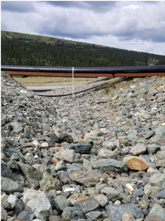
Photo 40 Discharge pad for vacuum trucks
