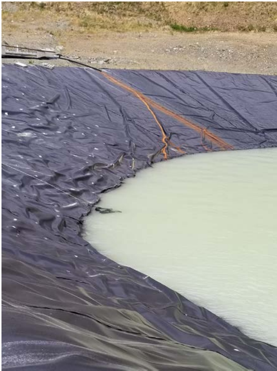
Photo 28 Animal burrow into liner
