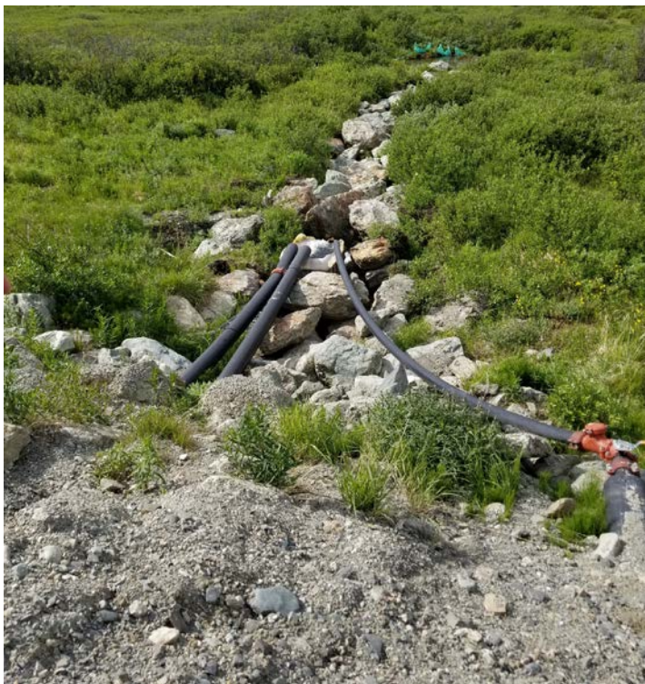
Photo 10 Discharge from under drain pipes downstream of seepage pond
