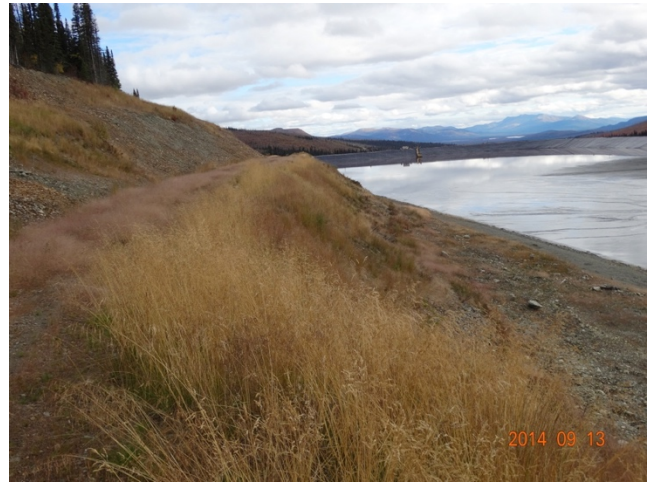
Photo 2-5: Revegetation Slong the TSF (September 2014)
