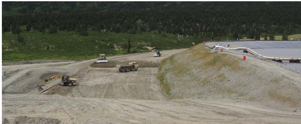
Photo 2-3: Construction of the Ultimate TSF dam; Note Seeding on the Starter Dam Face has Resulted in ~50% Grass Cover Between the Crest and Construction Zone (July 2012)
