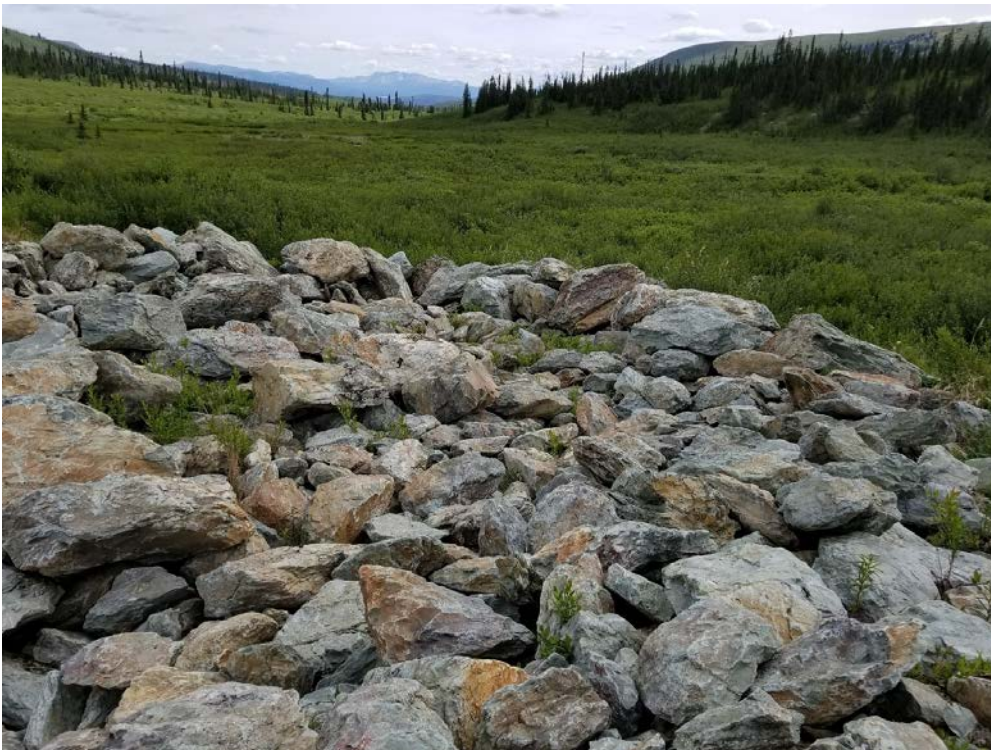
Photo 34 Ditch B Discharge Pad
