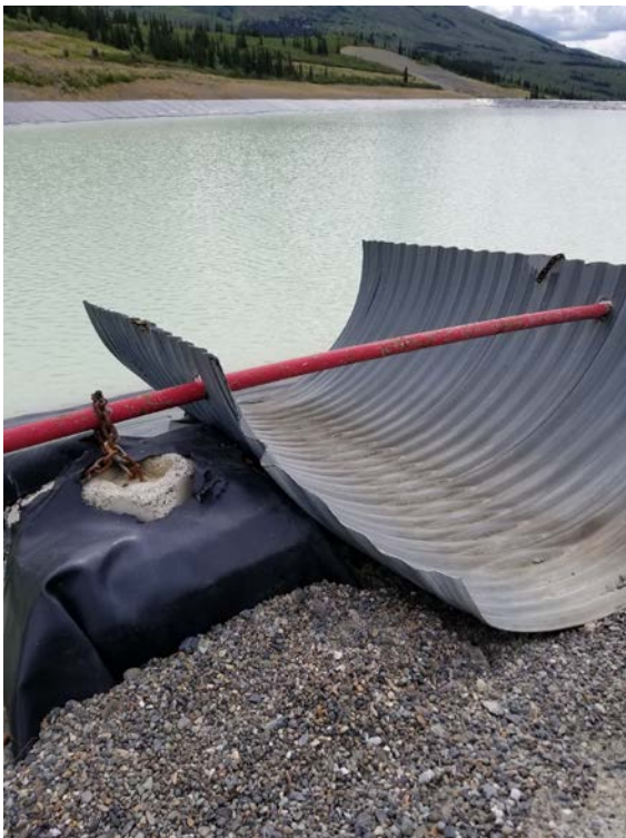
Photo 40 Discharge pad for vacuum trucks
