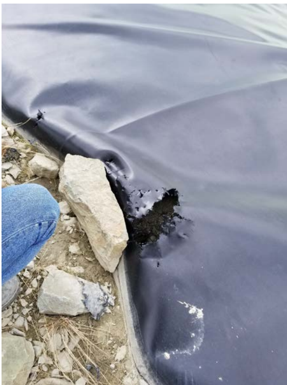
Photo 28 Animal burrow into liner
