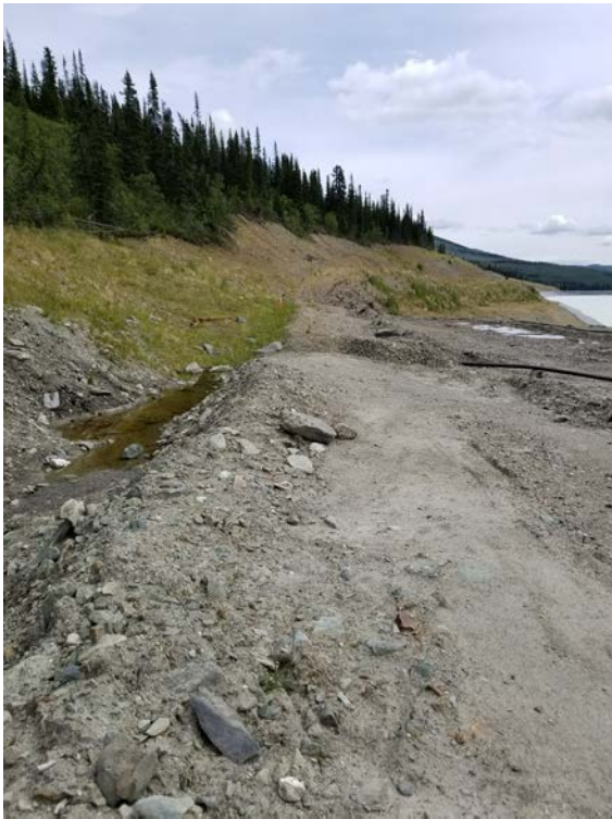
Photo 47 Ditch A Adjacent to Biopass
