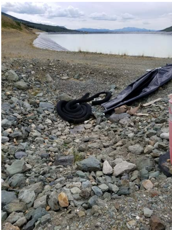
Photo 12 Upstream end of under drains
