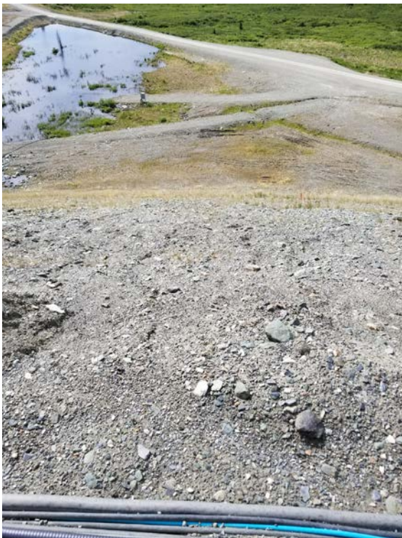
Photo 18 Minor erosion gullies on downstream slope
