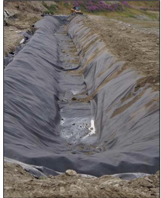
Photo 5-5: Bioreactor Trench Lined with Geotextile Fabric (July 12, 2016)
