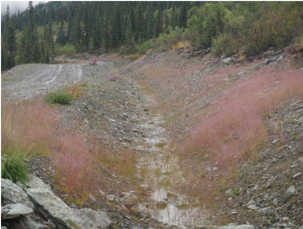
Photo 2-1: Looking North at Established Vegetation in Coarser Material Along Ditch B (August 2011)
