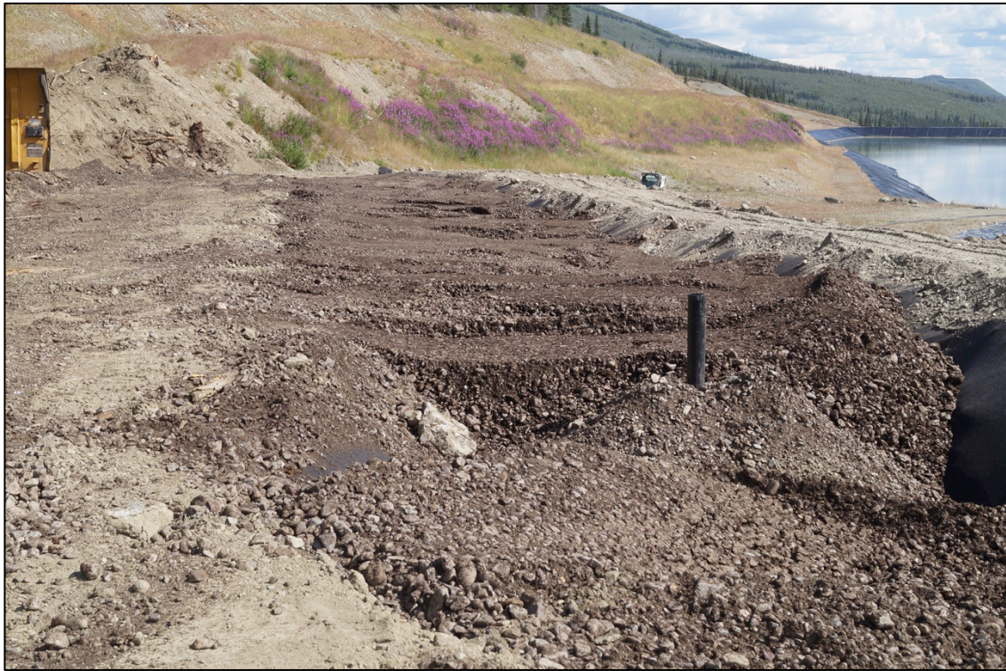
Photo 5-7: Bioreactor Filled with Substrate Material (July 16, 2016)
