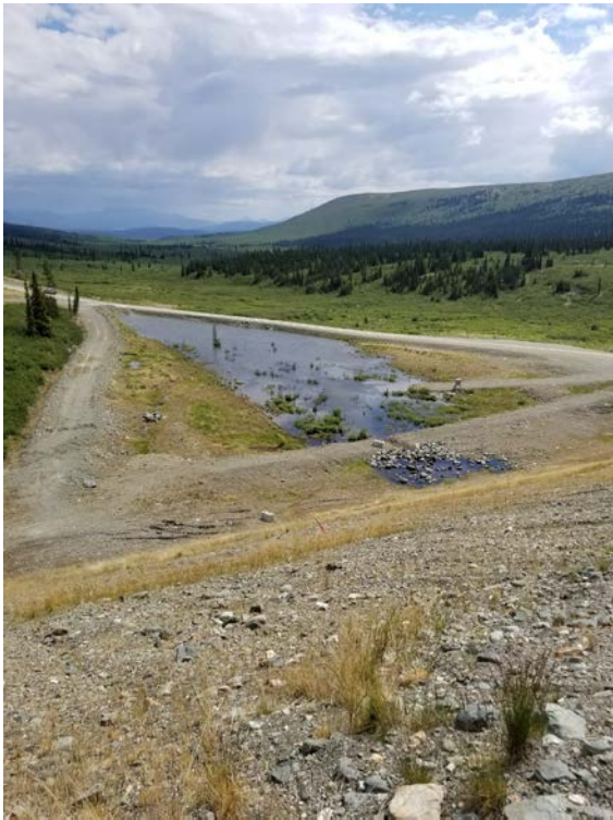
Photo 10 Discharge from under drain pipes downstream of seepage pond
