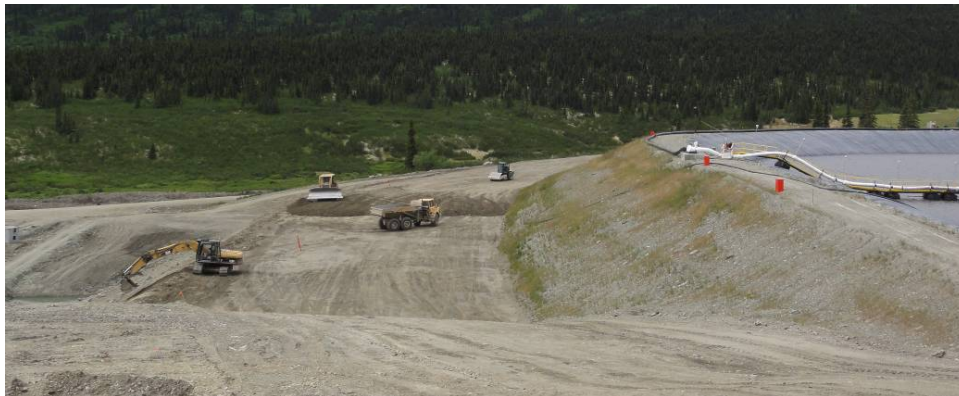
Photo 2-3: Construction of the Ultimate TSF dam; Note Seeding on the Starter Dam Face has Resulted in ~50% Grass Cover Between the Crest and Construction Zone (July 2012)
