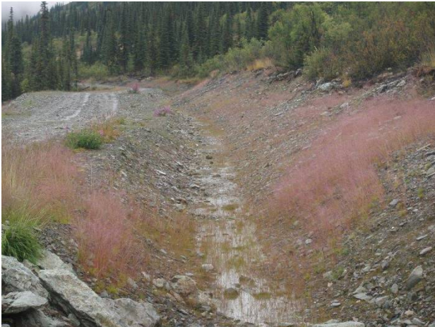
Photo 2-1: Looking North at Established Vegetation in Coarser Material Along Ditch B (August 2011)
