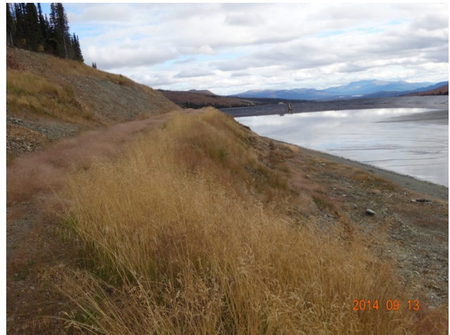
Photo 2-5: Revegetation Slong the TSF (September 2014)
