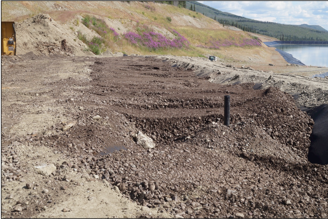
Photo 5-7: Bioreactor Filled with Substrate Material (July 16, 2016)
