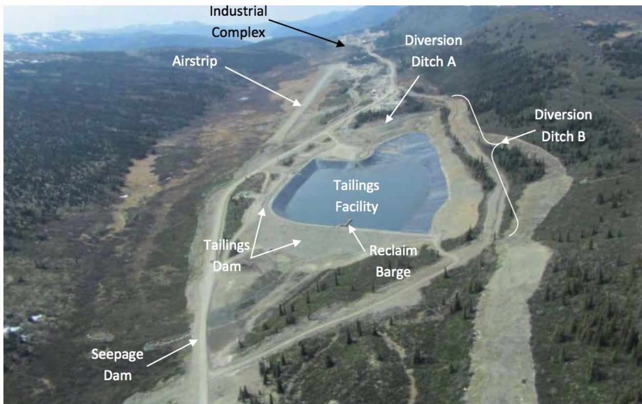
Figure 4-1: Tailings Storage Facility Layout
