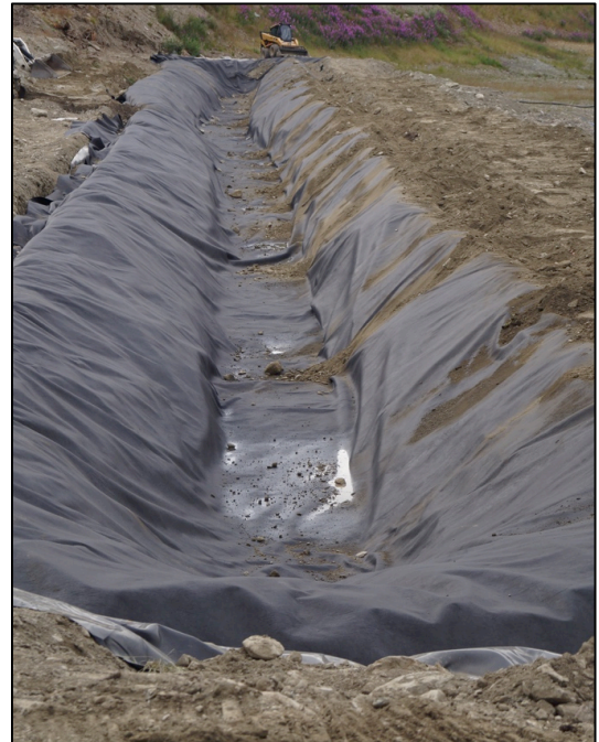
Photo 5-5: Bioreactor Trench Lined with Geotextile Fabric (July 12, 2016)
