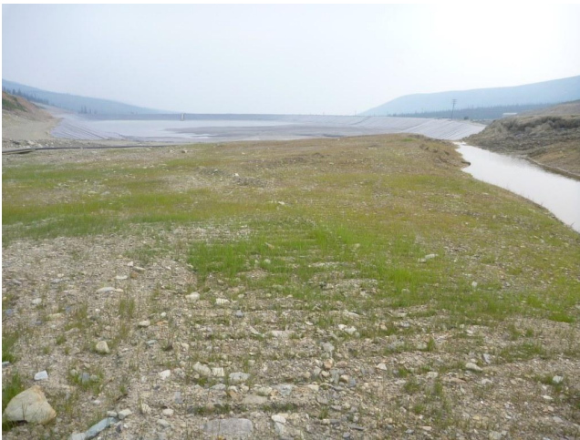
Photo 2-4: Looking South at Established Vegetation on Disturbed Ground Around the TSF Following Fall 2012 Seeding (July 2013)
