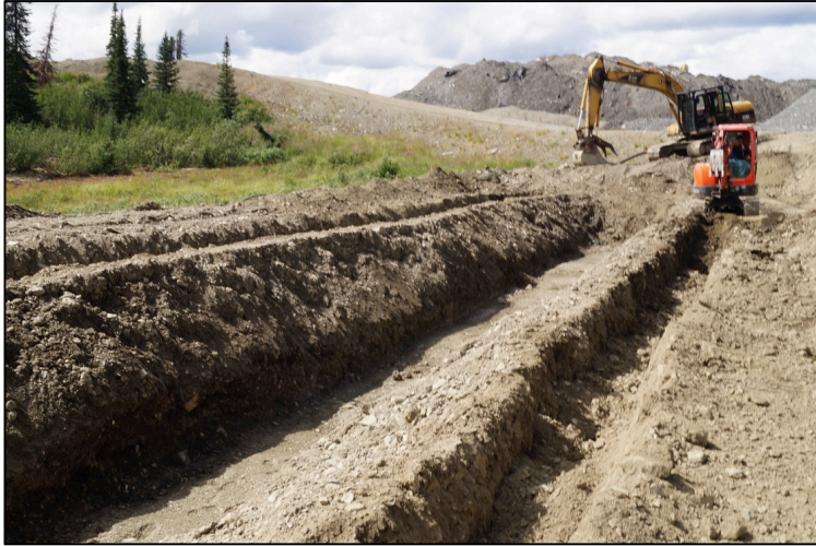
Photo 5-4: Bioreactor Trench (July 11, 2016)
