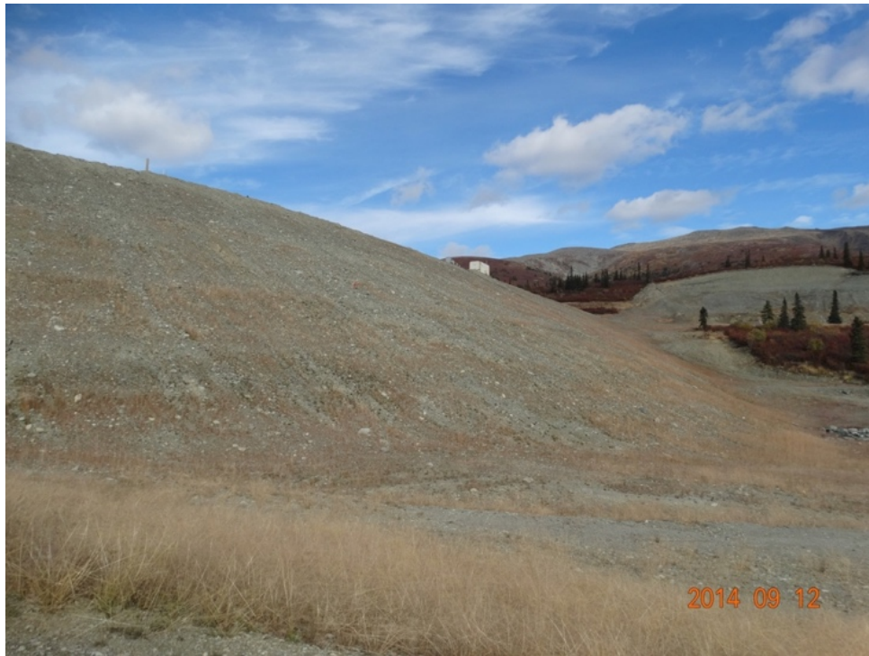
Photo 2-8: Revegetation Along the Downstream Face of the TSF Dam (September 2014)
