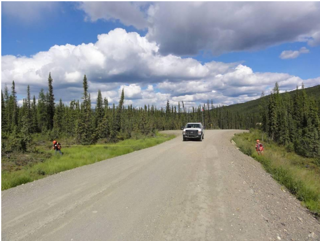
Picture 5-2: Example of revegetation (natural and from seed) along road corridor near km 3 (July 18, 2012)
