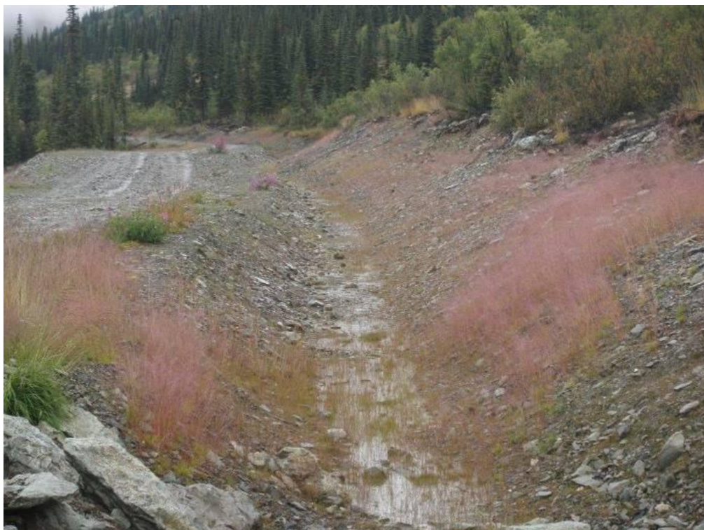
Picture 5-4: Looking north at established vegetation in coarser material along Ditch B (August 2011)
