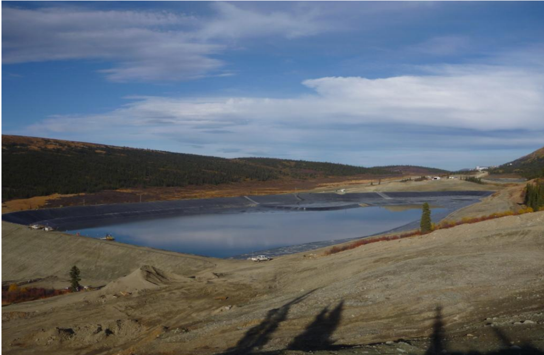
Picture 5-3: Ultimate tailings storage facility following dam lift construction project (September 21, 2012)
