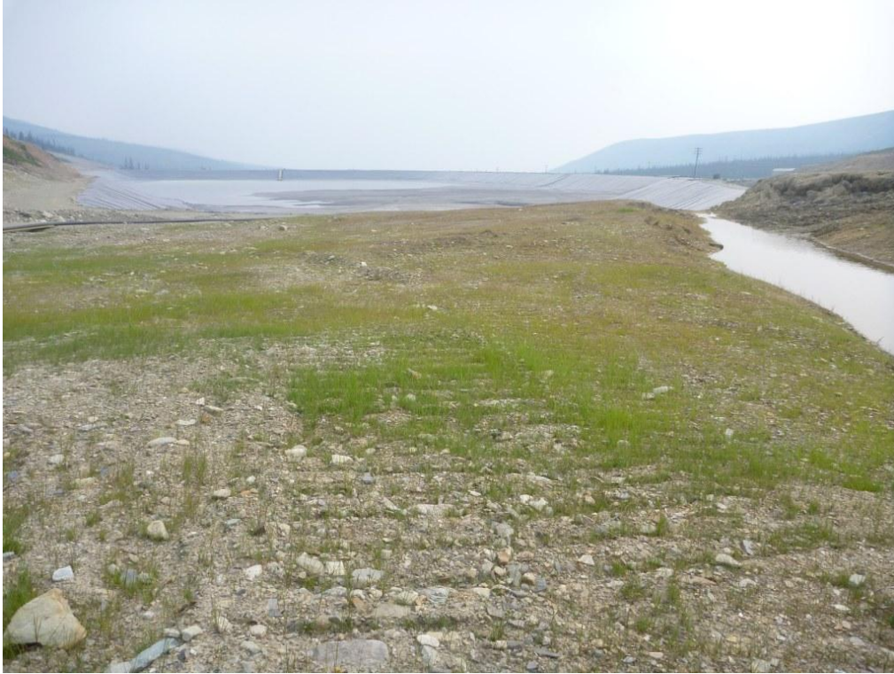
Picture 5-7: Looking south at established vegetation on disturbed ground around the tailings pond following fall 2012 seeding (July 2013)
