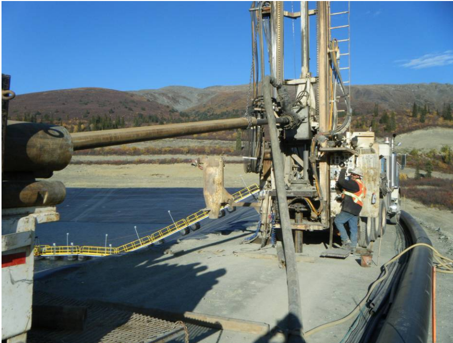
Photo 7 Instrumentation Installation Drilling
