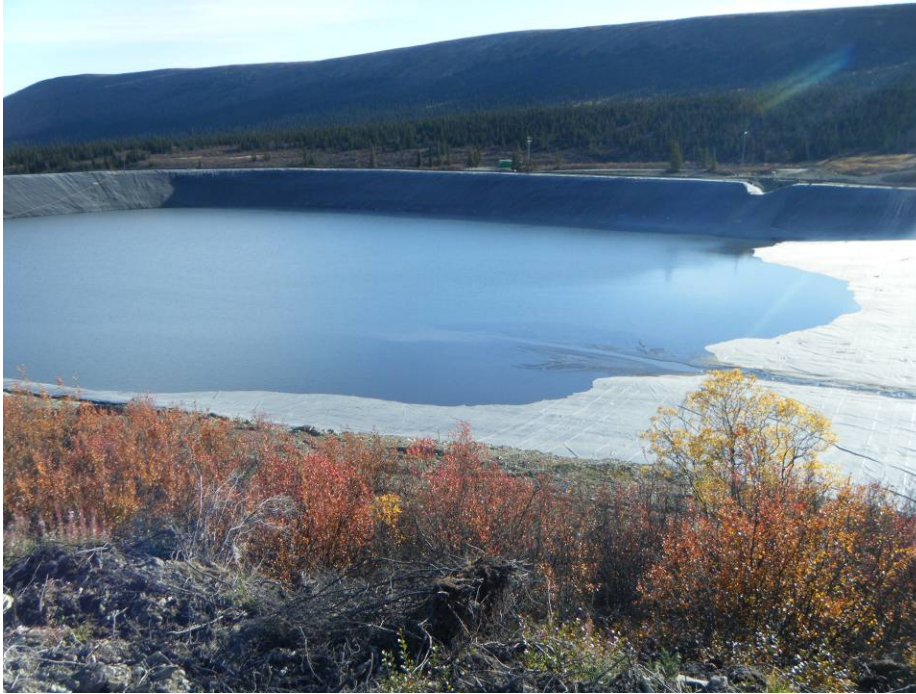
Photo 1 Completed Starter Spillway
