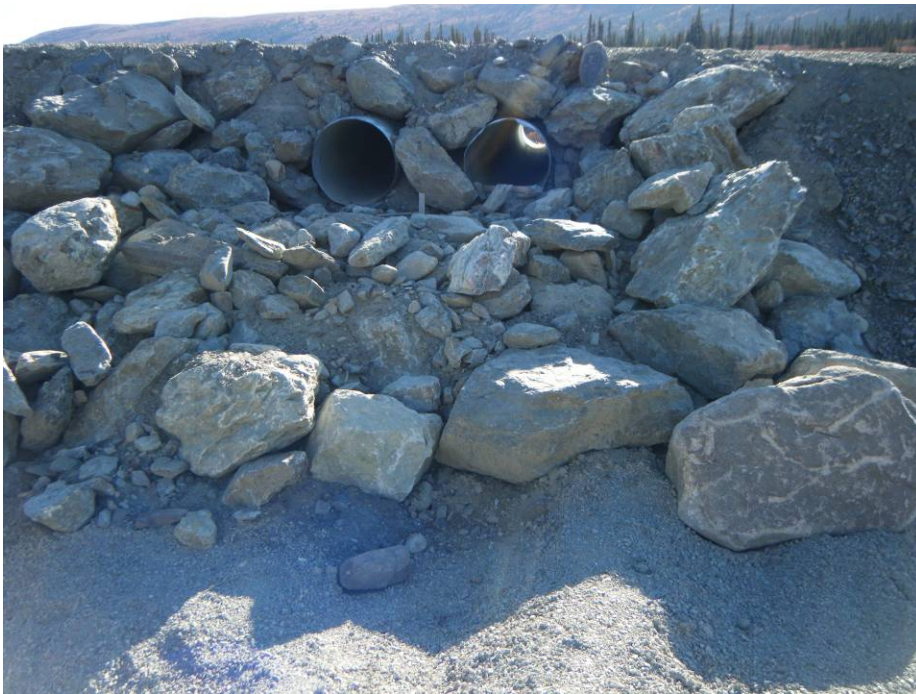
Photo 4 Seepage Collection Dam Spillway Inlet
