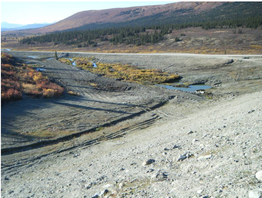
Photo 2 Seepage Collection Pond Area
