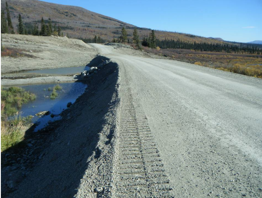
Photo 3 Completed Seepage Collection Dam
