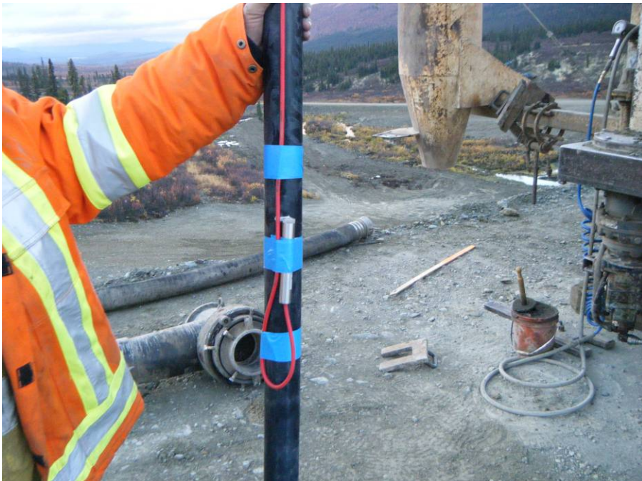
Photo 8 Vibrating Wire Piezometer taped to casing
