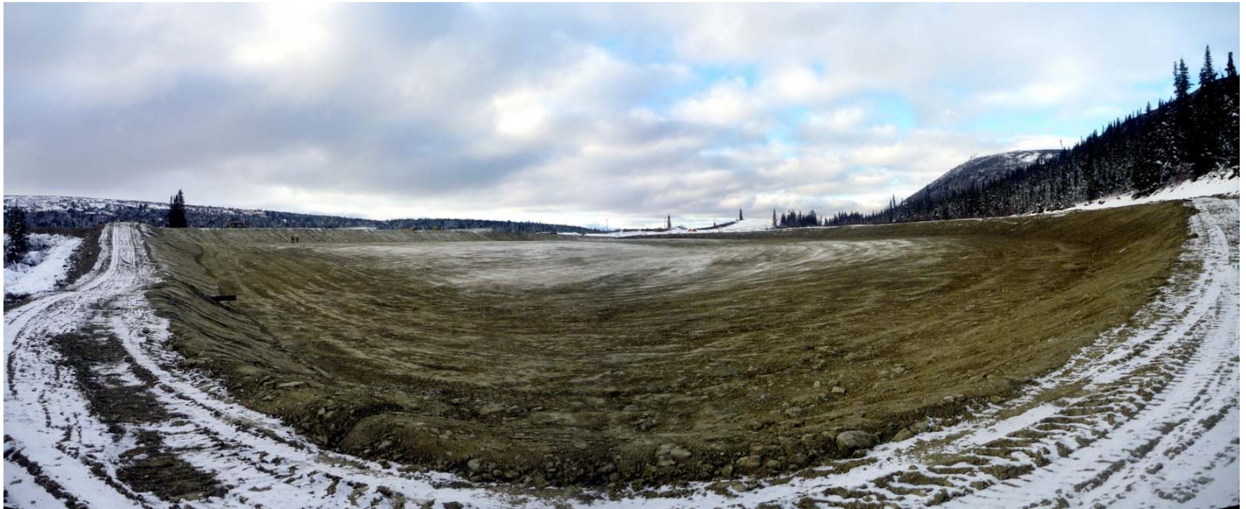
Photo 2 Waste Rock Storage Pad Liner Foundation
