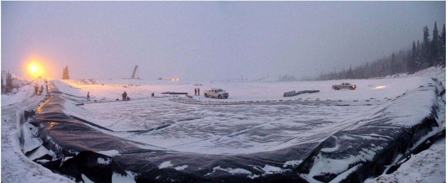
Photo 7 (11/11/01): Mid afternoon - looking west – 4 th & 5 th liner panels installed. The 2 nd geomembrane cloth cover is yet to be placed over the main liner. Steady southeast winds and snow. Sand bags placed onto the liner.
