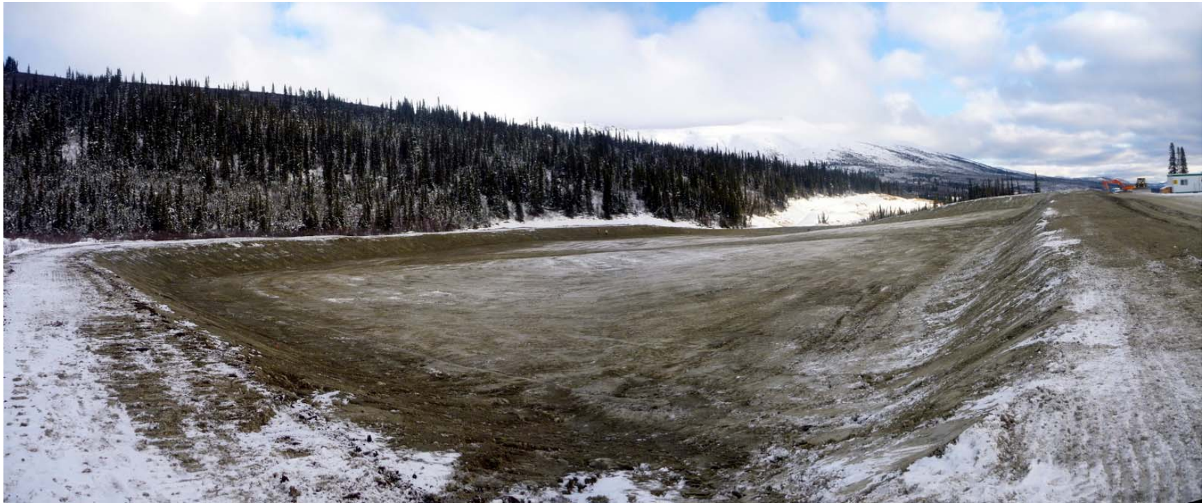
Photo 1 Waste Rock Storage Pad Liner Foundation
