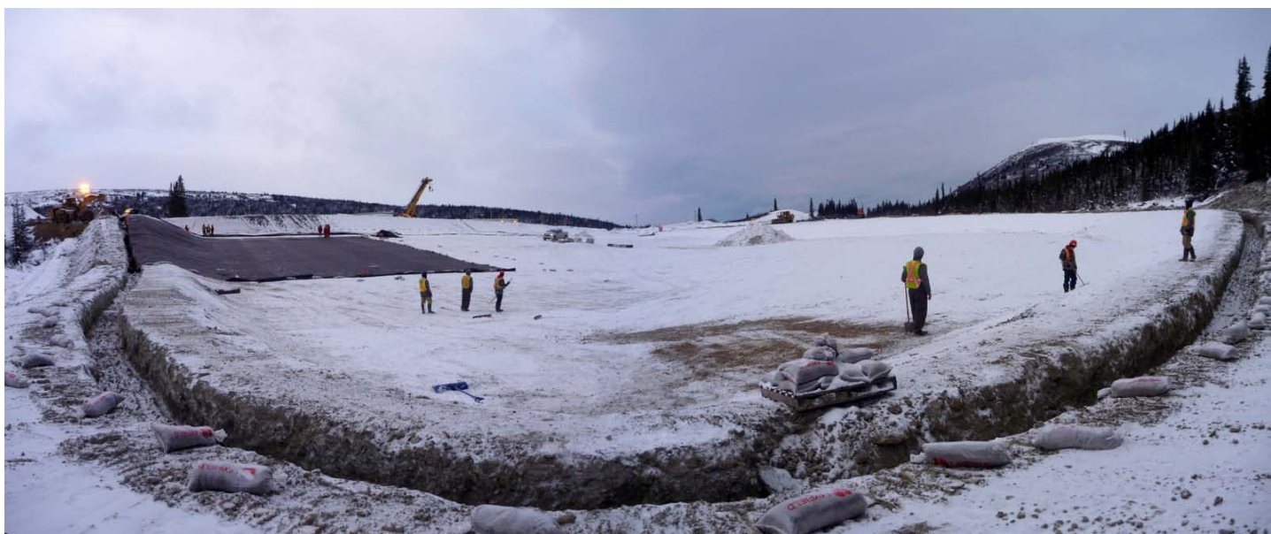
Photo 7 (11/11/01): .Looking west – Midmorning 3 rd liner panel installed along the southwest wall; snow removal within the pad and trenching the anchor trench along the perimeter of the pad.
