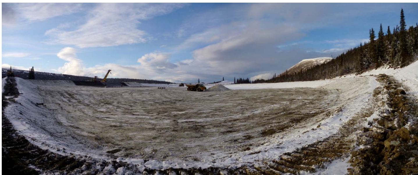
Photo 7 (11/10/30): .Looking west – installing geo-membrane cloth and G-panel liner along the southwest wall; snow removal within the pad and trenching the anchor trench along the perimeter of the pad.
