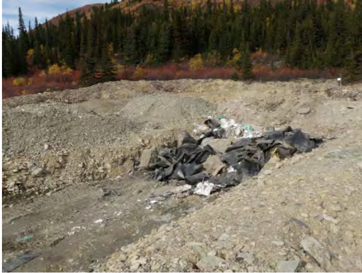
Picture 2-2: Active cell containing waste with cover material adjacent to the cell.
