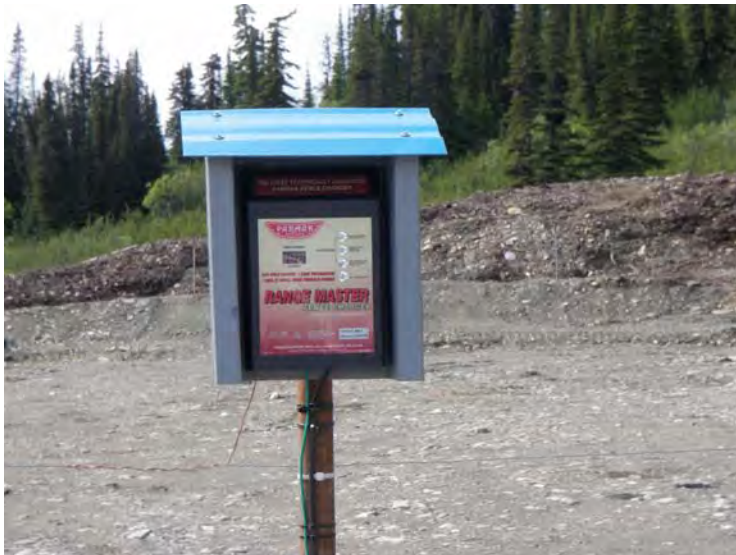
Picture 2-5: High Voltage Bear Fence.
