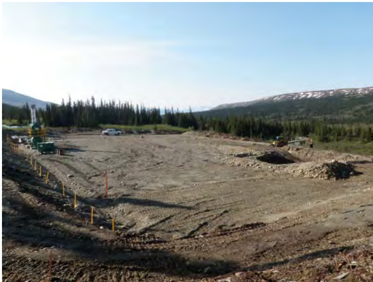
Picture 2-1: Active (middle right of picture) and future cells within the landfill. Note the electric fence that surrounds the landfill.
