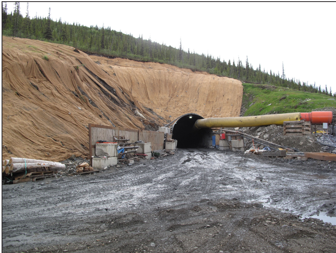
Bellekeno mine portal, Keno Hill silver property.
