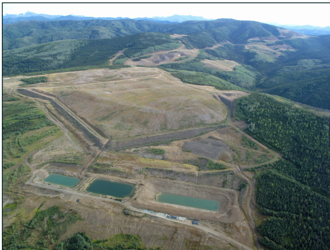
Brewery Creek gold property reclaimed heap leach pad and ponds in the foreground, 2009.
