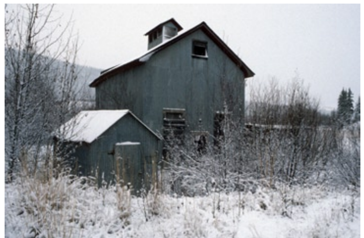
Pumphouse, Hunker Creek.
