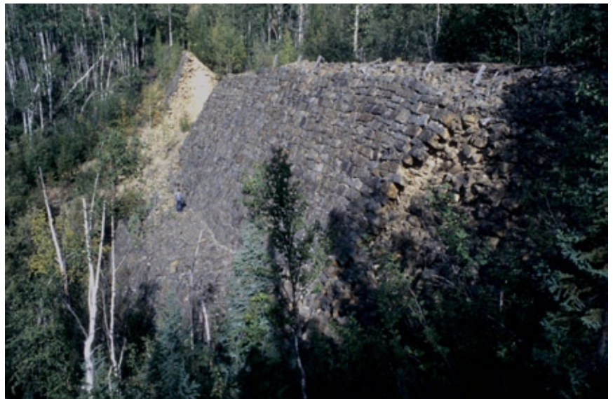
Dam at Adams Gulch
