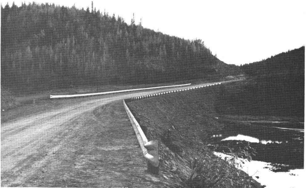
Figure 31 Location No. 131 - Mile 109 - Whitehorse-Mayo Highway, Y.T. This sloping area supports dense spruce up to 30 ft high with ground cover of feather moss, lichen and Labrador tea below which is peat 0 ft 9 in. thick overlying silty sand. The permafrost table is at the 2 ft 0 in. depth. September 22, 1964.
