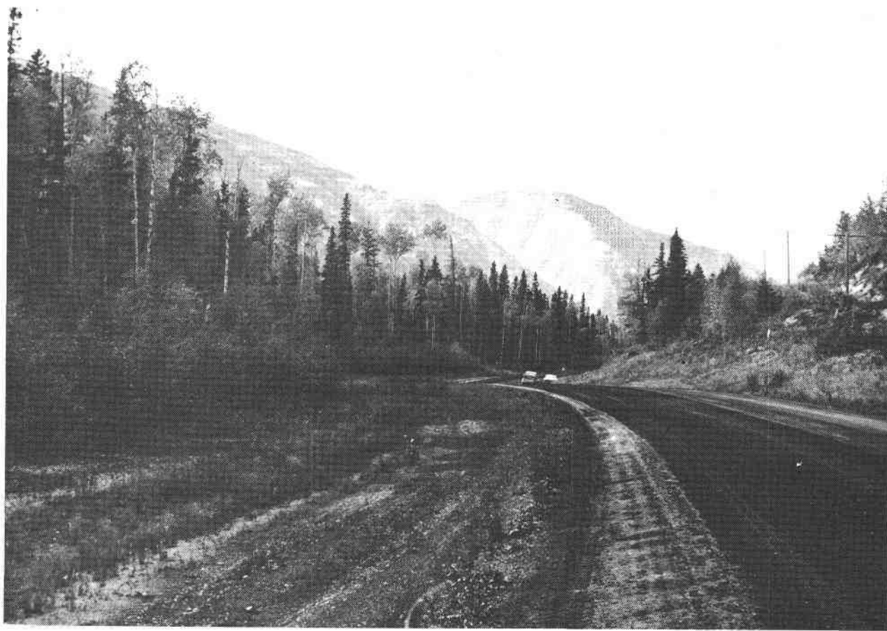
Figure 12 This high area located about Mile 500 on the Alaska Highway is typical of the high areas south of Whitehorse. The tree growth consists of tall spruce, jackpine and poplar. No permafrost was encountered in these locations. September 15, 1964.
