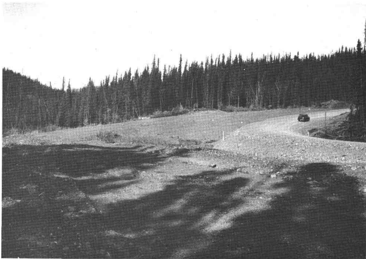
Figure 30 Location No. 128 - Mile 47 - Whitehorse-Mayo Highway, Y.T. This sloping area supports dense spruce up to 50 ft high with ground vegetation of continuous moss carpet below which is peat 1 ft 0 in. thick overlying brown silt. No permafrost was encountered above the road. Downslope from the road the permafrost table is at the 1 ft 0 in. depth. September 22, 1964.
