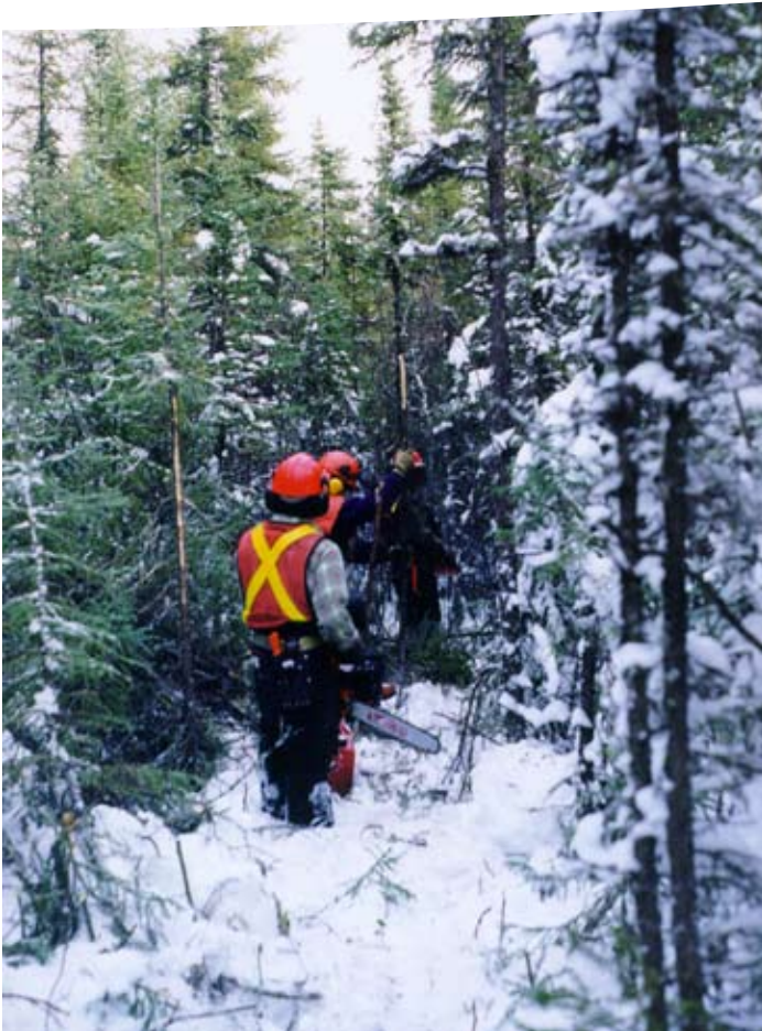
Hand cutting a seismic line photo: Lornel Consultants
