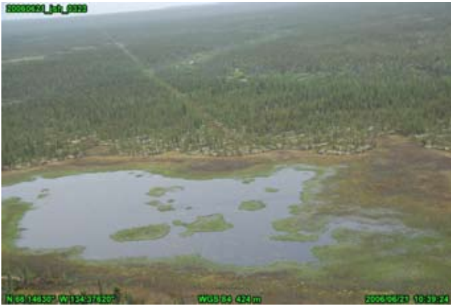
Use of lakes as a start point for winter construction photo: Canadian Wildlife Service/Ducks Unlimited, Yukon Government Seismic Line Regeneration Study, North Yukon
