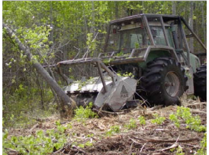
Mulcher selectively removing trees
