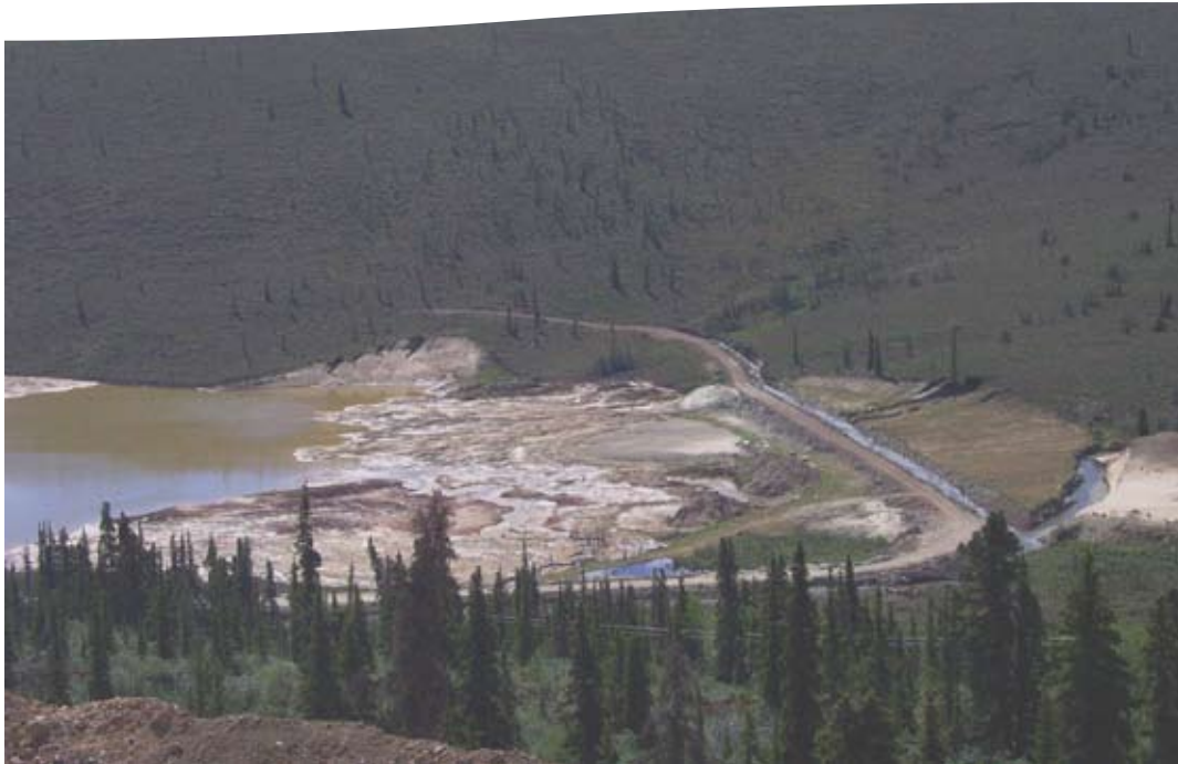
Stripping for road construction on a north facing slope with underlying permafrost resulted in significant thaw activity and movement of sediments into a waterbody
