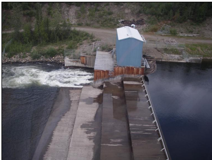
Figure 5-2 Mayo Lake Control Structure
