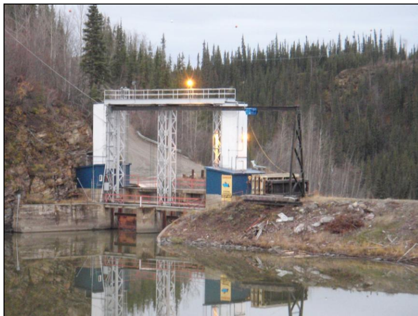
Figure 5-3 Top of Wareham Spillway
