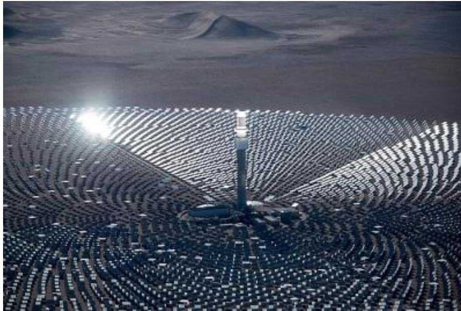
Figure 21 Crescent Dunes Solar Collector Site
