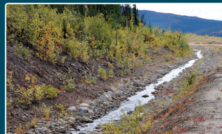
8. Faro Creek Diversion
