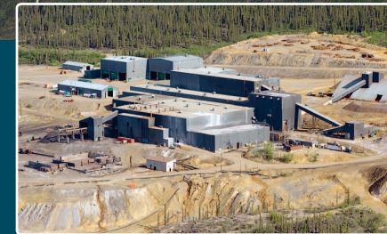
5. Mill Area - Faro Water Treatment Plant
