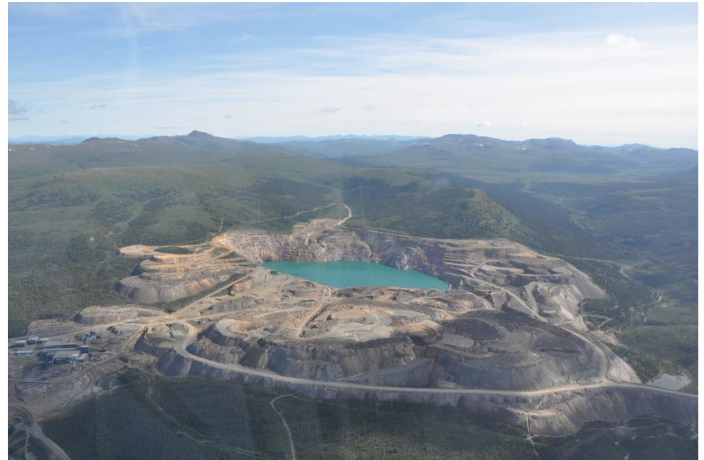
Aerial photo (looking North) Faro Pit and Waste Rock, and Mill Area on the bottom left
