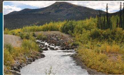
2. Rose Creek Diversion
