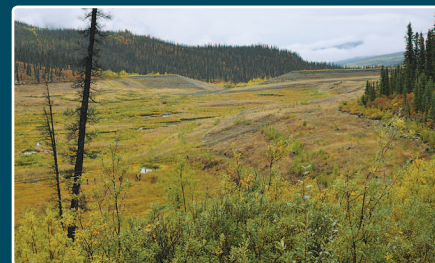
10. Fresh Water Supply Dam & Reservoir
