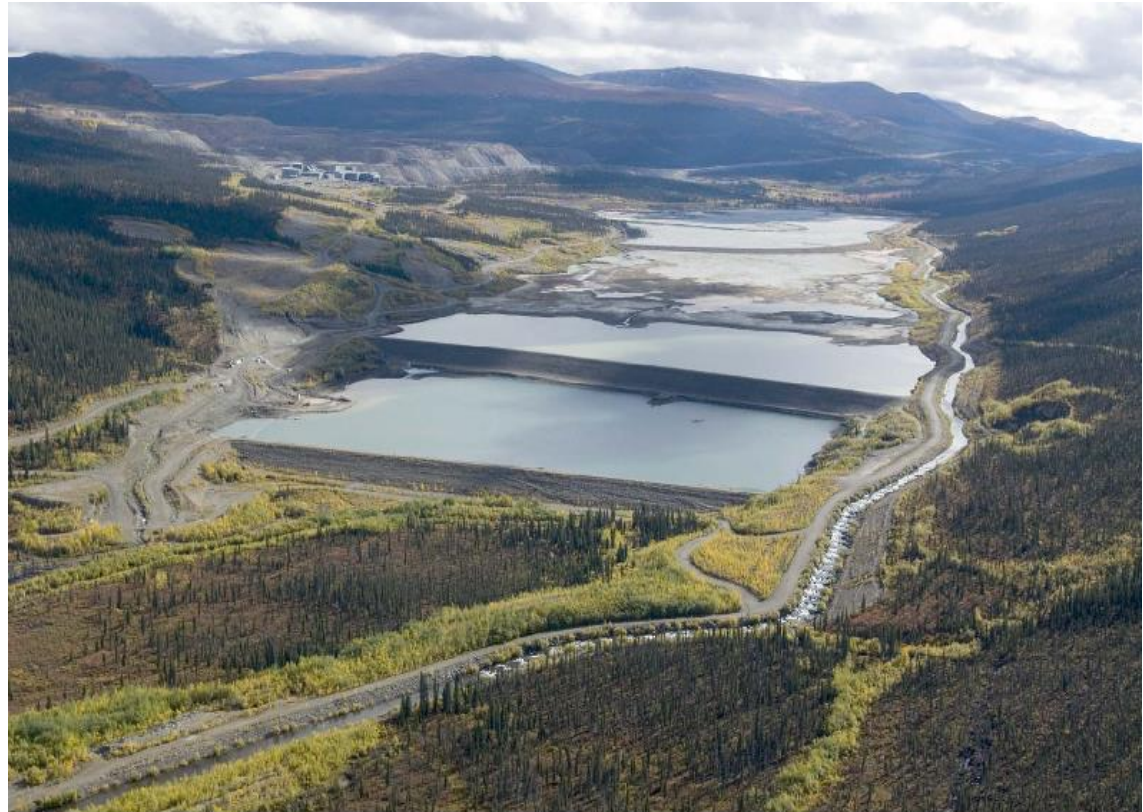
Looking East; CVP (closer), IP (farther), and RCD (right). Located within RCTA.
