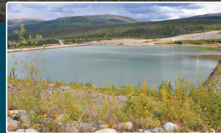
4. Cross Valley Pond & Dam
