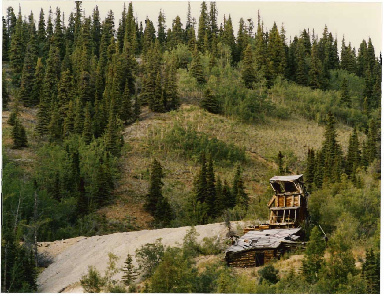
Plate 1 - 10 ton/day mill constructed by T.C. Richards and E. Kuebke in 1939 at No. 2 adit of LaForma Mine, Mount Freegold, Yukon
