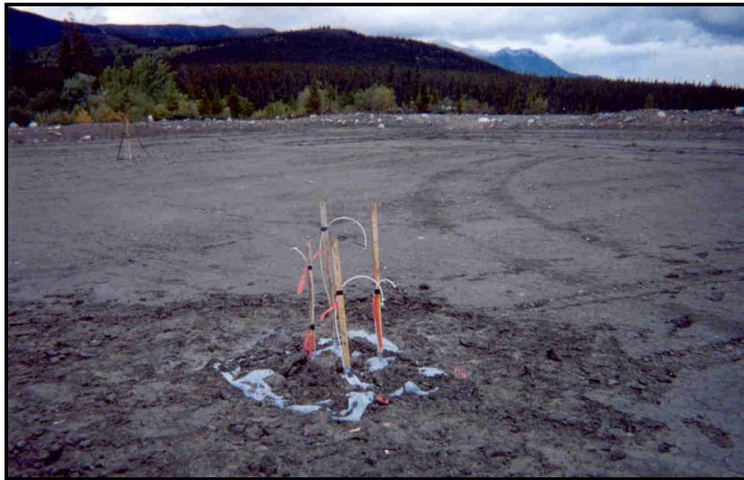
Photograph 1: View of the completed soil gas vapour probe SGP1. (September 2000)
