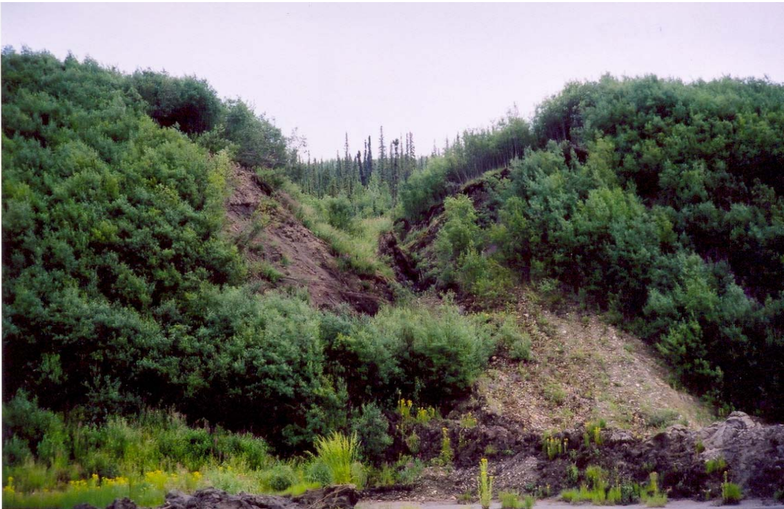
View of the slope failure from Gold Run Road. Note the gravel plug. July 14, 2003.
