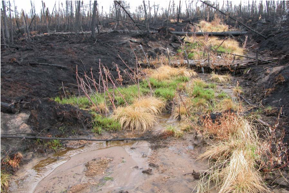
PLATE #19: Looking up to gully break #10 from intact gully break #11 (not in picture) Break # 10 is effectively holding back sediment terrace. Live staking of willows appear scorched but not dead. Most grasses are viable.
