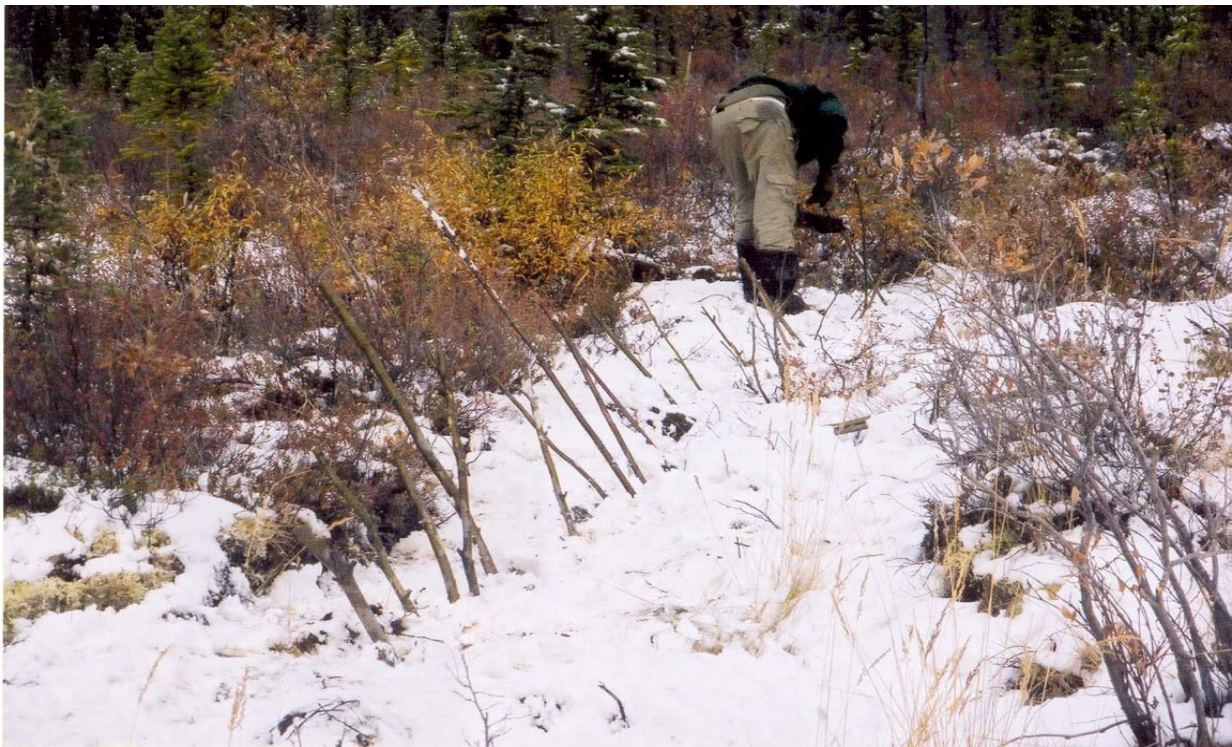
PLATE #8: Live staking up slope of "Y" pole drain, September 24, 2003.
