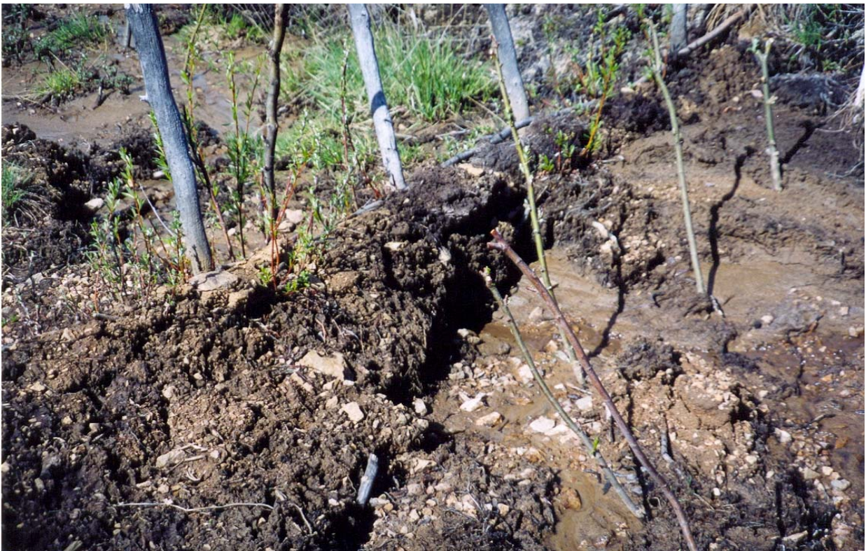
PLATE #14: Gully break #6 prior to upgrades, May 27, 2004.
