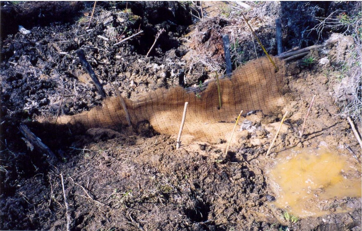
PLATE #12: Gully break #3 after placement of geotextile, May 27, 2004.
