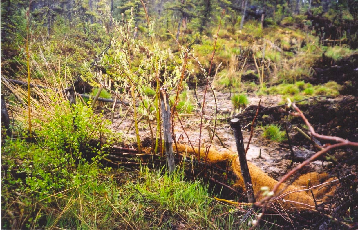
PLATE #13: Repaired gully break #8. Note spring shoots of willow growing from wattle fence.
