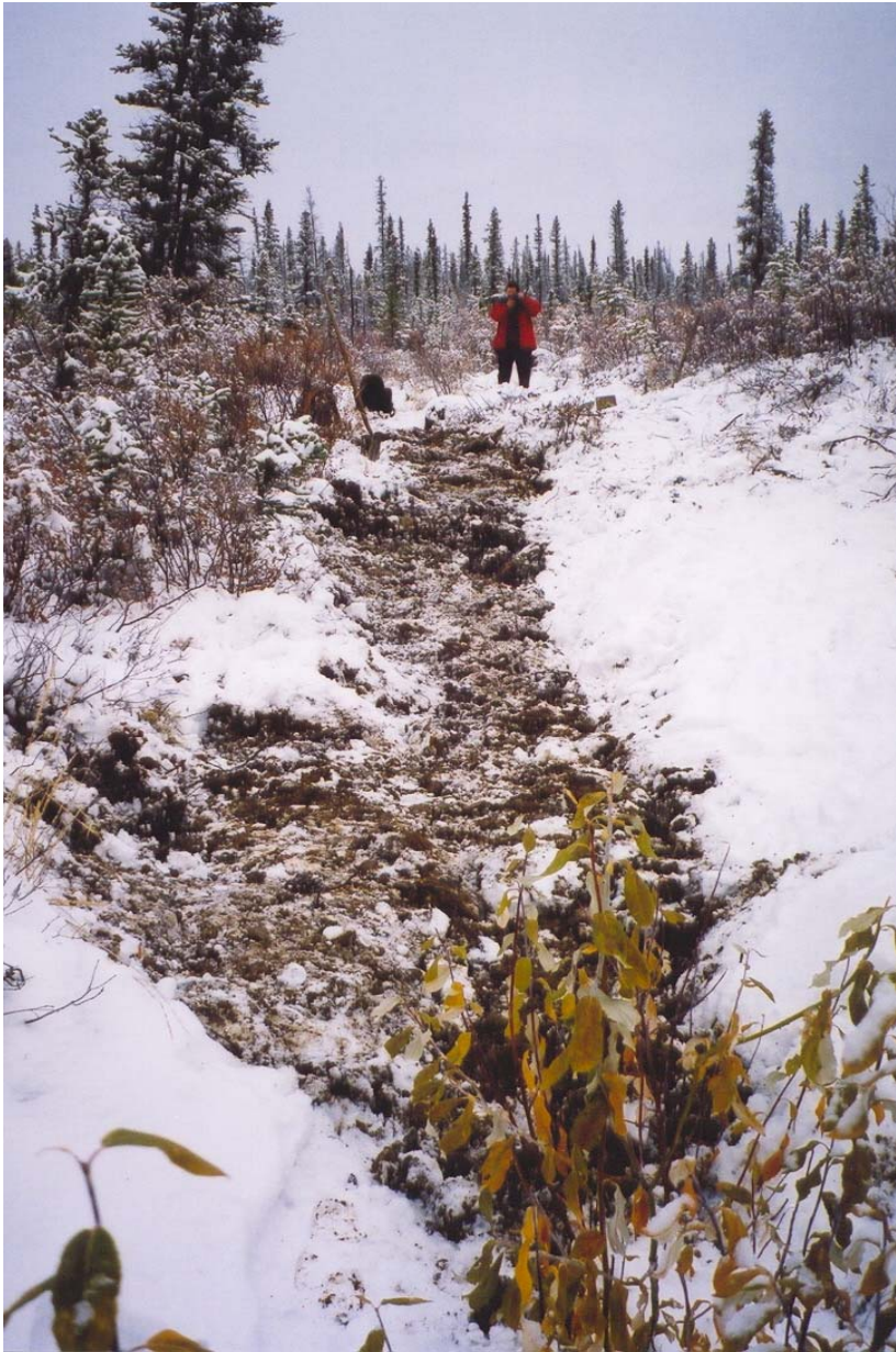
PLATE #6: Backfilling pole drain with frozen material.
