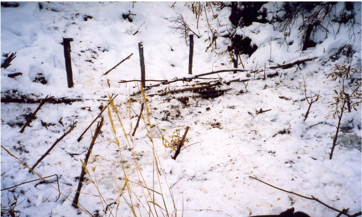
PLATE # 2: First gully break prior to upgrades. September 24, 2004.
