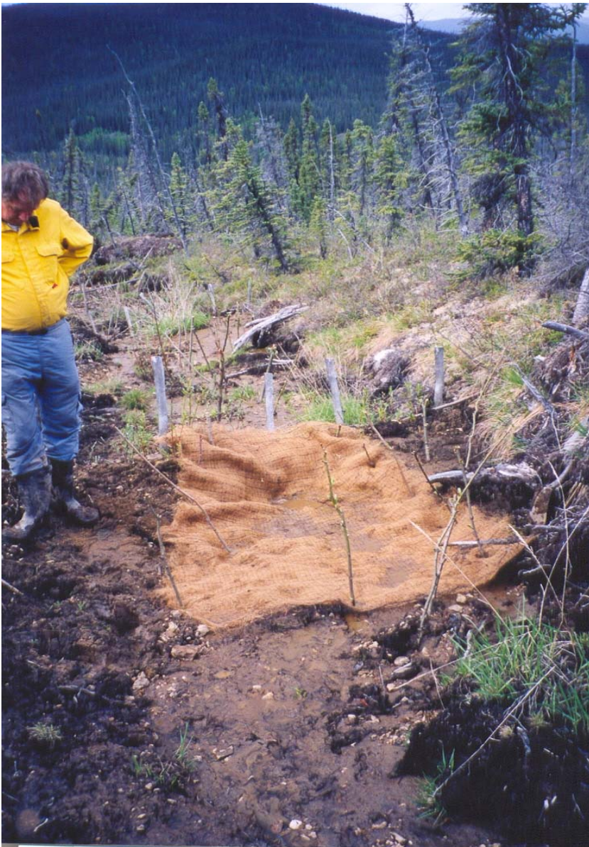
PLATE #15: Gully break #6 after upgrades. May 27/04.
