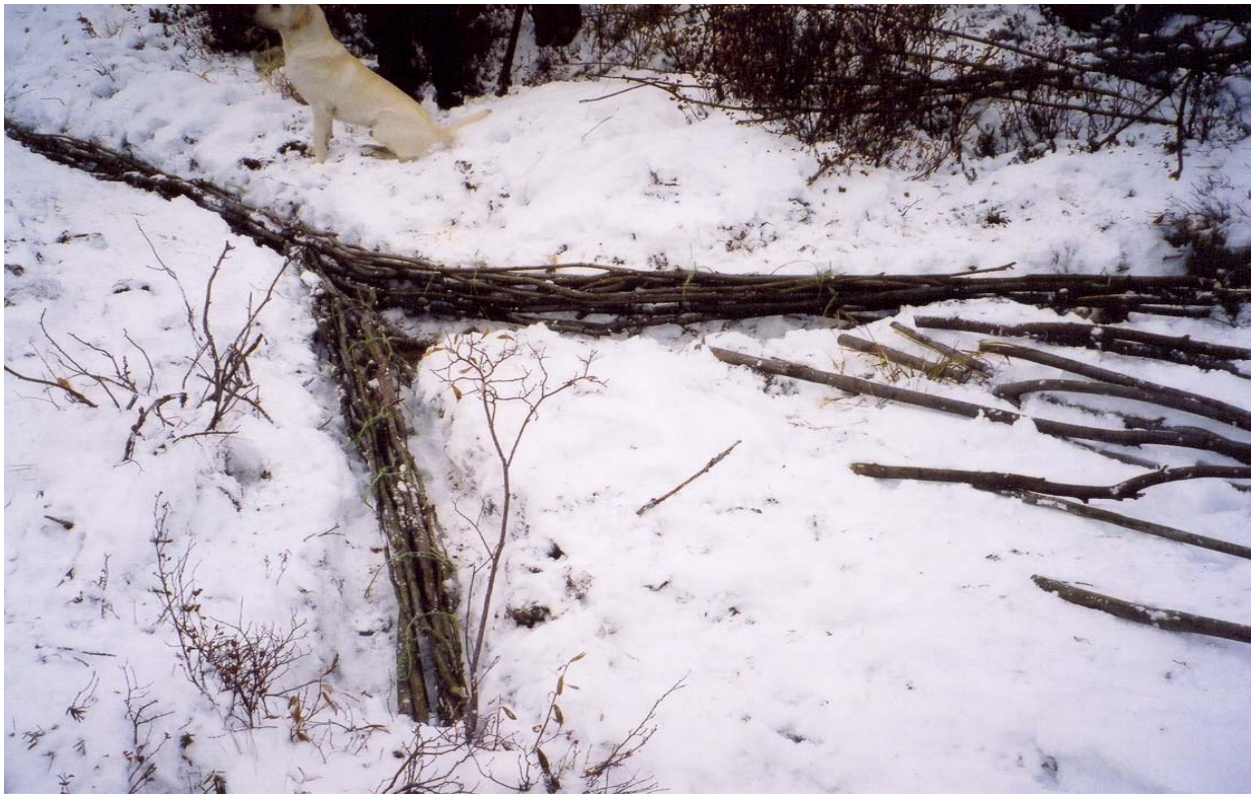
PLATE #7: "Y" pole drain at top of new pole drain, September 24, 2003.
