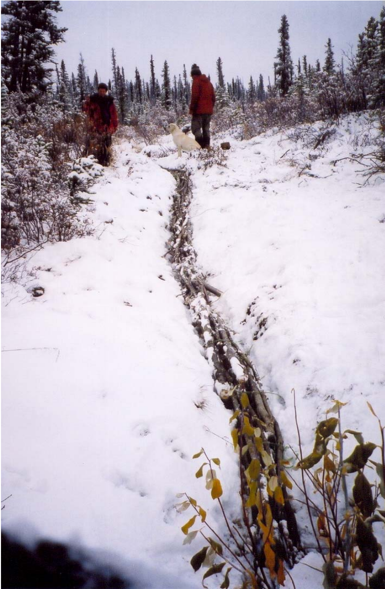
PLATE #5: Installing new pole drain into frozen trench.
