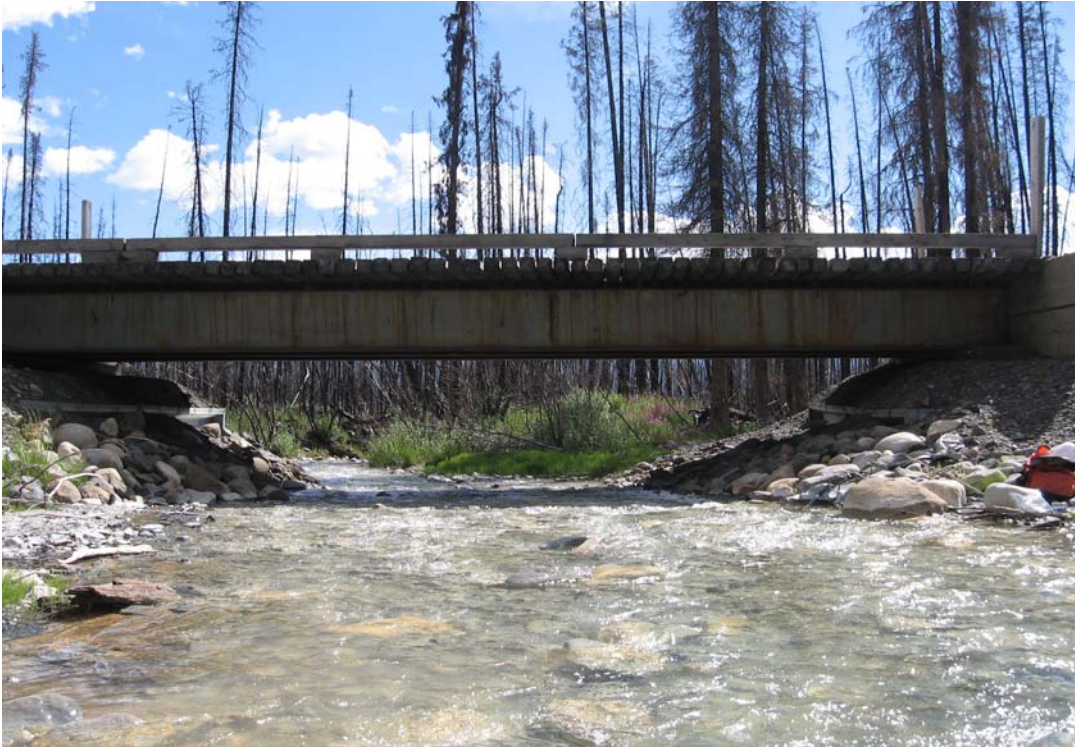
Water quality and flow measurement site M18, looking downstream on a Dewhurst Creek.
