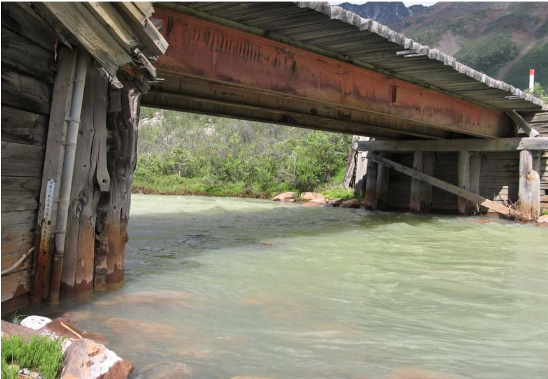
Water quality and flow measurement site M15, looking upstream on the South MacMillan River.
