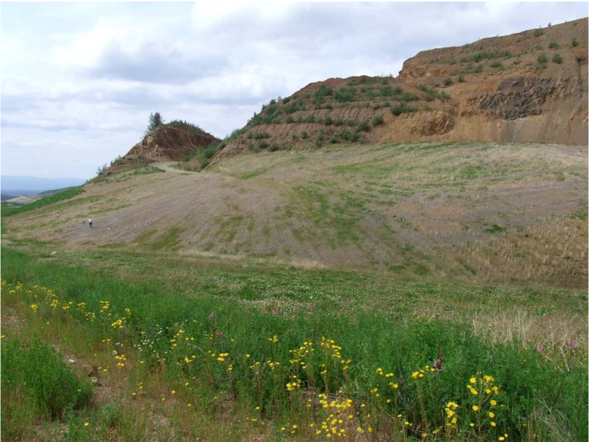
Photo #9: The Kokanee Inpit backfill area with the Haul Road in the foreground.
