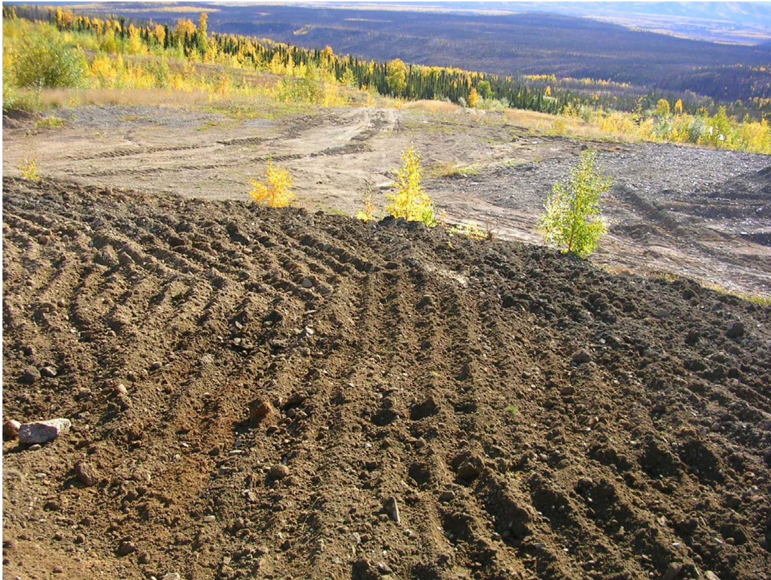
Final reclamation of water treatment pond
