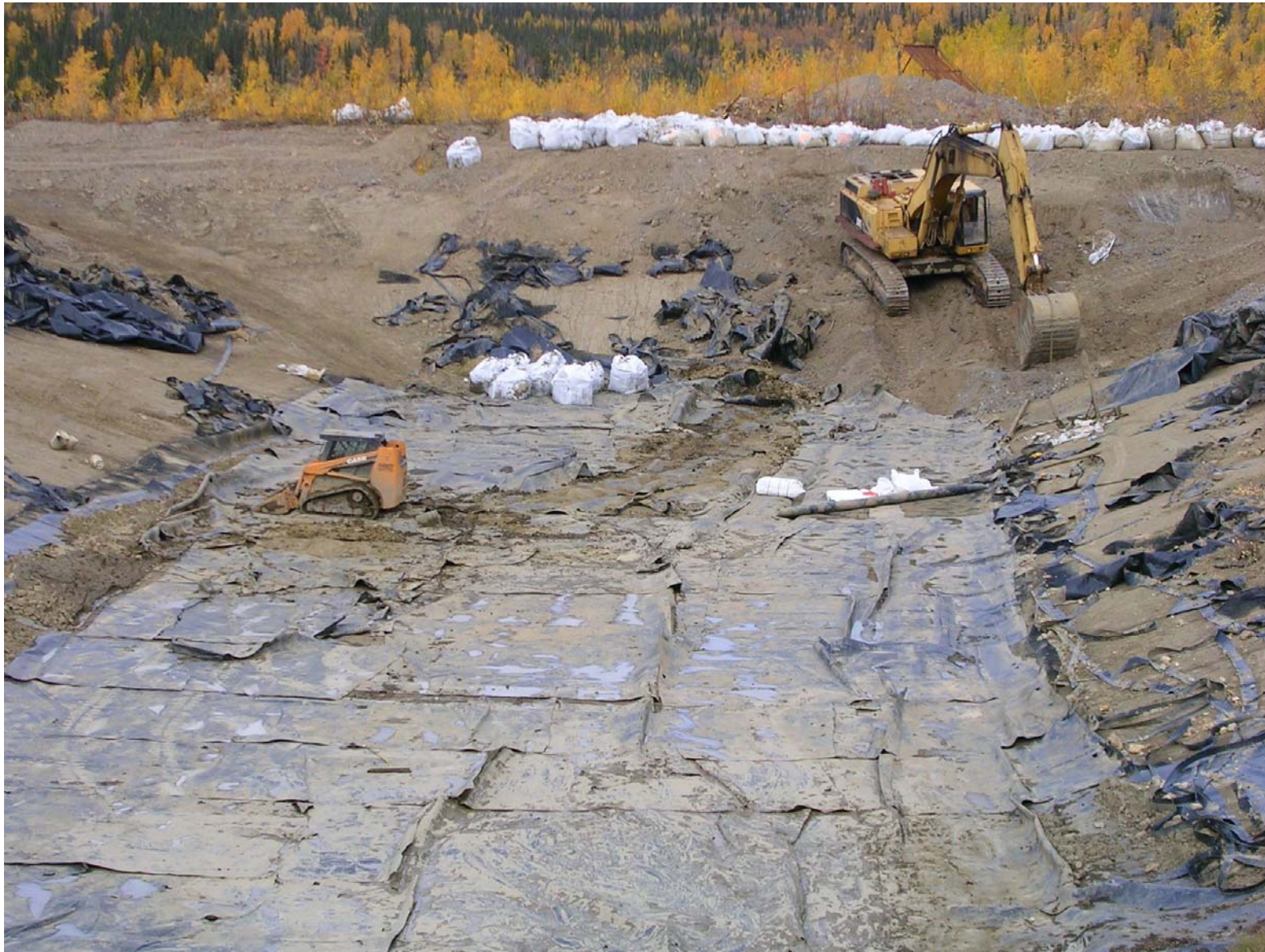
Removal of sludge and liner from preg pond
