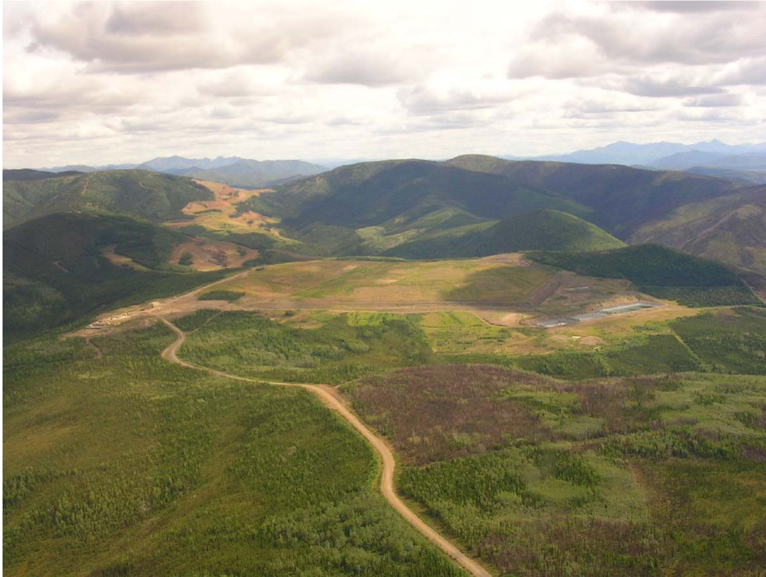
Looking east from the above the access road over the heap leach towards the open pits (2006)
