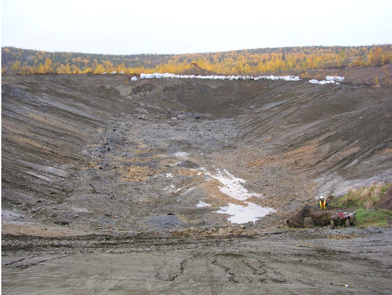
All sludge and liner removed from the preg pond
