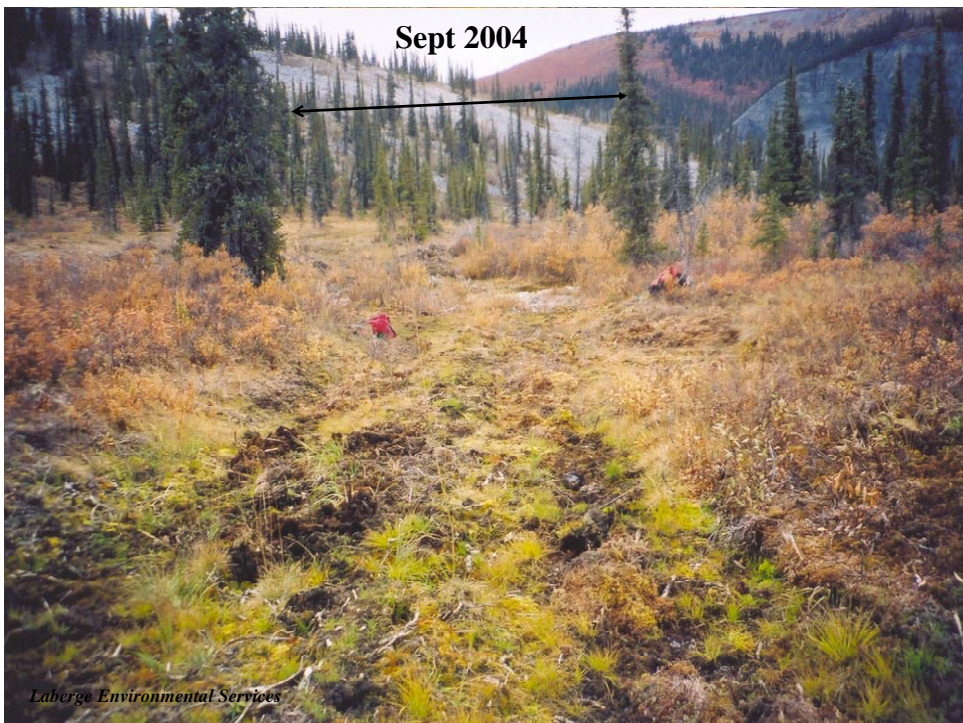
Photo #16: Completion of backfilling the problem areas, September 13 th , 2004.
