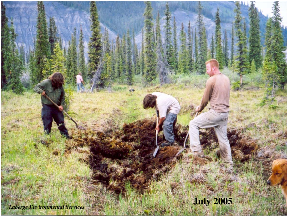
Photo # 27: Leveling and backfilling Site 7, July 13, 2005.
