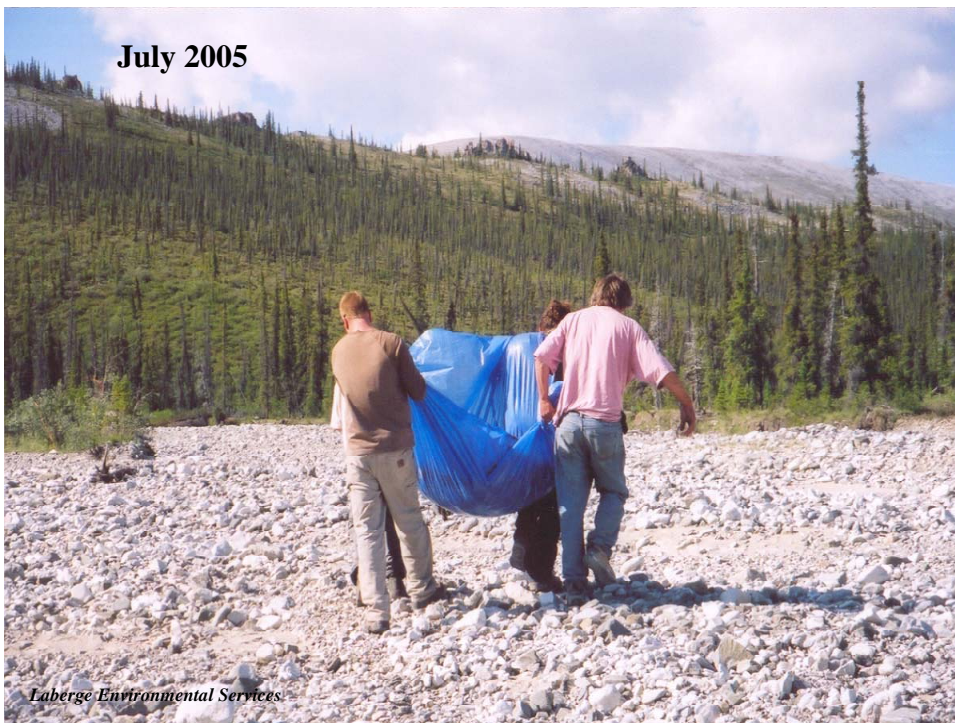
Photo # 44: Tarp loads of peat are hauled across the dry river bed to the trail head to be deposited into the ruts at Site 16.
