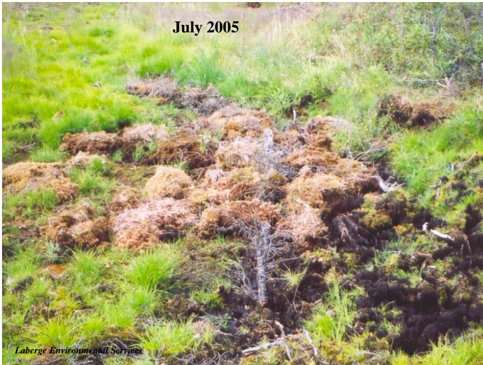
Photo # 12: Site #5; following backfilling with local material, July 2005.
