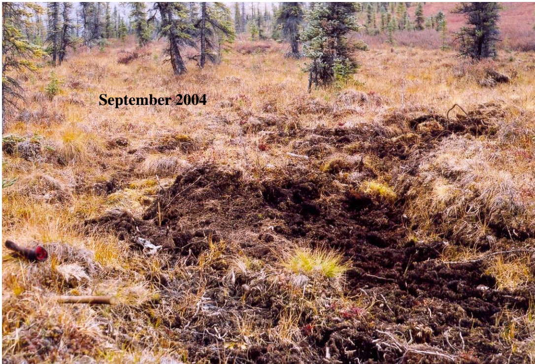
Photo #7: Site #2; the eroded and rutted corner has been backfilled with local material, Sept 13, 2004.
