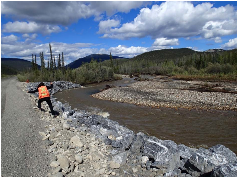
KM 172.9 (Photo 1). Looking downstream at recently placed riprap
