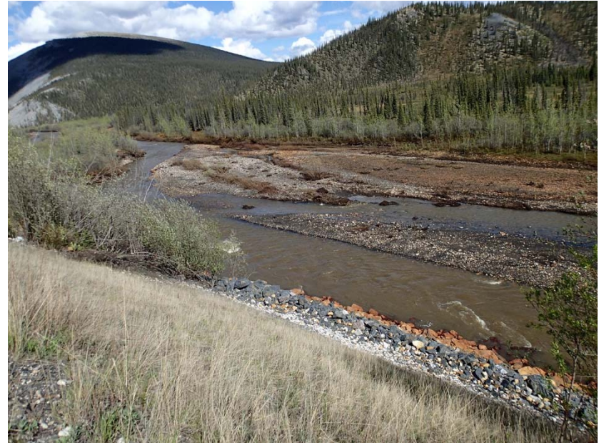
KM 175.2 (Photo 2). Looking downstream at recently placed riprap from atop the scarp
