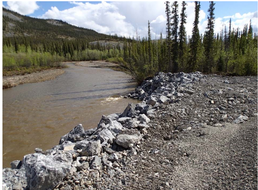
KM 172.9 (Photo 2). Looking upstream at recently placed riprap
