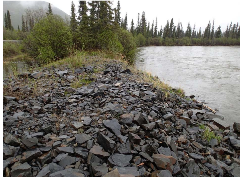
KM 131.4 (Photo 2). Looking downstream from riprap spur
