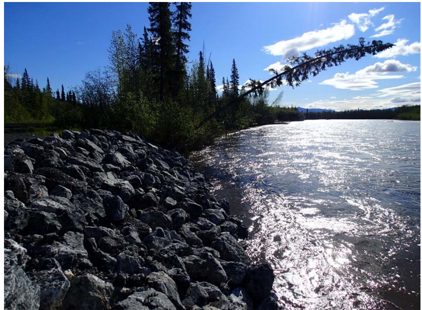
KM 243.8 (Photo 2). Leaning trees downstream of recently placed riprap
