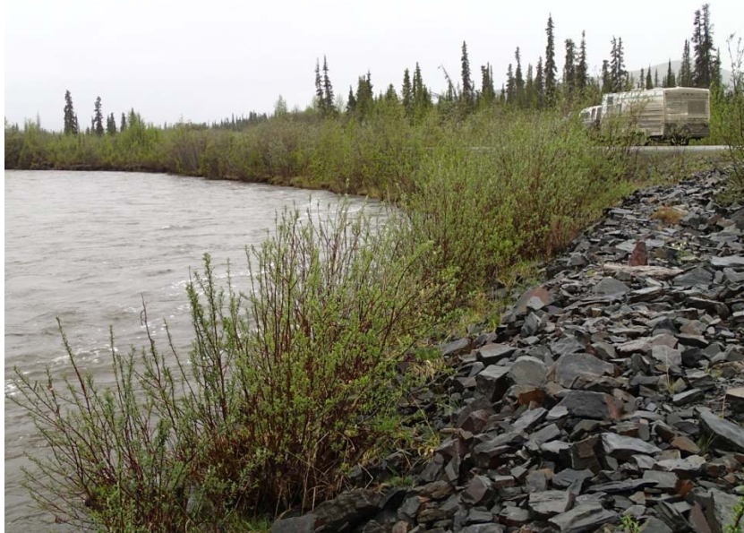
KM 131.4 (Photo 1). Looking upstream from riprap spur
