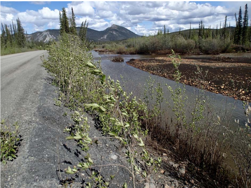
KM 180.7 (Photo 1). Looking downstream from highway embankment
