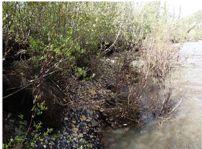
KM 185.8 (Photo 2). Slumping/exposed banks
