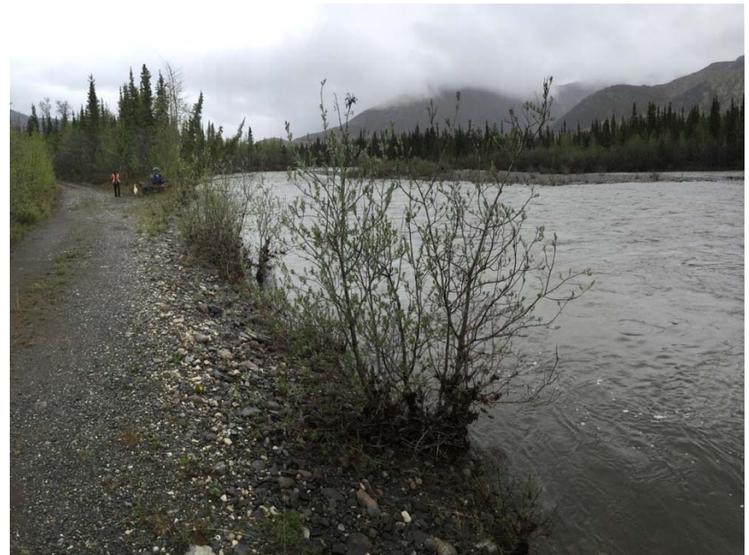
KM 136.1 (Photo 2). Looking downstream from previously placed riprap
