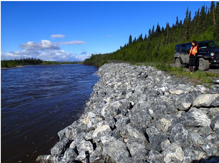
KM 243.8 (Photo 1). Looking upstream from recently placed riprap
