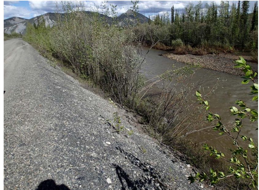
KM 181.5 (Photo 2). Looking downstream from highway embankment
