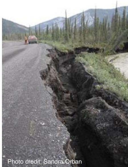
Figure 2-5. Meander-induced Mass Movement of Highway Embankment along Engineer Creek at km 182
