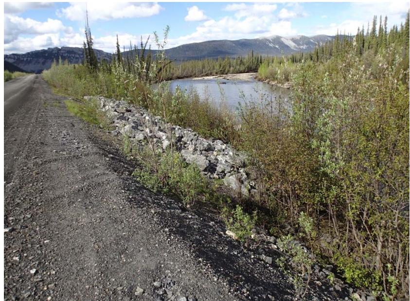
KM 189.4 (Photo 2). Looking downstream from highway embankment
