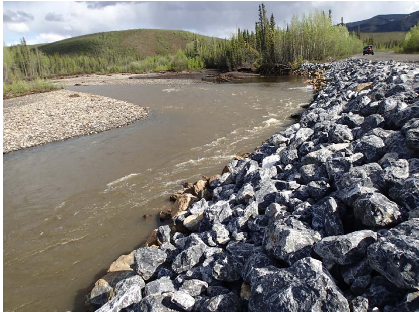
KM 188.6 (Photo 1). Looking upstream at channel approach from recently placed riprap
