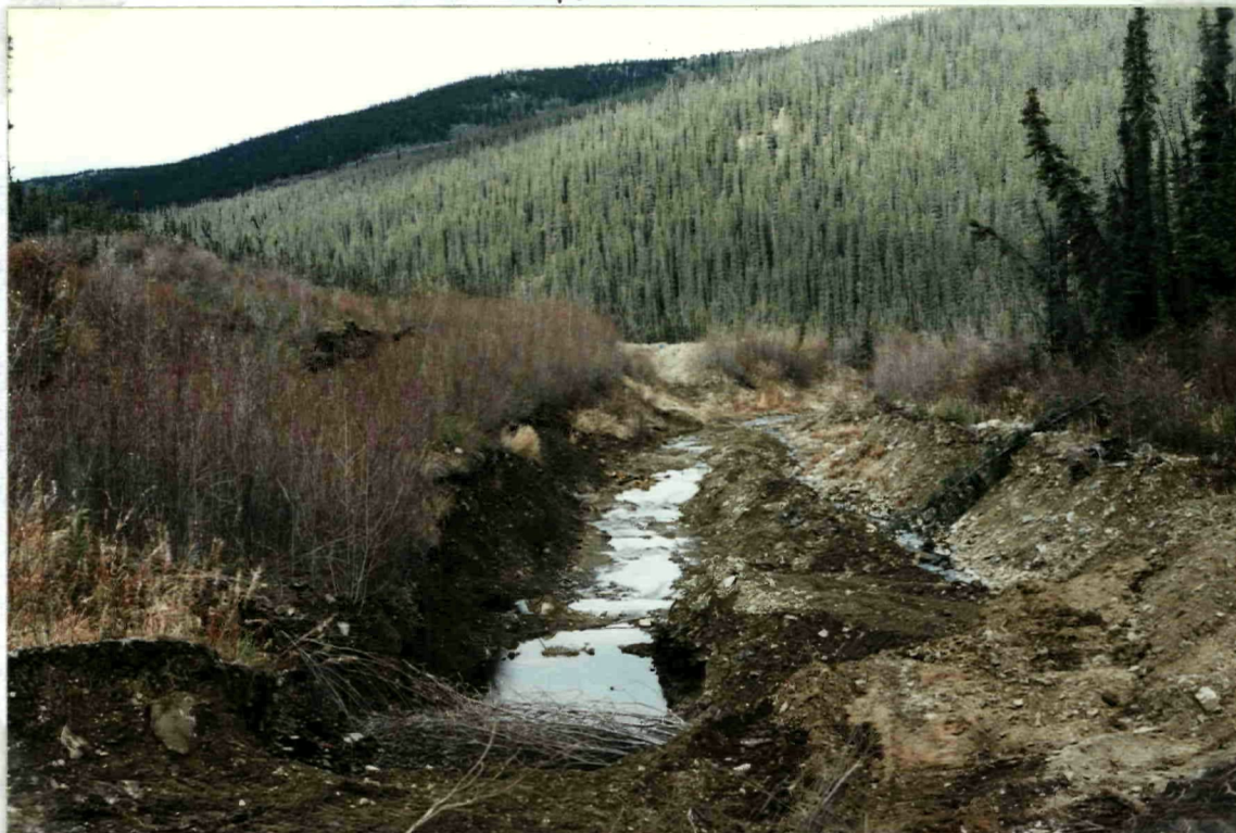
TRENCH SITE #1 SAMPLE SITE #1, #2, #3 LOOKING DOWNSTREAM TO STODDART CR.
